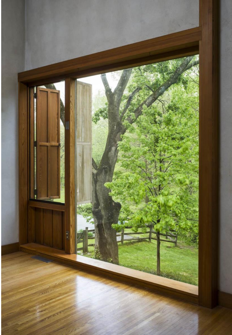
Photo 15 – The dining area features an eight-by-ten foot window that looks out onto the sloping yard and the creek beyond. To the west of this window is a large, shuttered window opening, containing no glass, which opens inside of the house to the outside. (National Trust/Tom Crane, Photographer)
