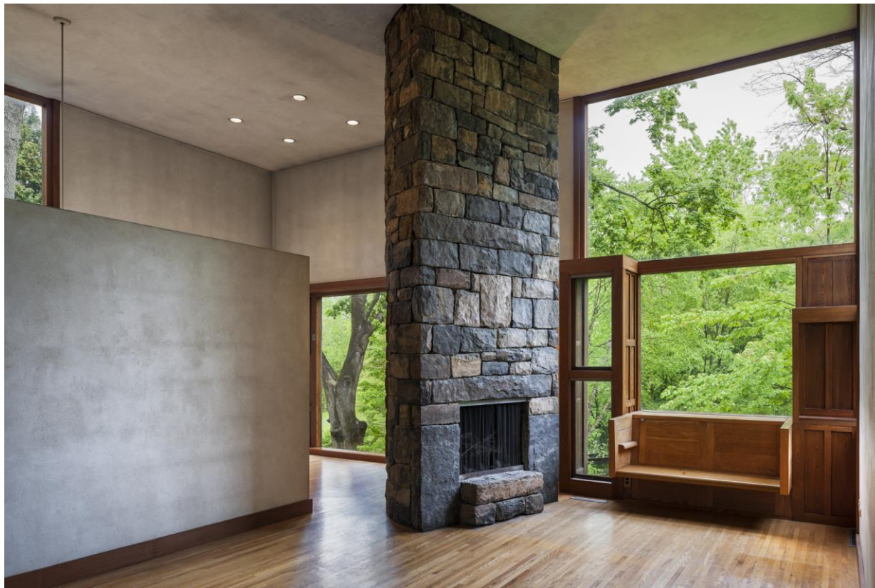
Photo 11 – The semi-cylindrical chimney made of random rubble “Montgomeryville” limestone serves as the centerpiece of the living cube. The built-in window seat complements the hearth and creates a space where people can gather in the natural light from the surrounding windows. (National Trust/Tom Crane, Photographer)
