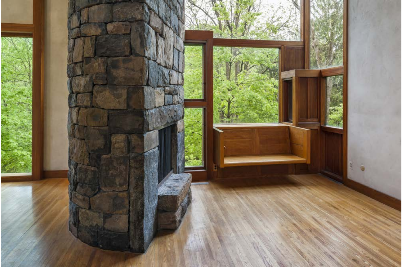
Photo 12 – Detail of the semi-cylindrical hearth and window seat in the living cube. (National Trust/Tom Crane, Photographer)
