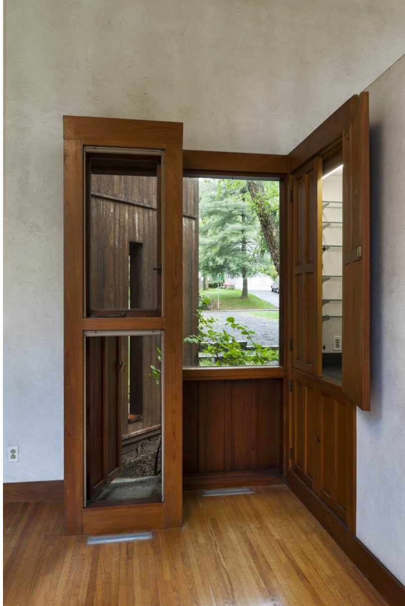
Photo 13 – A window unit located on the southwest wall of the living cube. At the west end of the partition wall is a wet bar with a sink and shelving hidden behind mill-worked doors. (National Trust/Tom Crane, Photographer)
