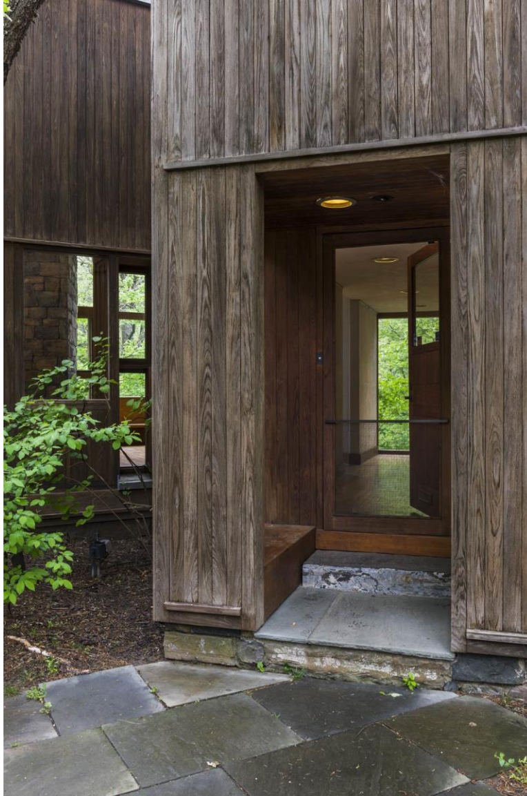
Photo 7 – The main entrance is inset into the west elevation of the sleeping cube and features a small, elevated porch with a slate floor and a low built-in bench. (National Trust/Tom Crane, Photographer)
