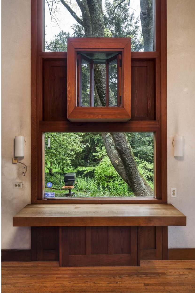
Photo 17 – Opposite the kitchen, on the northwest wall of the living cube is a rectilinear “breakfast table” with pullout drawers and a distinctive deeply-inset window above. (National Trust/Tom Crane, Photographer)
