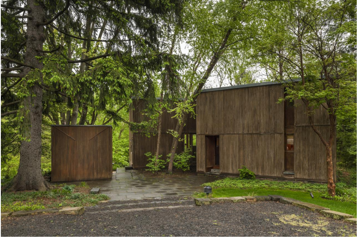
Photo 6 – The west elevation of the sleeping cube is in the foreground and the north elevation of the living cube is in the background. The flagstone walkway is original. The stone edging around the northern edge of the driveway was added by Rodney Robinson in 1983. The utility shed is to the northwest of the house.
