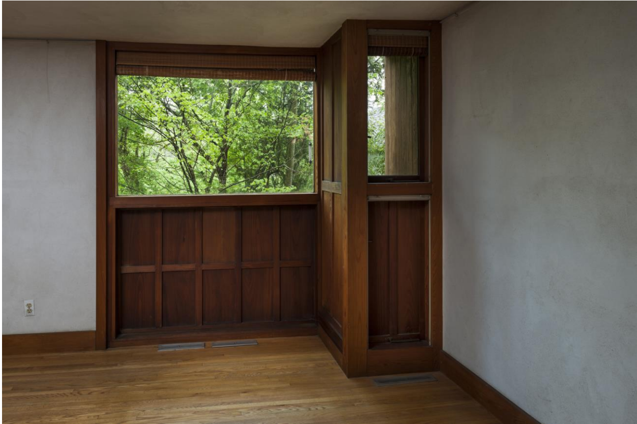
Photo 10 – A deeply-inset window unit on the southeast corner of the master bedroom. There are three of these window units in the master bedroom. (National Trust/Tom Crane, Photographer)
