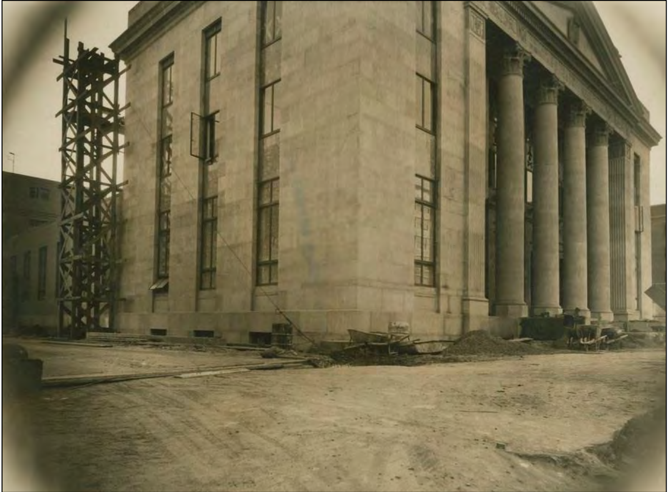
Figure 3. A construction progress photograph from November 1, 1933 shows the building's original casement windows.
