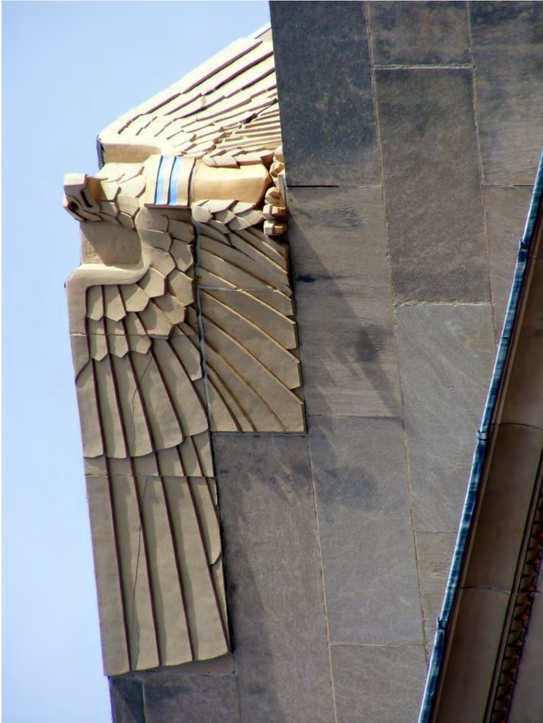
KS_Shawnee County_United States Post Office and Court House_0003
