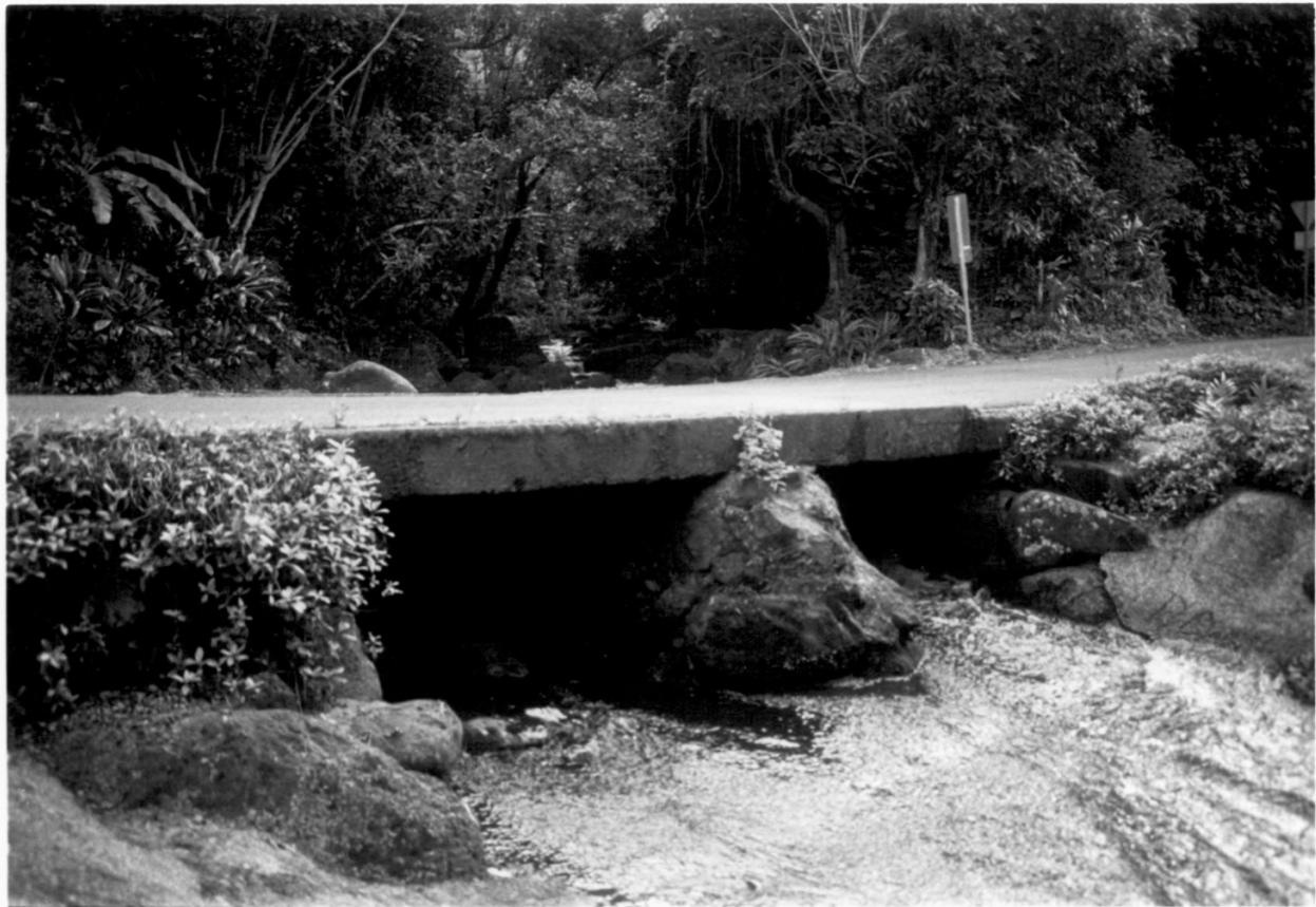
Kaua'i Belt Road, Kaua'i County, HI # 13
