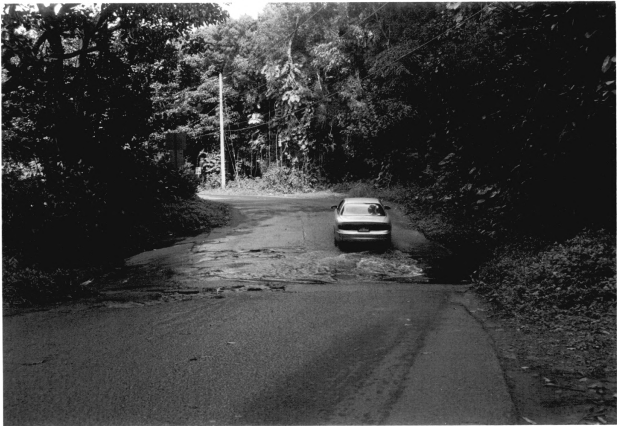
Kaua'i Belt Road, Kaua'i County, HI # 12
