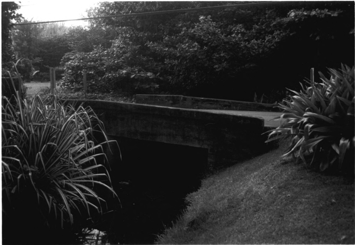
Kaua'i Belt Road, Kaua'i County, HI # 11
