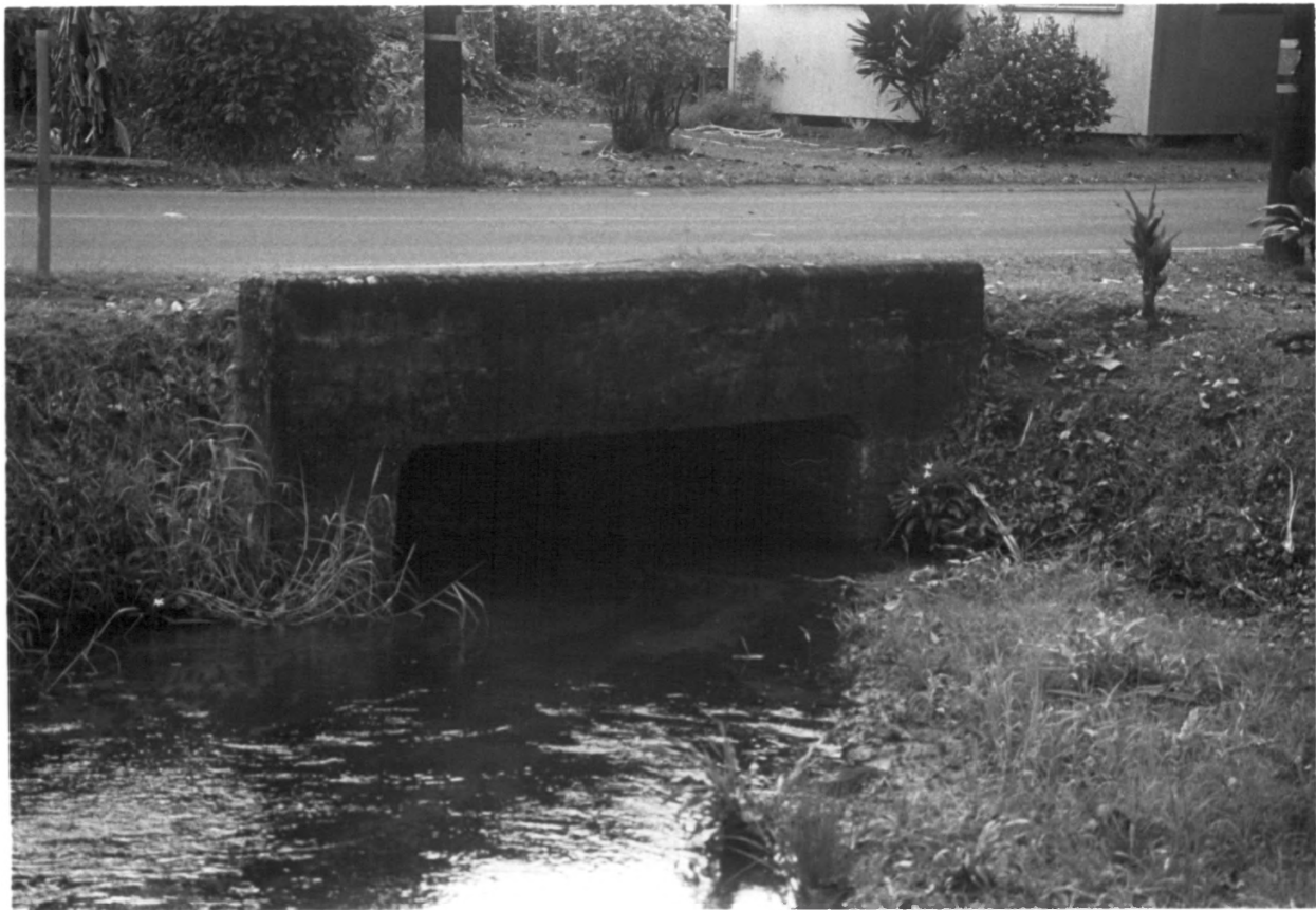
Kaua'i Belt Road, Kaua'i County, HI #4
