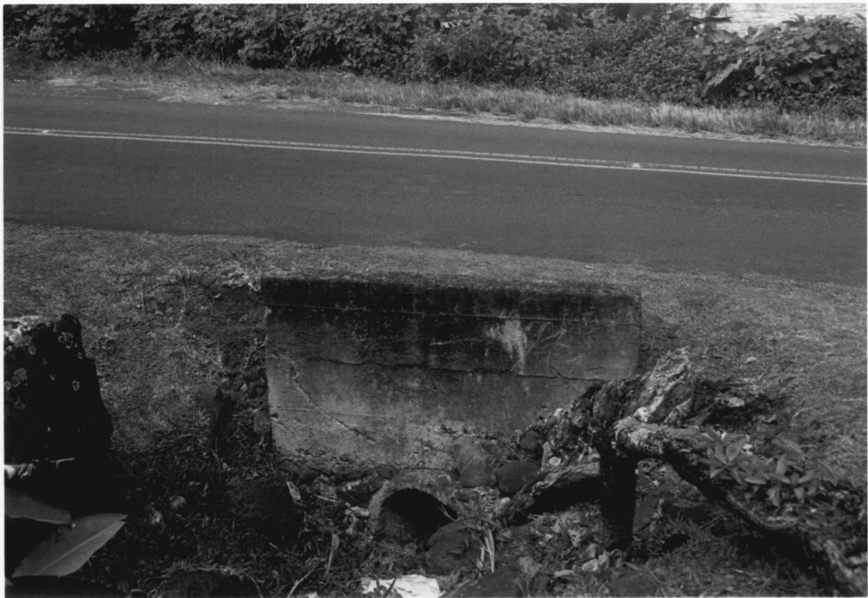
Kaua'i Belt Road, Kaua'i County, HI #20
