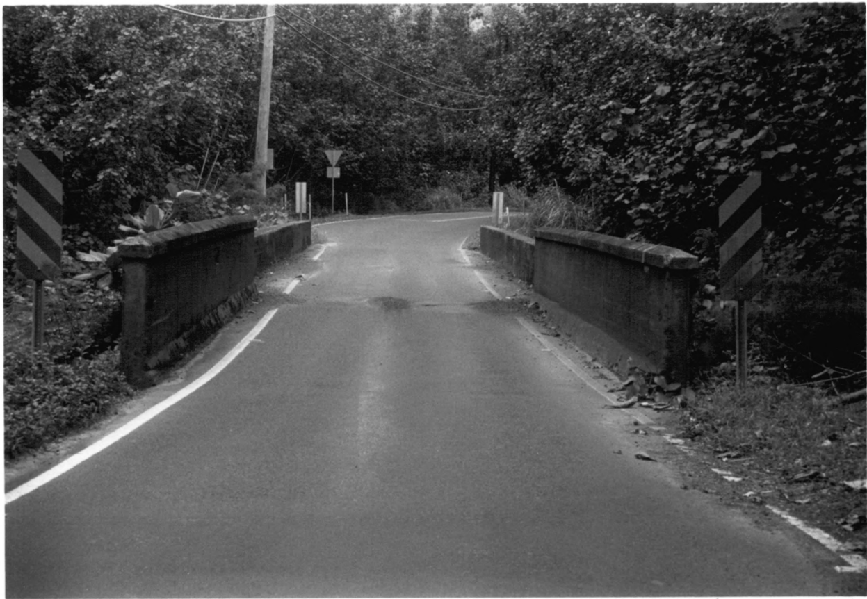
Kaua'i Belt Road, Kaua'i County, HI #6
