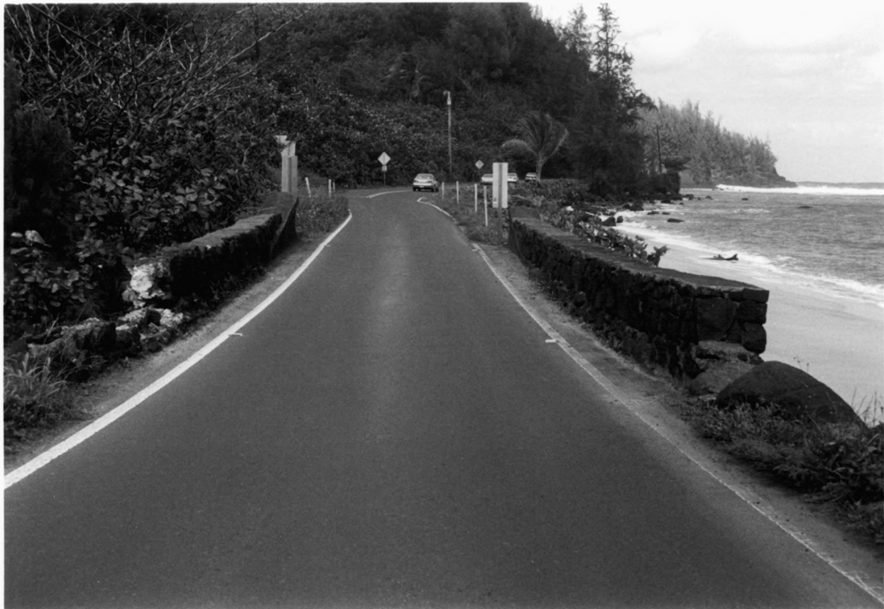
Kaua'i Belt Road, Kaua'i County, HI #14
