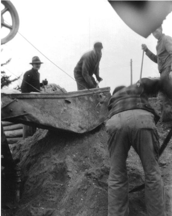
a. Hand excavating the basement and foundations
