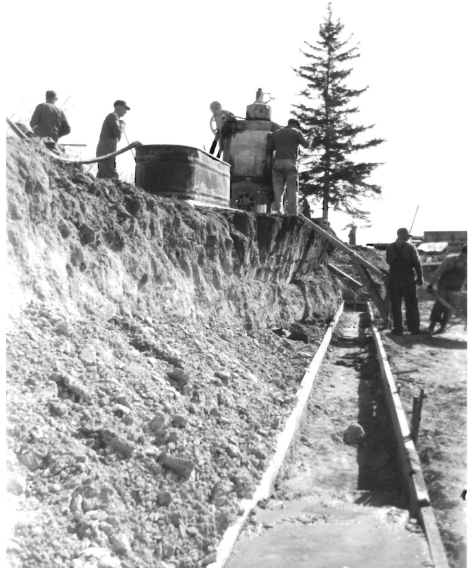
b. Forming the new footings, with concrete mixer
