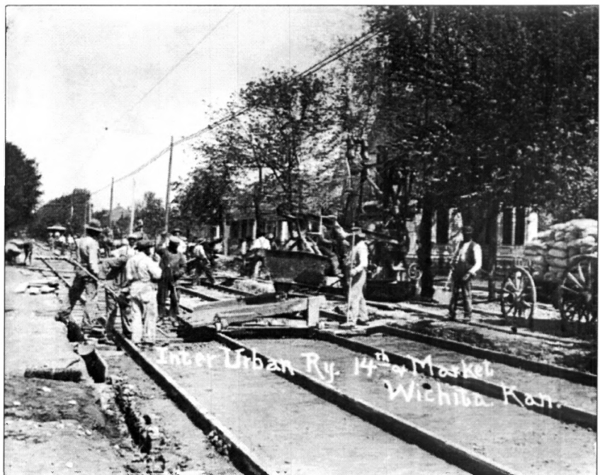
Track Laying for Arkansas Valley Interurban Railway at 14 th and Market, Wichita 1910
