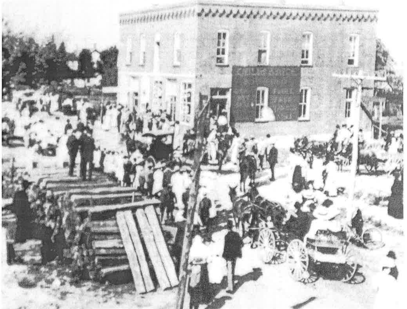
Fig. 2 This view along West Main Avenue looks across South Smith Street and show the c. 1885 Kinder Building on the corner but not the 1897 Hotel Grand which was eventually built beside it to the west. The railroad ties indicate that some manner of rail construction project was on-going at the time. [Crawford County Historical Society]
