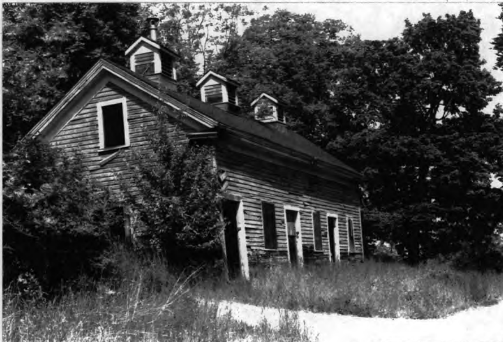
Outbuilding (Hen house?)
