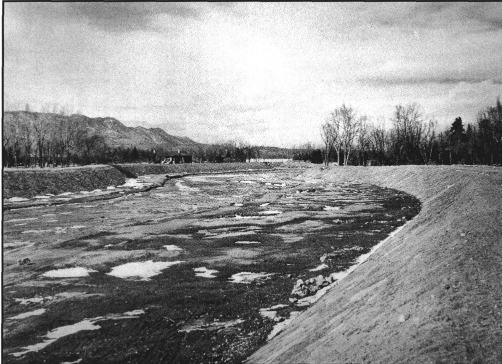
Figure 8. The WPA widened the channel of Monument Creek and created slanting walls riprapped with sandstone as a flood control measure following the deluge of Memorial Day 1935. The effort spanned five years and cost at least $1.2 million. SOURCE: City of Colorado Springs, Annual Report, Fiscal Year Ending December 31, 1936 (Colorado Springs: City of Colorado Springs, 1936).
