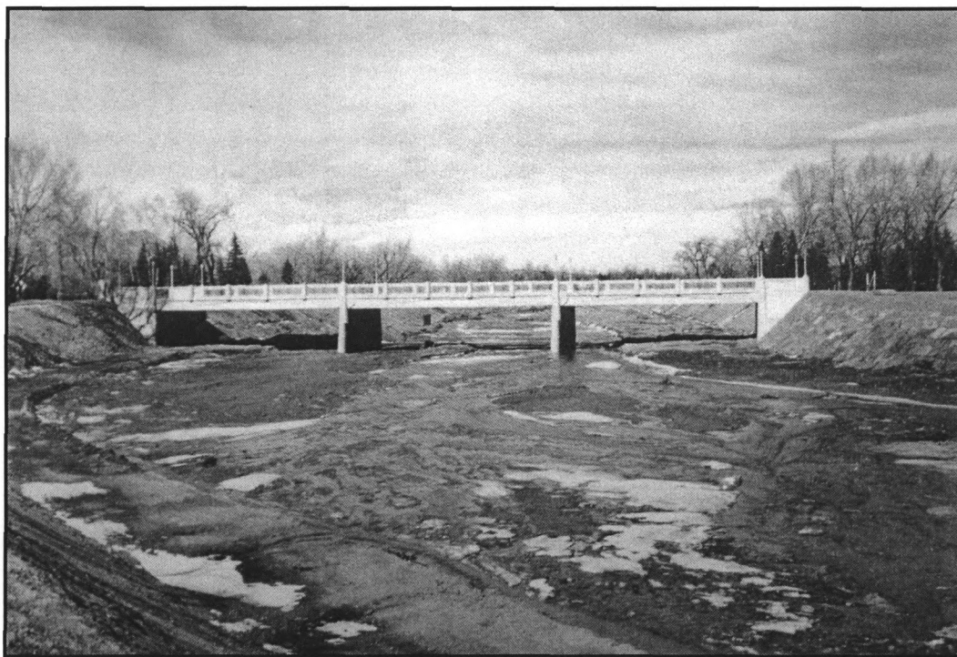
Figure 9. The replacement of the Mesa Road (above) and Uintah Street bridges in the park were achieved through Public Works Administration funding. Due to the widening of the streambed the new bridges were considerably longer than the ones they replaced. SOURCE: City of Colorado Springs, Annual Report, Fiscal Year Ending December 31, 1936 (Colorado Springs: City of Colorado Springs, 1936).
