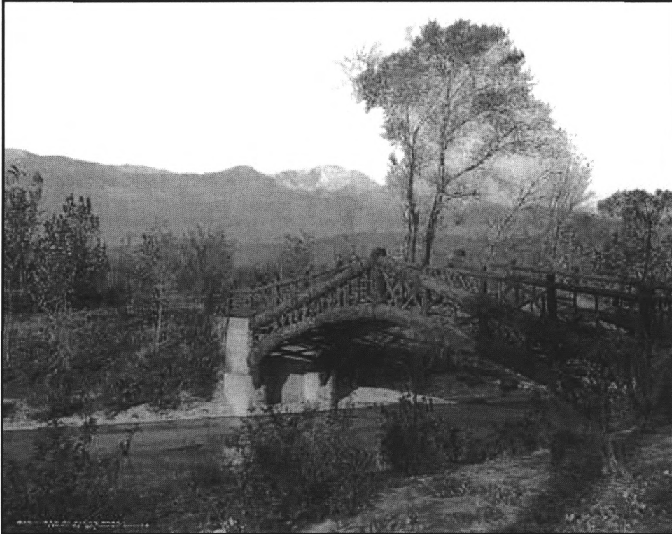
Figure 2. The original construction of the park ripped the banks of Monument Creek, but the channel was still sufficiently narrow to be spanned with this Rustic bridge of unpeeled logs. SOURCE: Denver Public Library, Western History and Genealogy Department, L.C. McClure image number MCC-809, Denver, Colorado.
