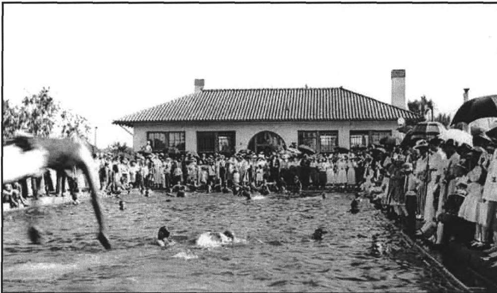
Figure 6. The Penrose Bathhouse and Swimming Pool is pictured here in 1916, the year it opened. It survived the 1935 flood and continues to be a popular attraction. SOURCE: Pikes Peak Regional Library District, Special Collections, E.L. Fowler image, call number 001-2252-di-72, Colorado Springs, Colorado.
