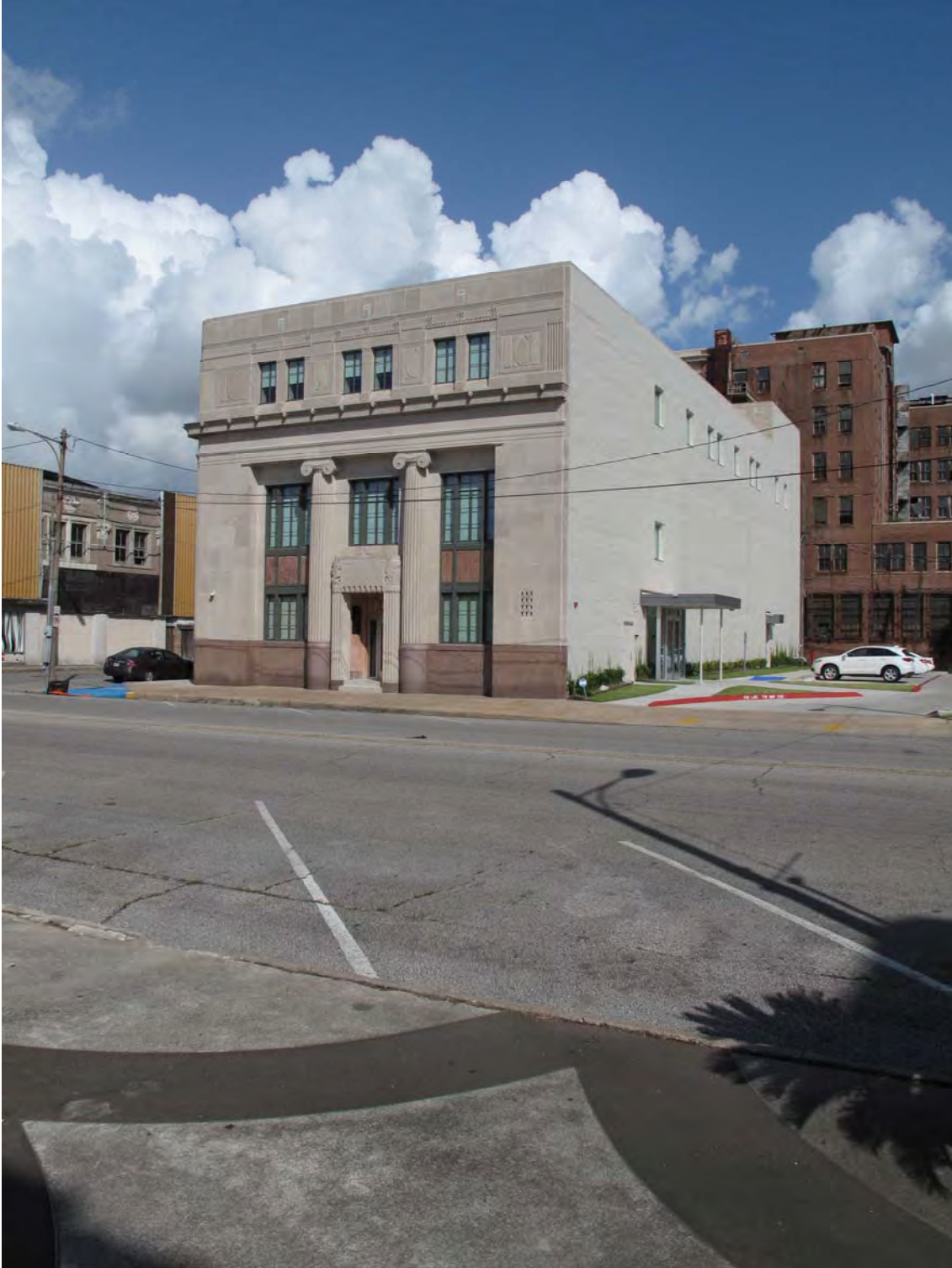
TX_Jefferson County_First National Bank of Port Arthur_0002 Procter Street elevation. Camera facing west.
