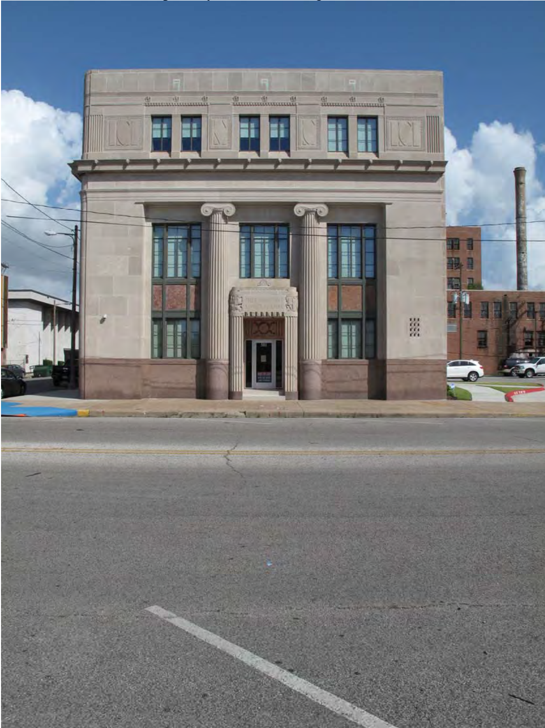
TX_Jefferson County_First National Bank of Port Arthur_0005 Procter Street elevation (primary). Camera facing northwest.
