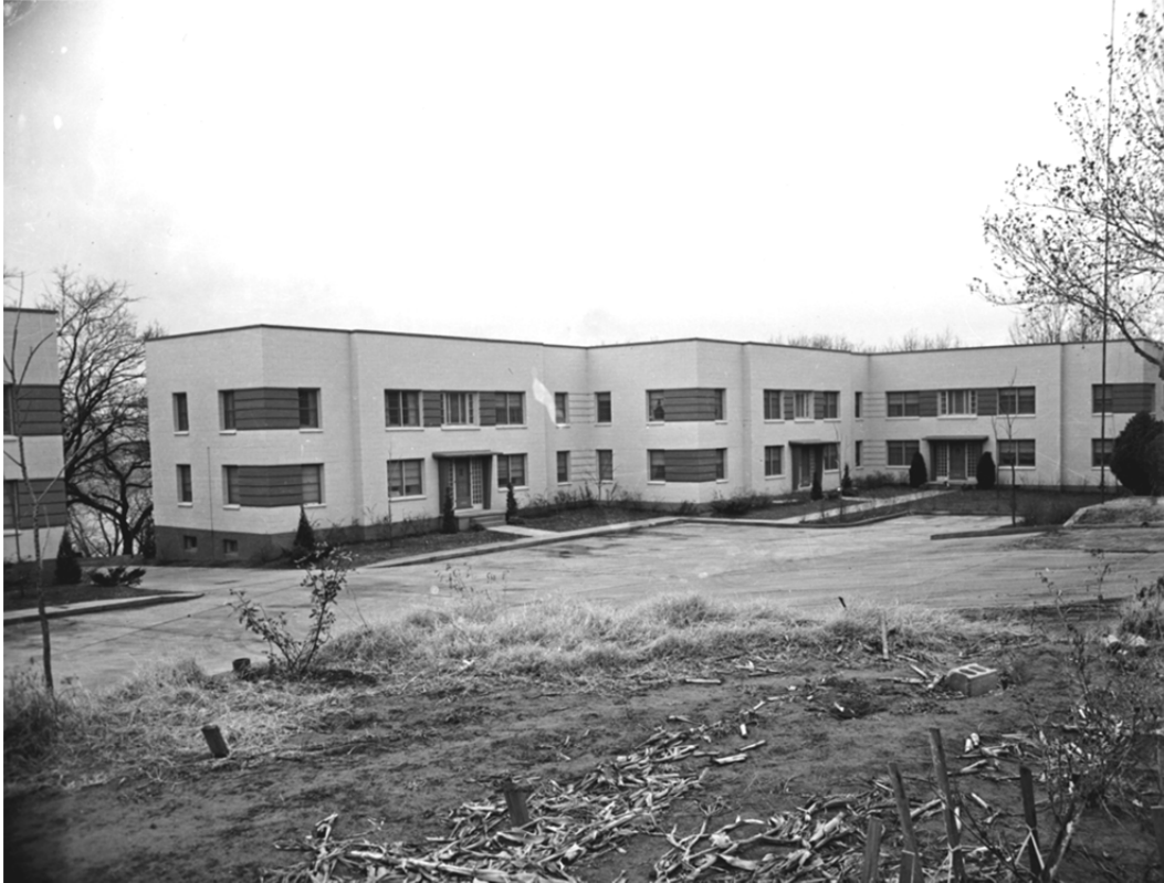
Looking SW at 1314 – 1312 & 1310 comprising west section of Sally Ann Apartments
