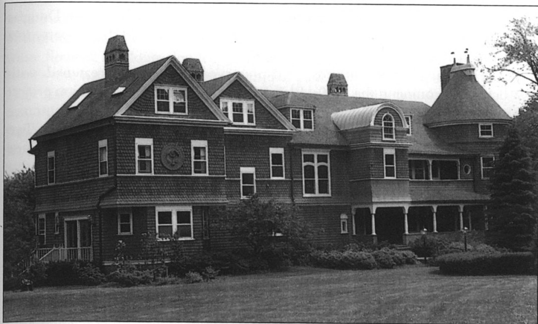
The McKim, Mead, and White-designed William A. Street house built in 1887 at 70
