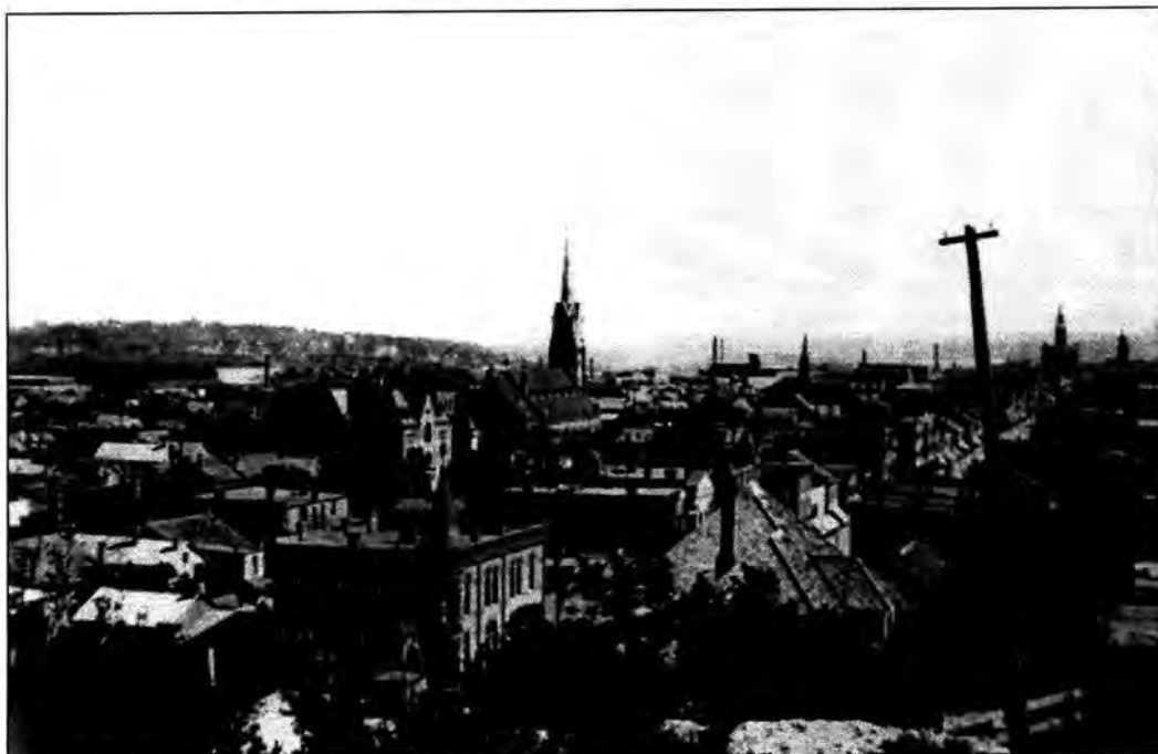
Figure 18: Overview from above the fire house (1805 Central Avenue), ca. 1915, view southeast (Center For Dubuque History, Hoffman Photo #1227)
