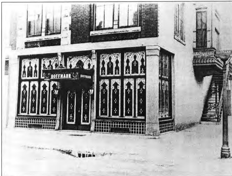
Figure 16: Remodeled façade and exterior, 1497 Central Avenue, ca. 1910 (Center For Dubuque History, Photographs, Hoffman, Photo #1056)
