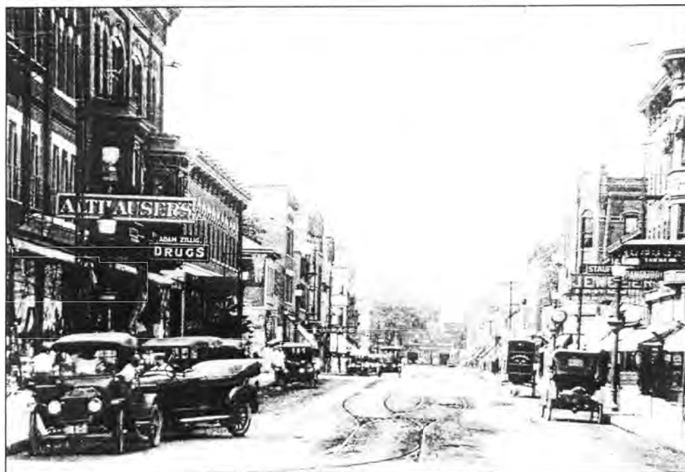
Figure 14: View north on Clay from 13 th Street, ca.1920, note single-story firehouse (Center for Dubuque History, Loras College, Photograph Hoffman #1054)
