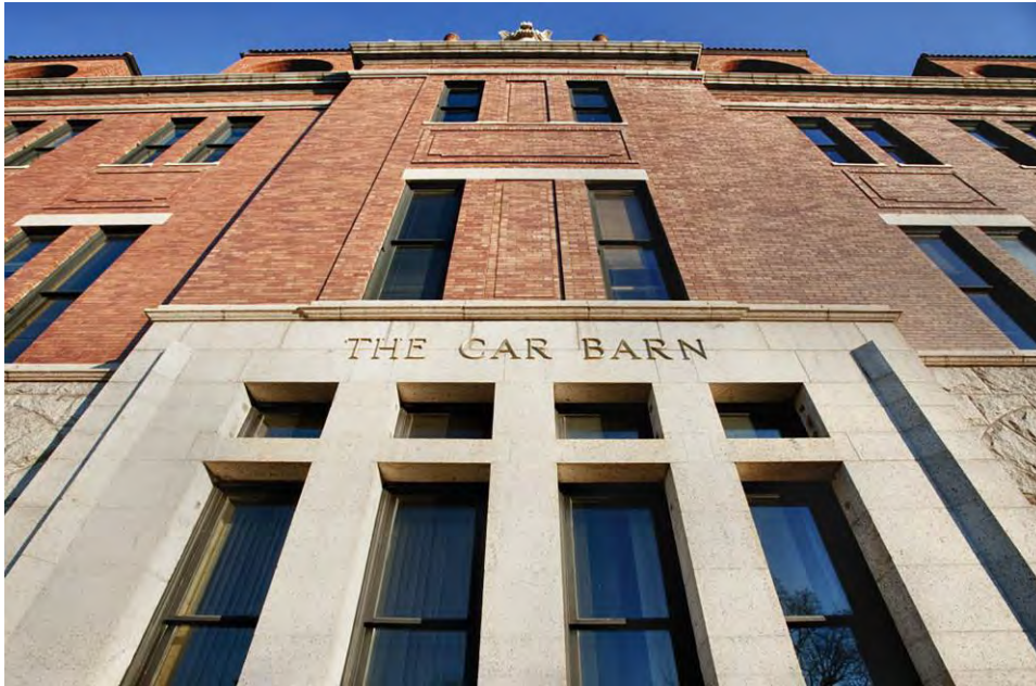
Image 14 of 19 View looking skyward at central block, south elevation
