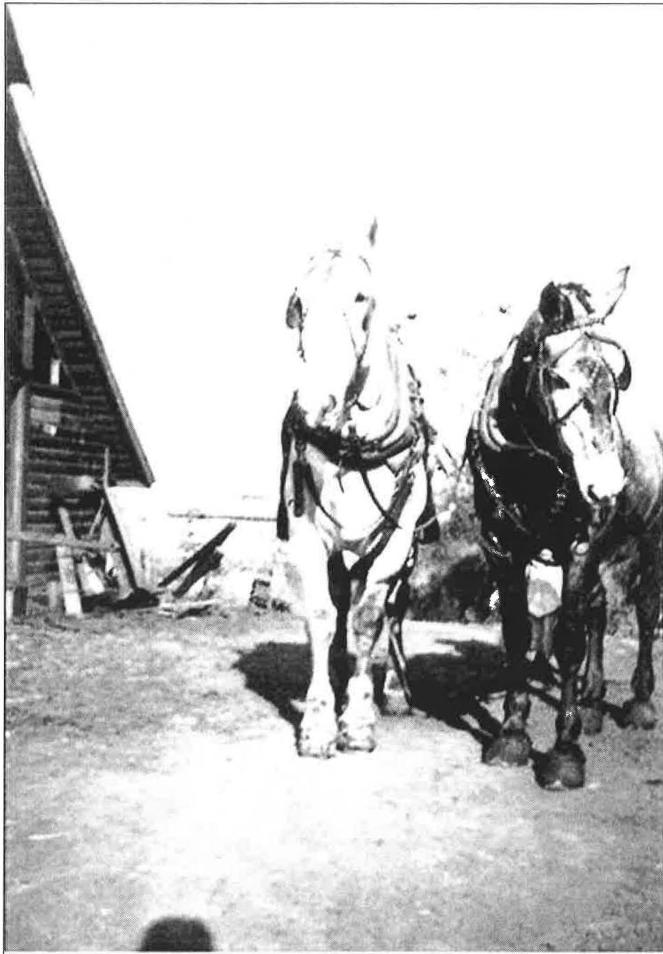
Figure 15: Horses in alley on northeast side of barn, unknown year; 1912 shed addition seen on left side of image. 50
