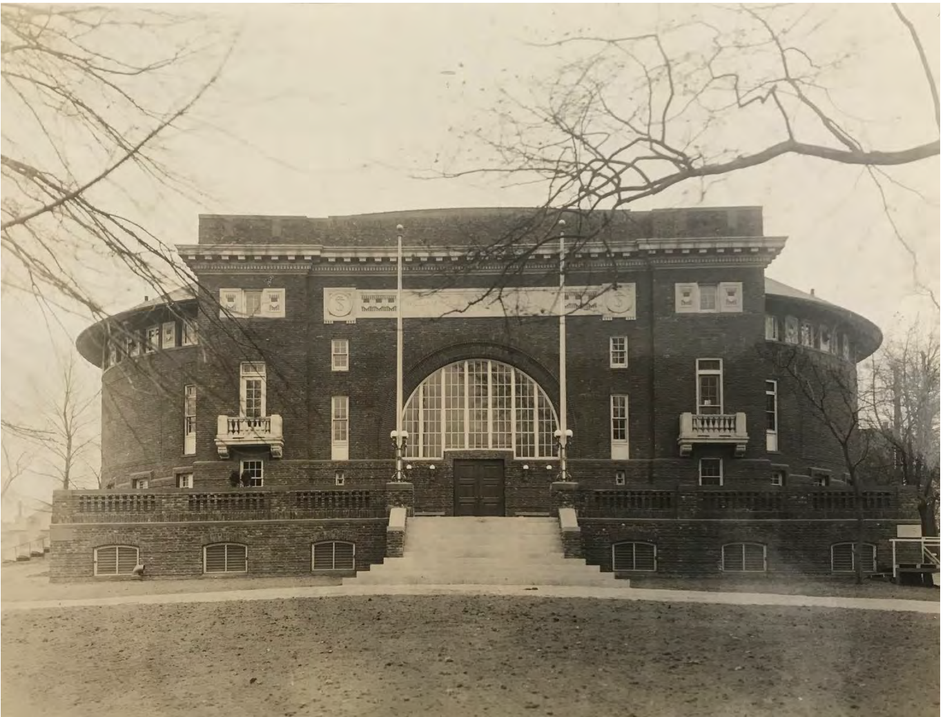
Figure 14. Walker Gymnasium, shortly after completion in 1916. (Archives and Special Collections, Stevens Institute of Technology)
