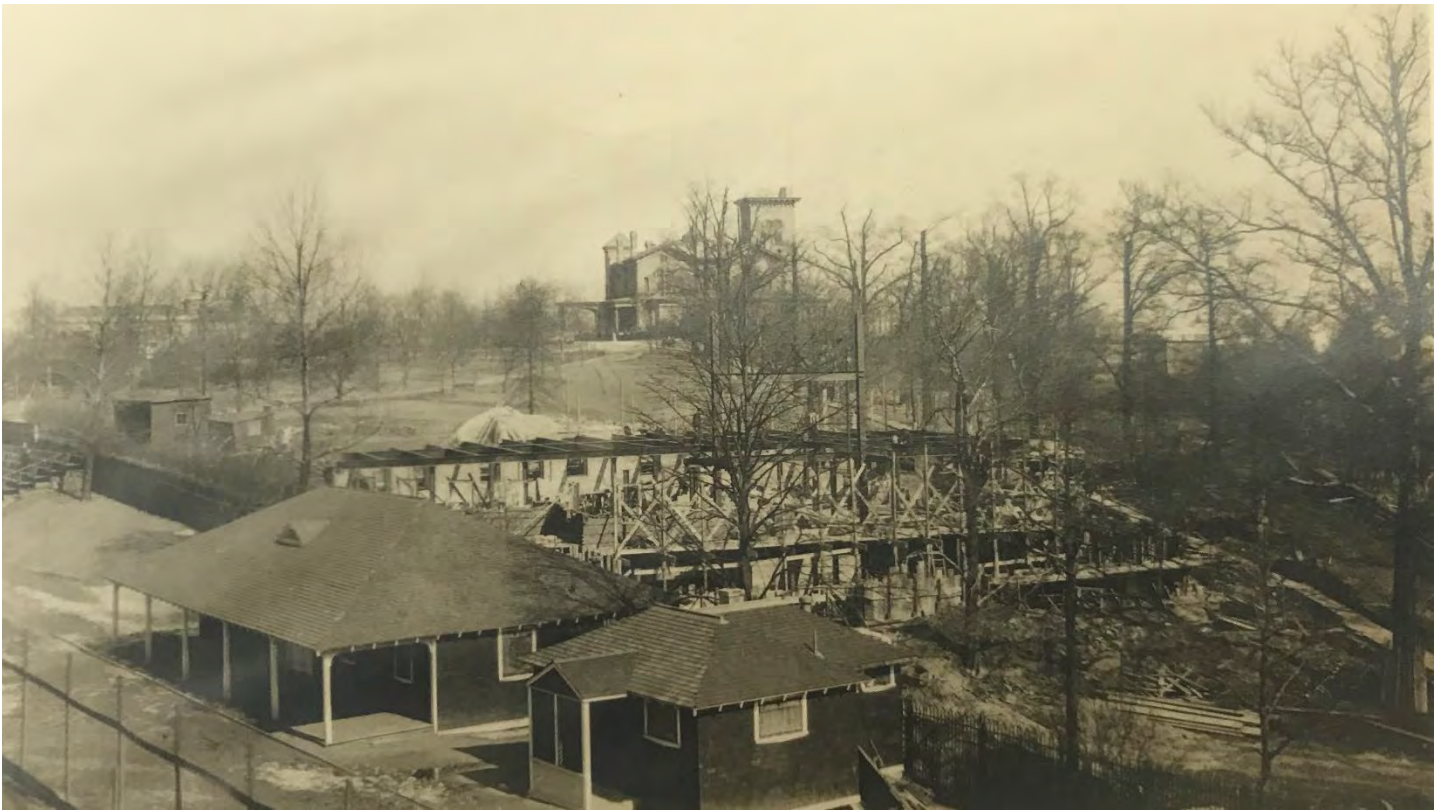
Figure 13. Walker Gymnasium under construction, 1916. Note athletic fields and field houses in the foreground and Stevens Castle in the background. Wittpenn Walk, which extended from the Sixth Street Gate to the Stevens Castle (and which is extant today) is clearly visible at the right side of the photo. (Archives and Special Collections, Stevens Institute of Technology)
