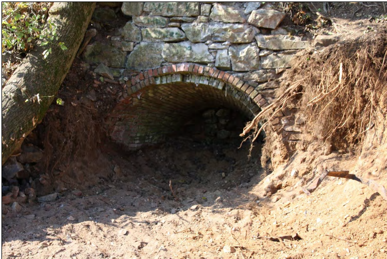
Figure 22 – Lime Kiln #2, Photographer- Bonnie Wilkinson Mark, October 8, 2016.
