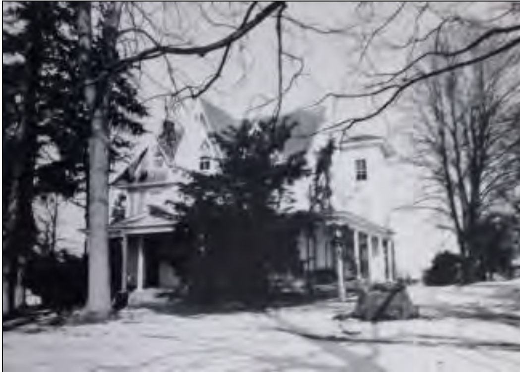
Figure 16 - Silas Eshleman House, Paradise Township, Lancaster County, Key No. 070814
