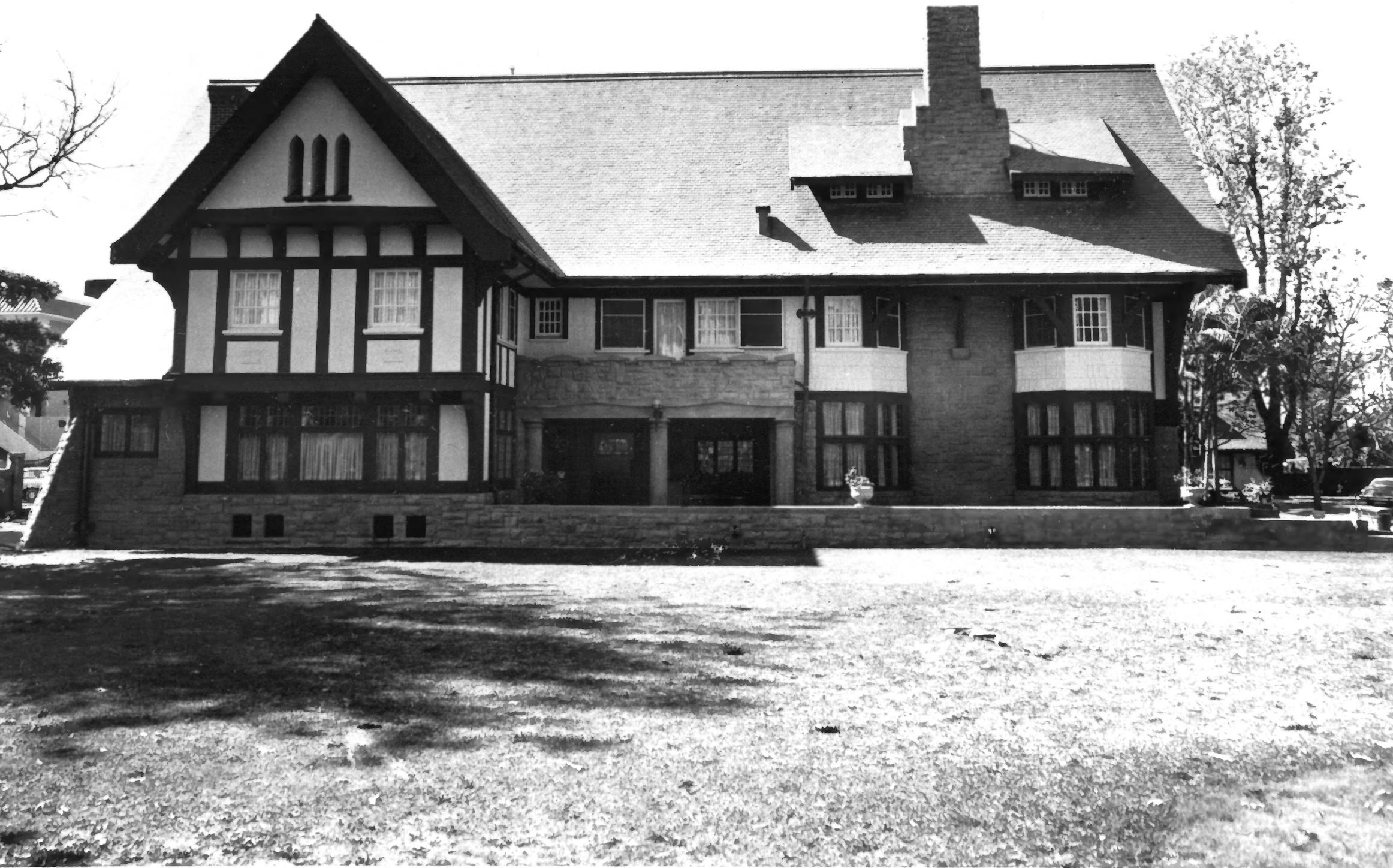
FIGURE 16: The Main Residence - east facade. The ashlar stone work is buttressed at the southern edge of the structure.
