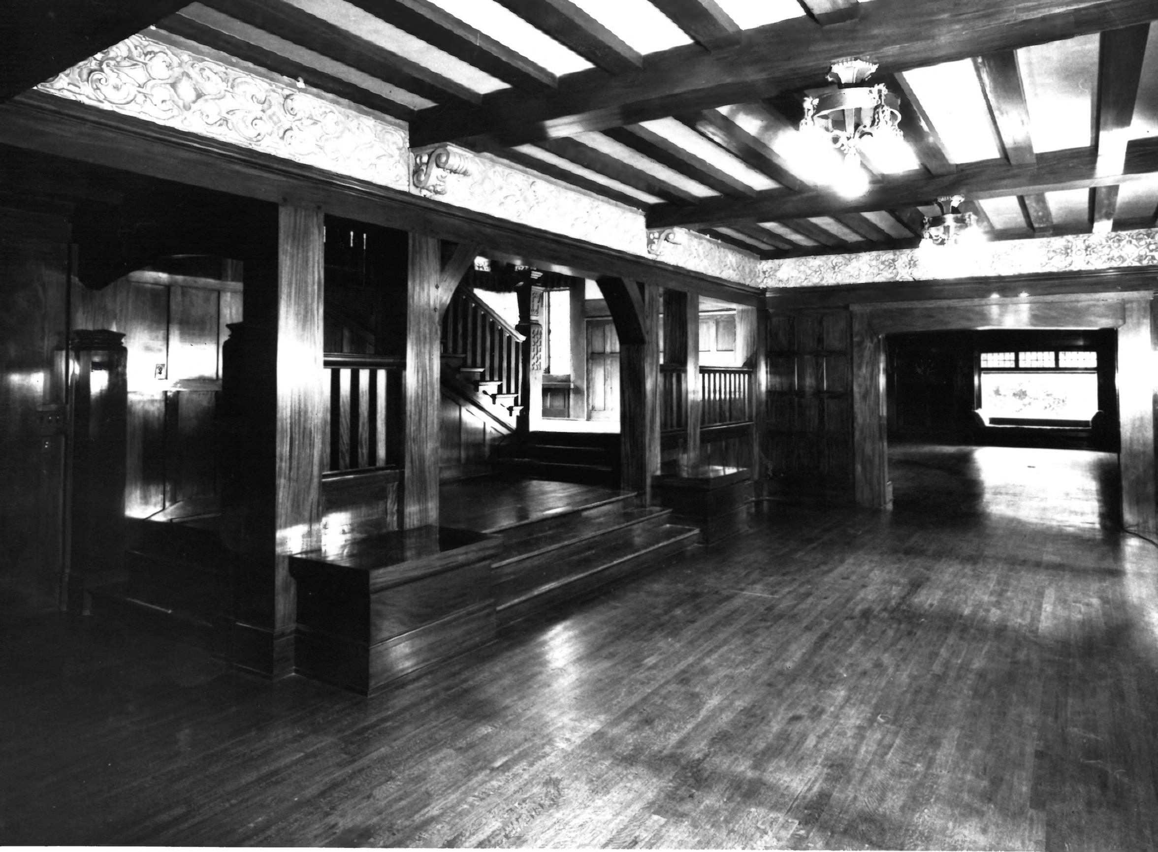
FIGURE 20: The Reception Hall features bronze painted plaster formwork at the upper register of the walls.
