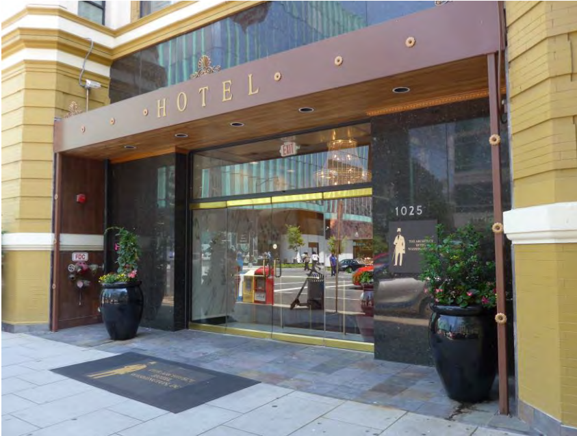
Exterior detail of entrance, west elevation Photo 6 of 17
