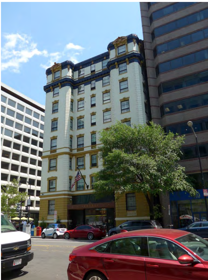
View looking northeast showing west elevation Photo 1 of 17
