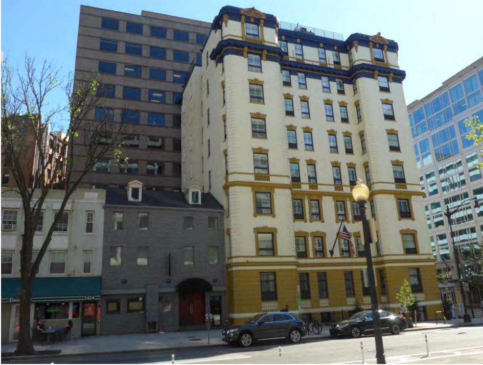
View looking south showing north and east elevations Photo 4 of 17
