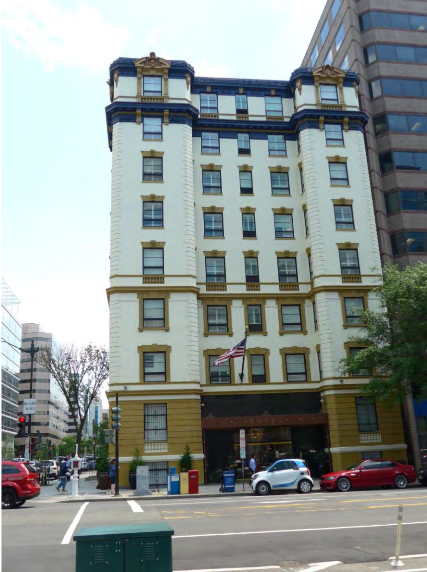
View looking east showing west elevation Photo 2 of 17
