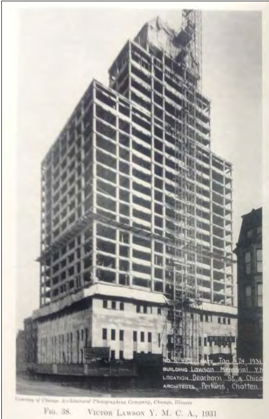
Figure 5: Victor F. Lawson House YMCA under construction, January 24, 1931
