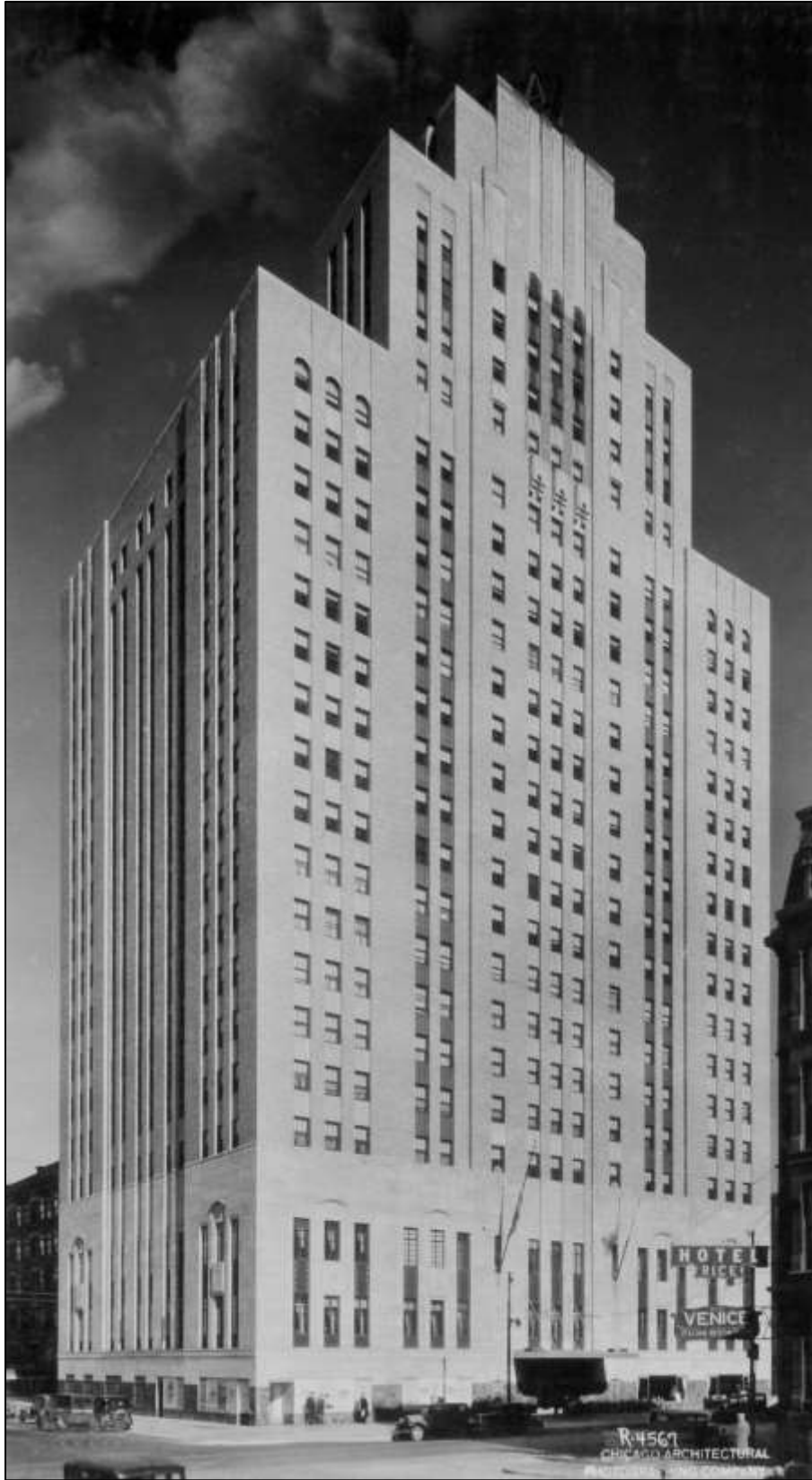
Figure 6: Victor F. Lawson House YMCA after completion, late 1931
