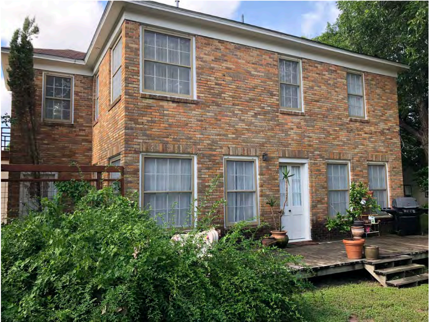
Photo 005—North elevation, looking southwest.
