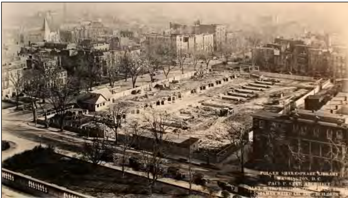
Figure 23. Undated image of the construction site (Folger Archives)
