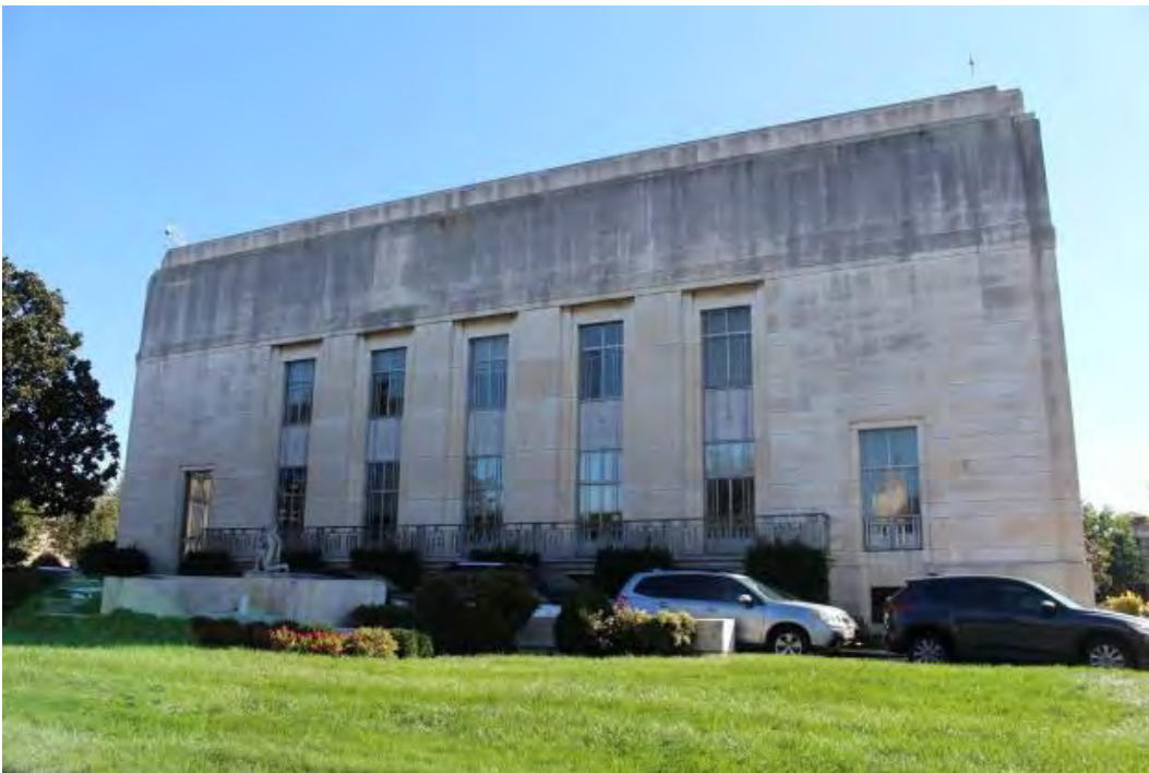
Photo #0003: DC_Washington_Folger Shakespeare Library_0003.tif West elevation, looking east.
