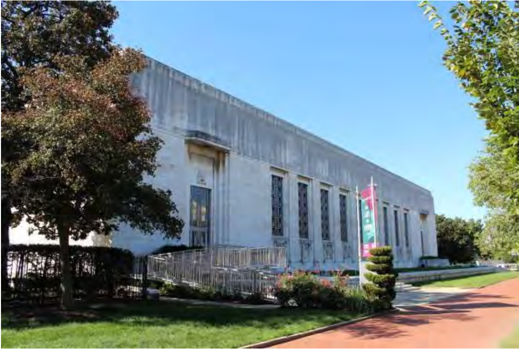
Photo #0002: DC_Washington_Folger Shakespeare Library_0002.tif North elevation, looking west.
