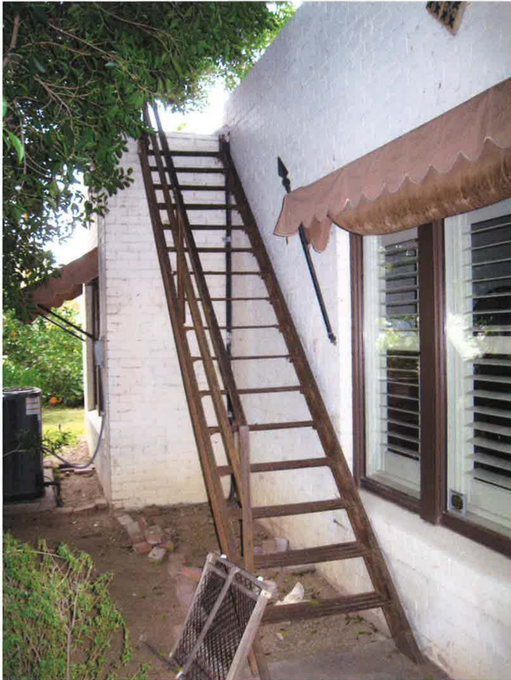
Photograph 3. Staircase to sleeping porch, facing north.
