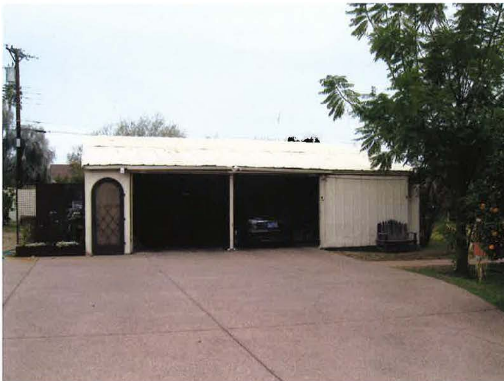
Photograph 11. Barn, facing southeast.
