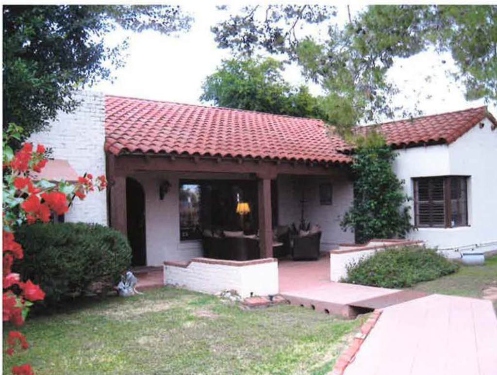
Photograph 2. Façade of front, facing east.
