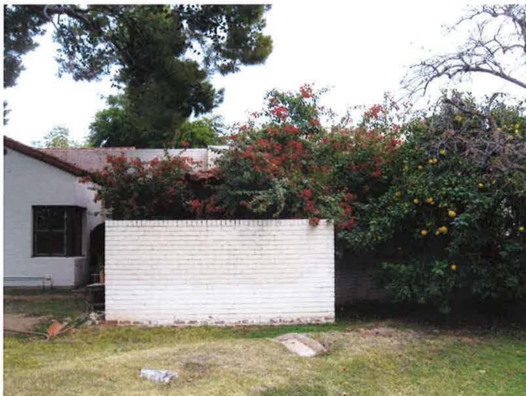
Photograph 6. South corner of 1990s east addition, facing northeast.
