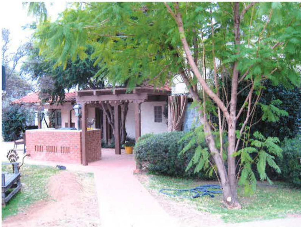
Photograph 10. Rear addition, facing southwest.
