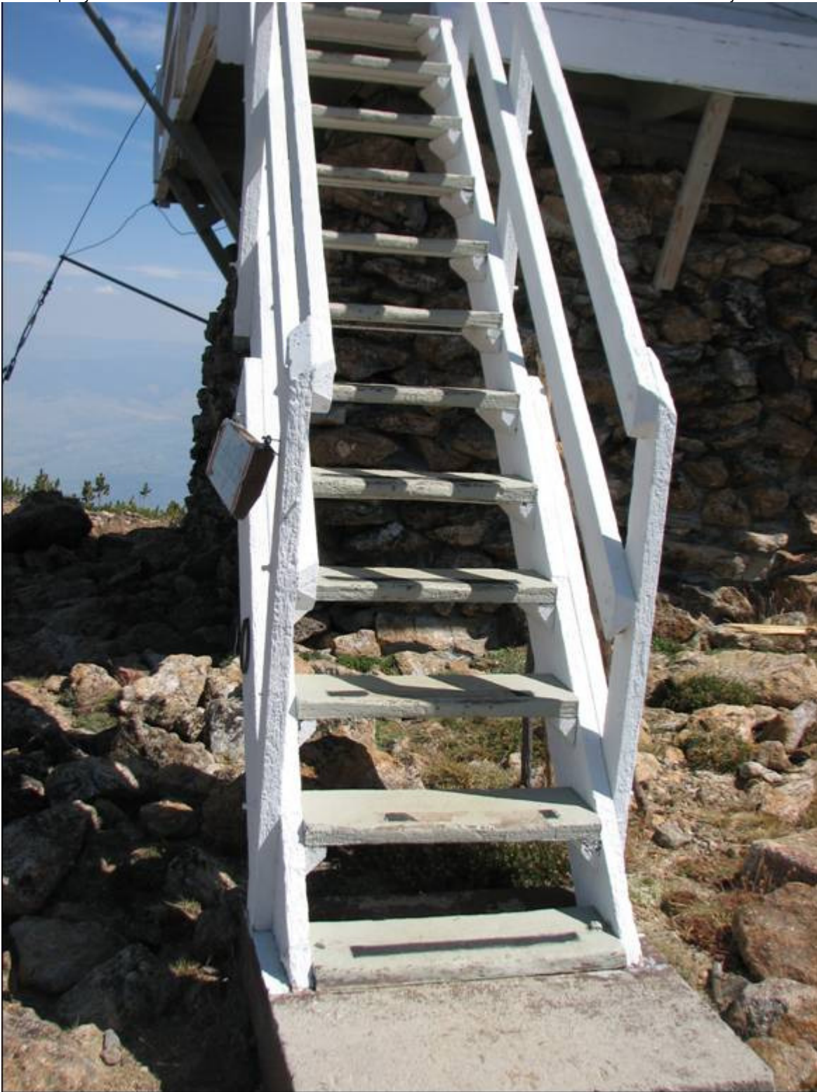
MT_ RavalliCounty_StMaryPeakLookout_0003. Looking east: detail of the stairway.
