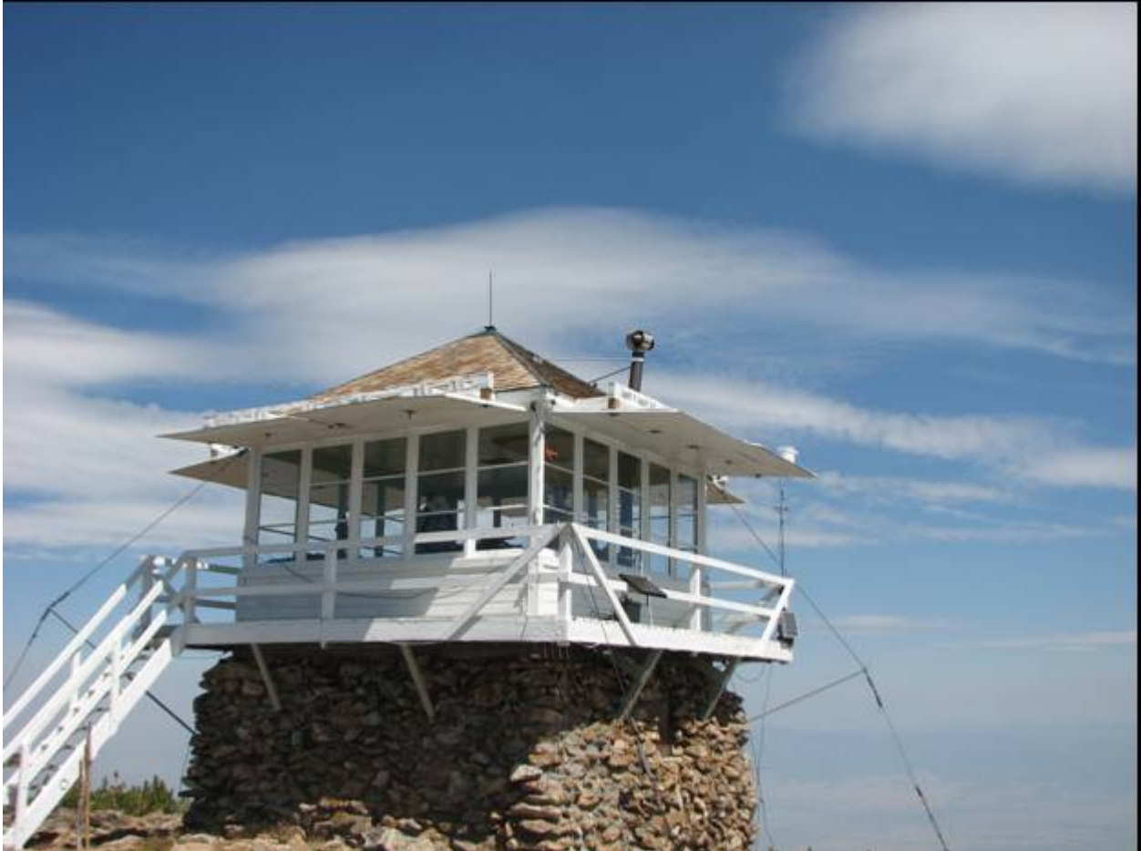
MT_RavalliCounty_StMaryPeakLookout_0002. Looking northeast to the west and south walls of the lookout.
