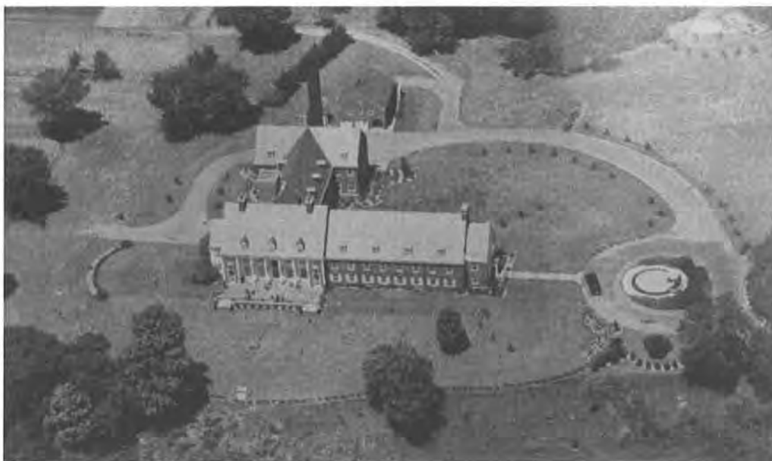
Figure 14: Royal Neighbors National Home, aerial view, c. 1962. Photographer unknown. The garage shown behind the building is no longer extant. Source: The Royal Neighbor , July 1962.
