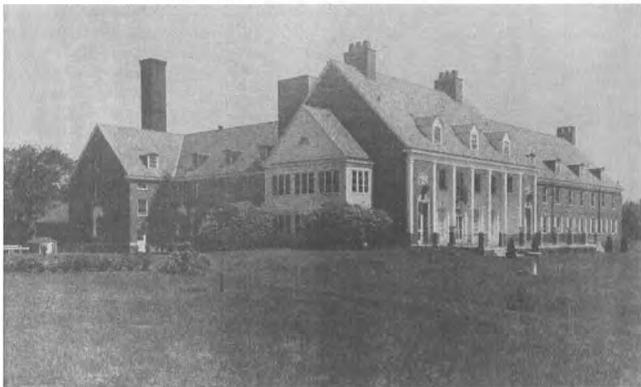
Figure 17: Royal Neighbors National Home, south corner, c. 1974. Photographer unknown. Source: The Royal Neighbor , April 1974.
