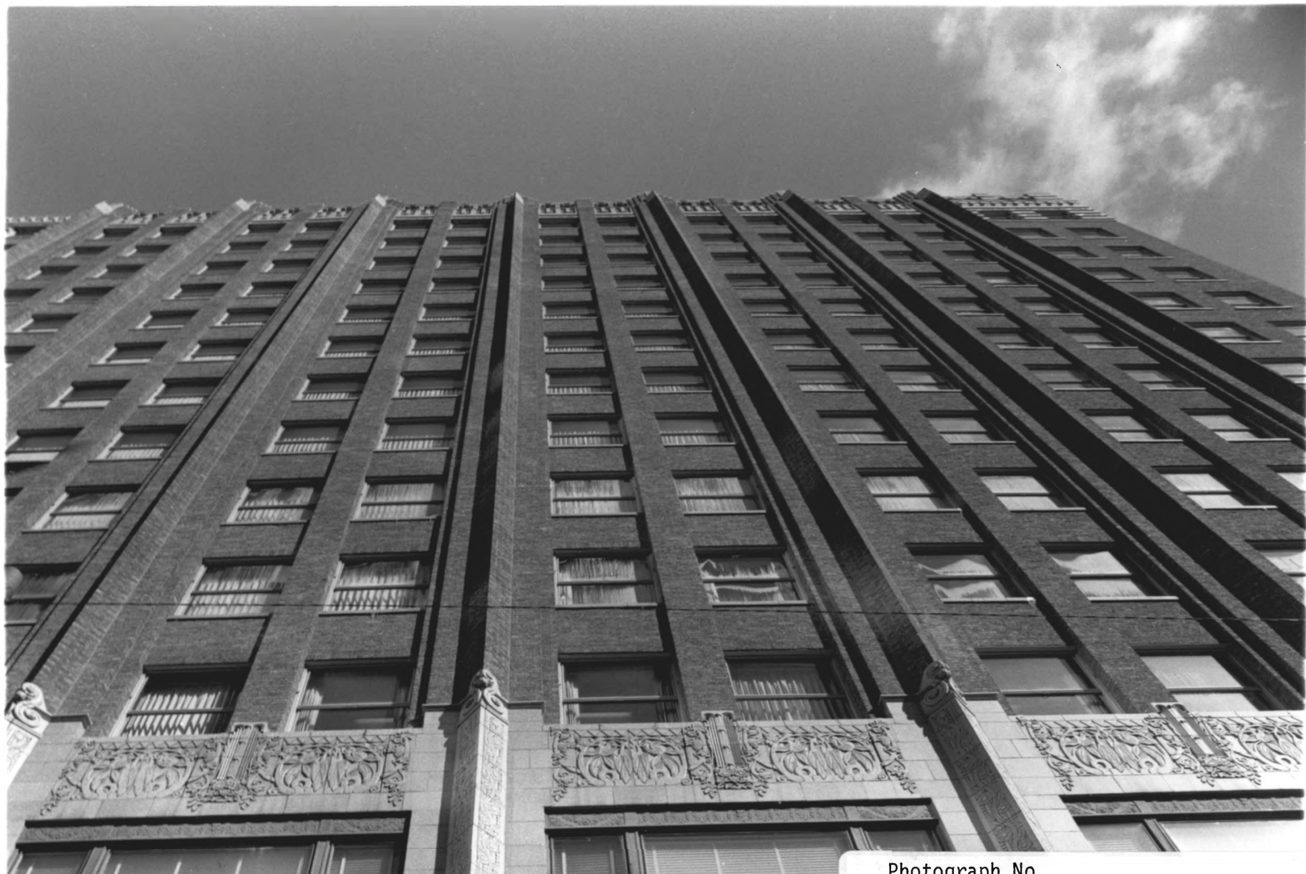
Photograph No. Philcade Building January 15, 1985 Detail of West Elevation
