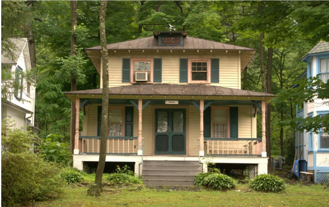
Photo 9. "Sunshine," cottage #8, facing north.
