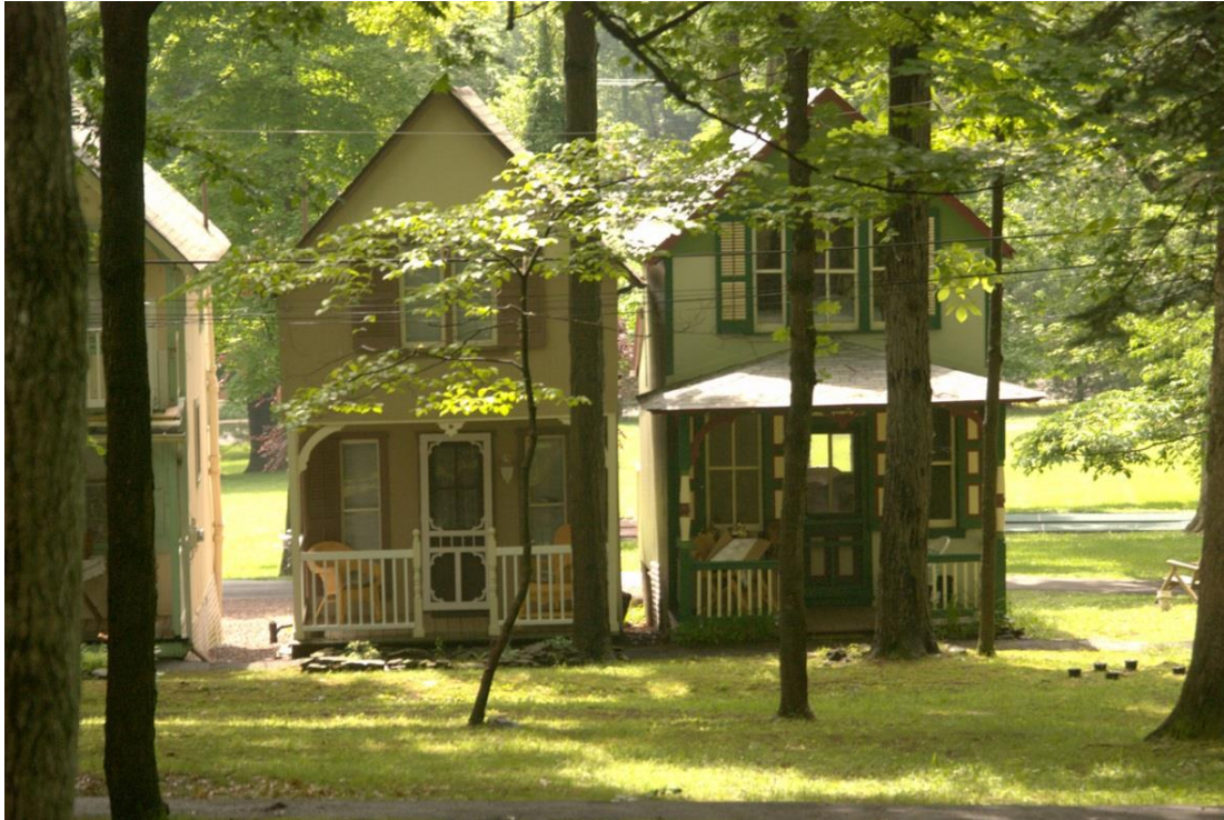
Photo 3. Cottages at west corner of commons, main elevation, facing southwest.
