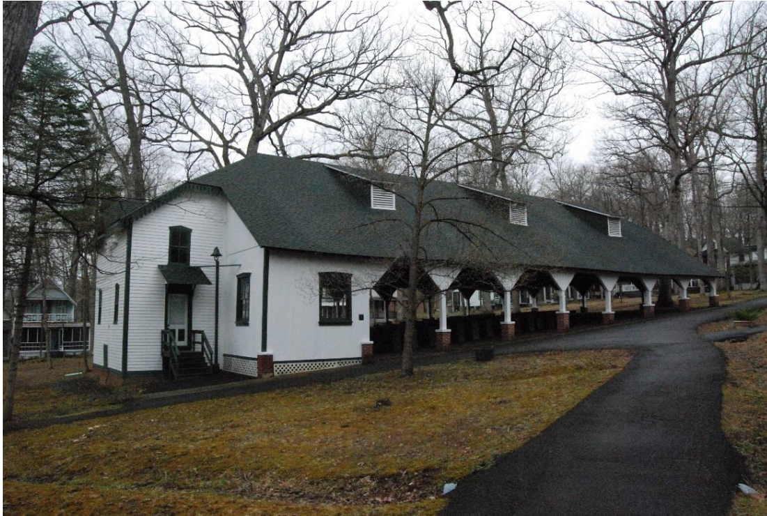
Photo 1. Auditorium, facing west
