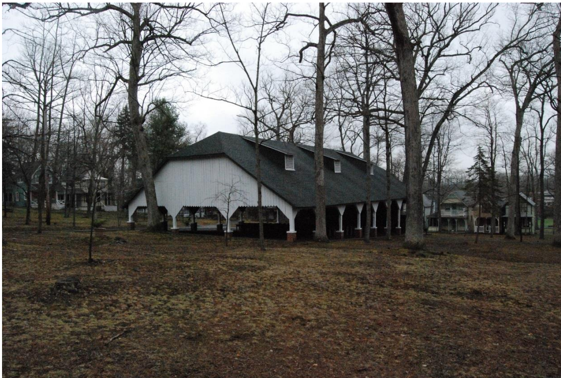
Photo 13. North elevation of Auditorium.
