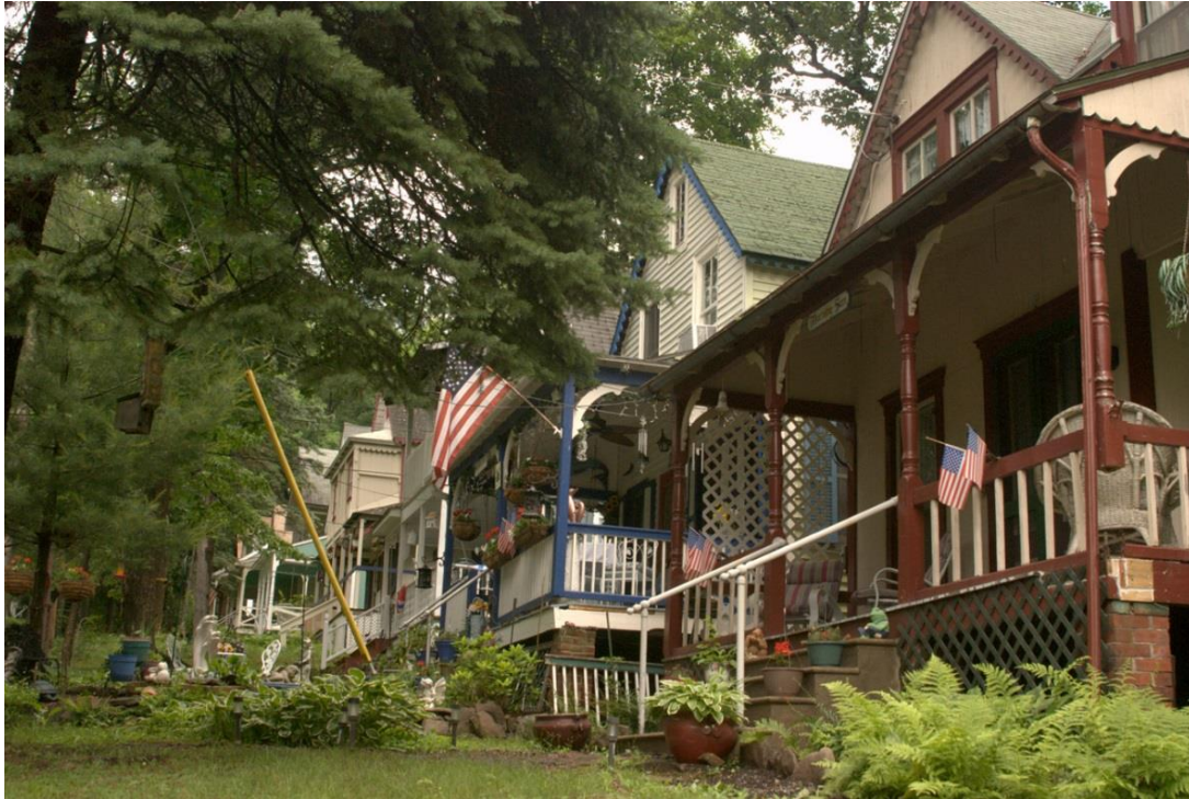
Photo 5. Cottages along northeast side of commons, facing north.
