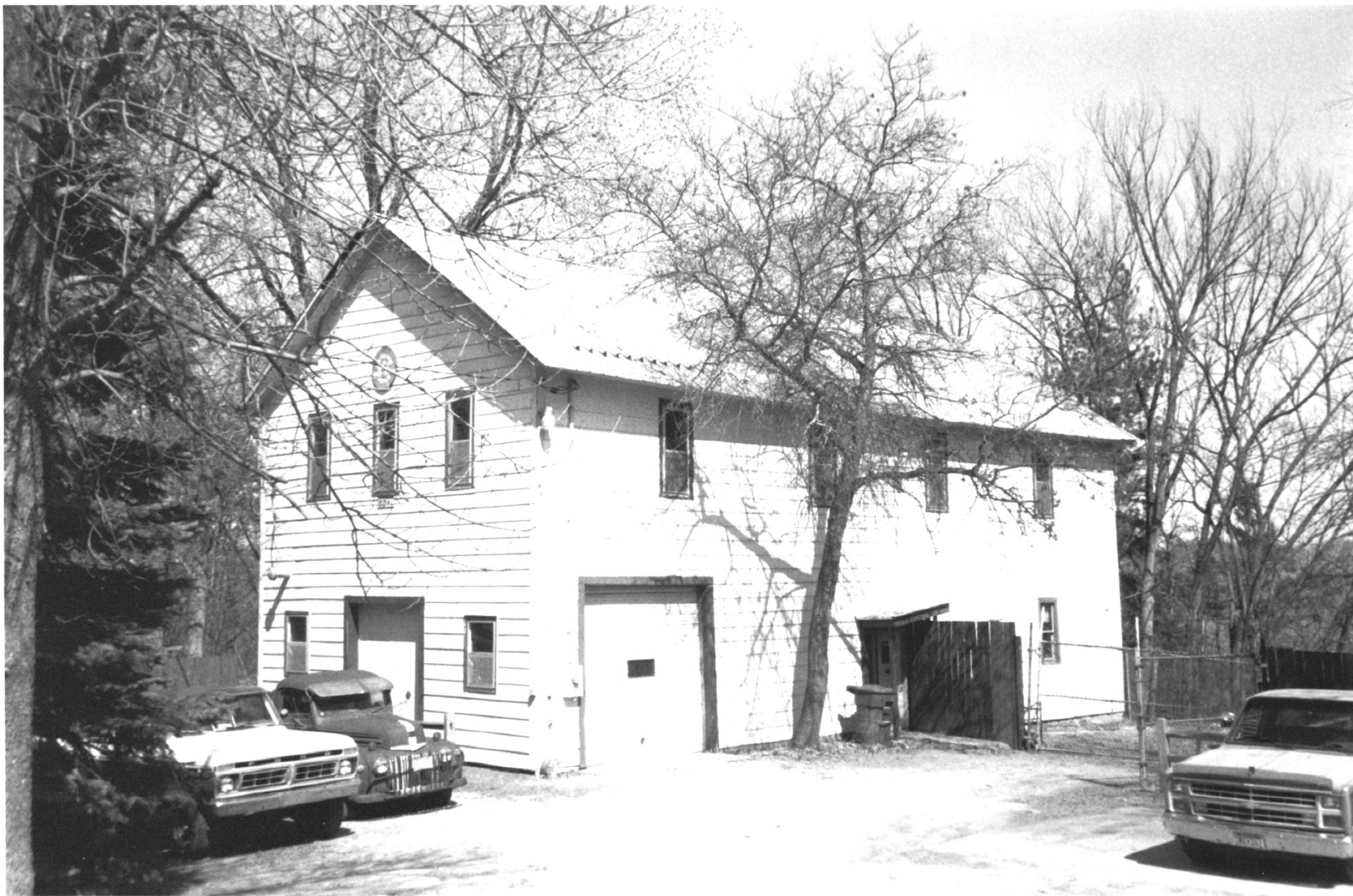
BERGSTEIN SHODDY MILL & WAREHOUSE (WAREHOUSE)
