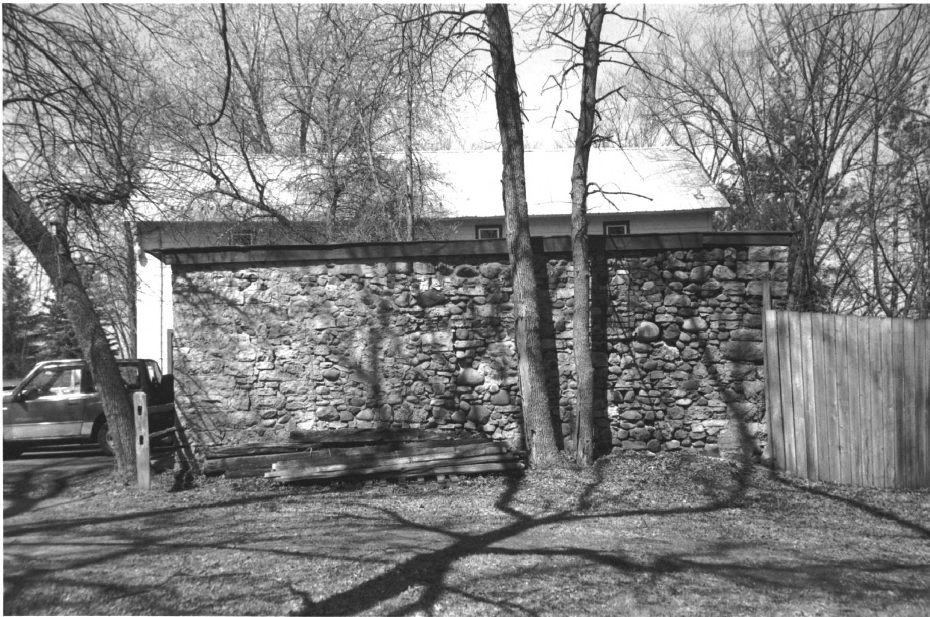
BERGSTEIN SHODDY MILL & WAREHOUSE (SHODDY MILL) WASHINGTON CO., MN
