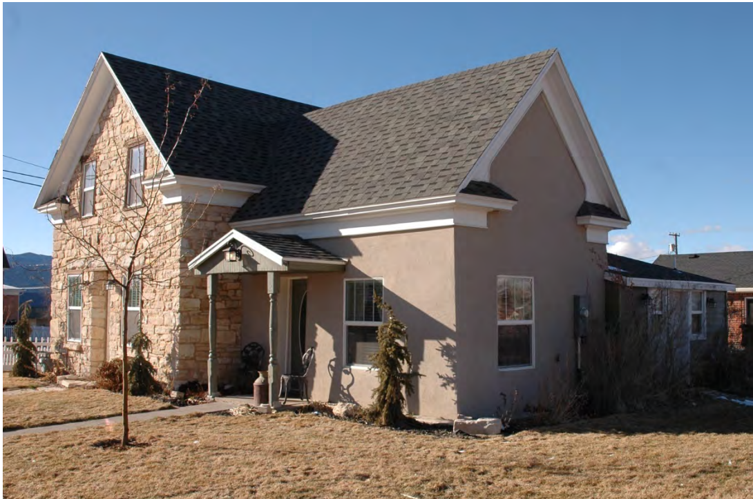
Photograph 3 South and east elevations. Camera facing northwest.
