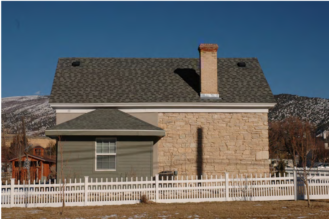
Photograph 5 West elevation. Camera facing east.
