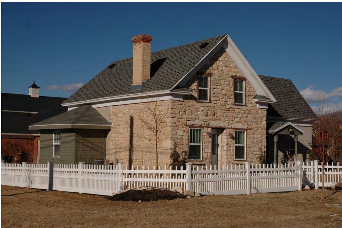
Photograph 6 South and west elevations. Camera facing northeast.
