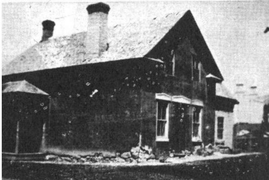
Figure 1 Pectol-Works House, circa 1910 South and west elevations. Camera facing northeast. Photograph courtesy Works Family.
