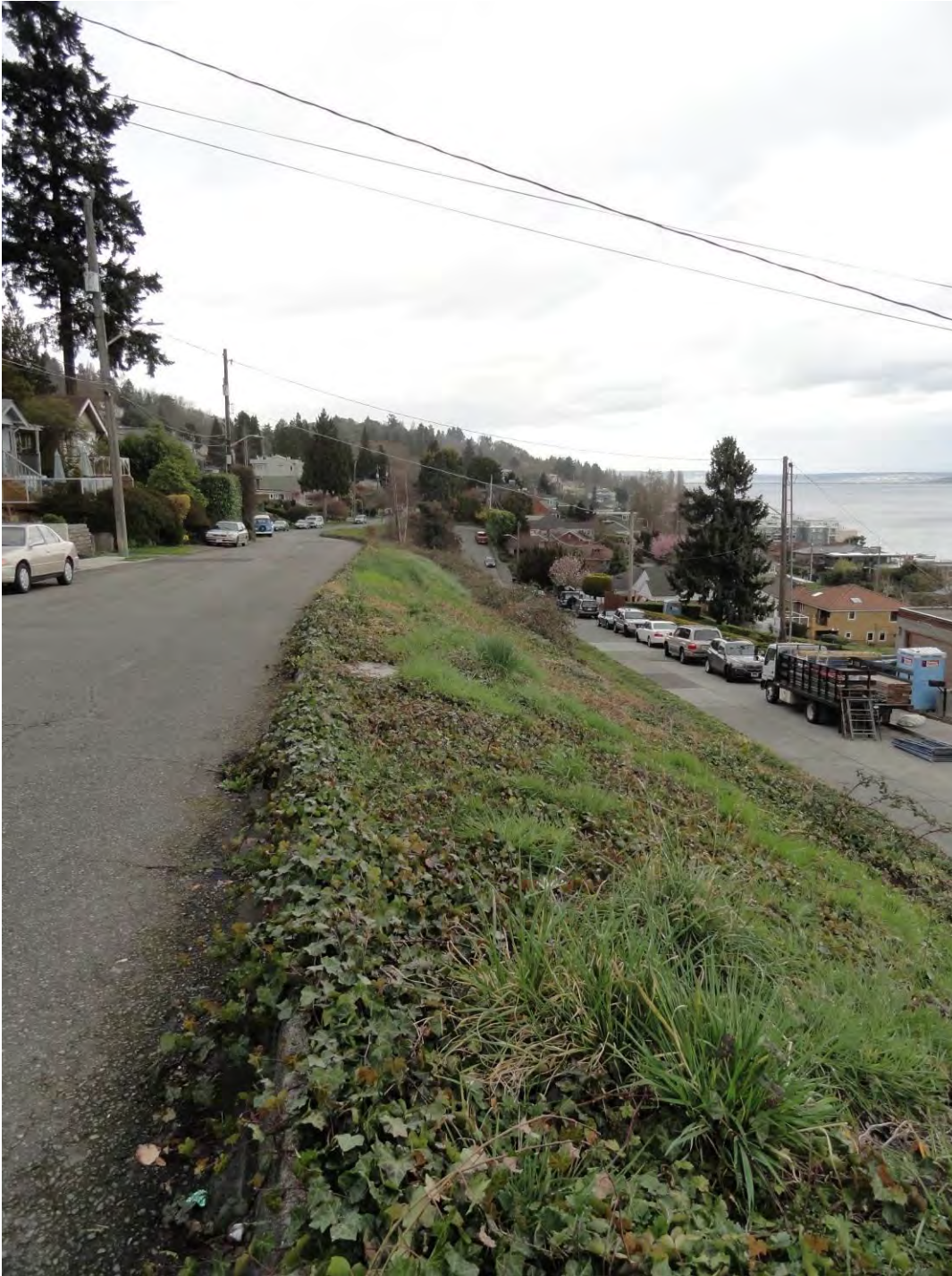
Photo 13. WA_KingCounty_LakeWashingtonBoulevard_0013. The South Charles Street Bed (contributing resource no. 3), view north.
