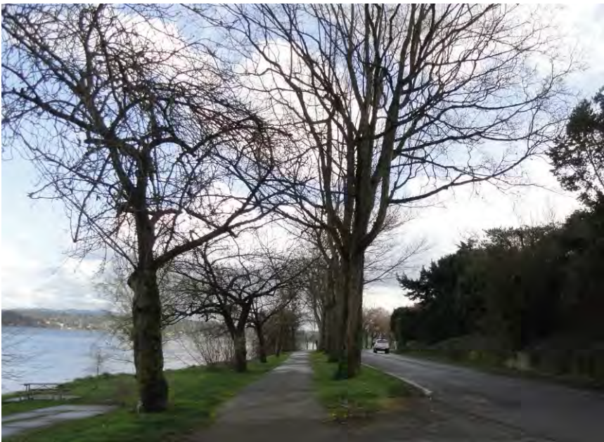
Photo 21. WA_KingCounty_LakeWashingtonBoulevard_0021. Lake Washington Boulevard and the Lake Washington Footpath (contributing resource no. 7) and the Lake Washington retaining wall (contributing resource no. 8), view south.
