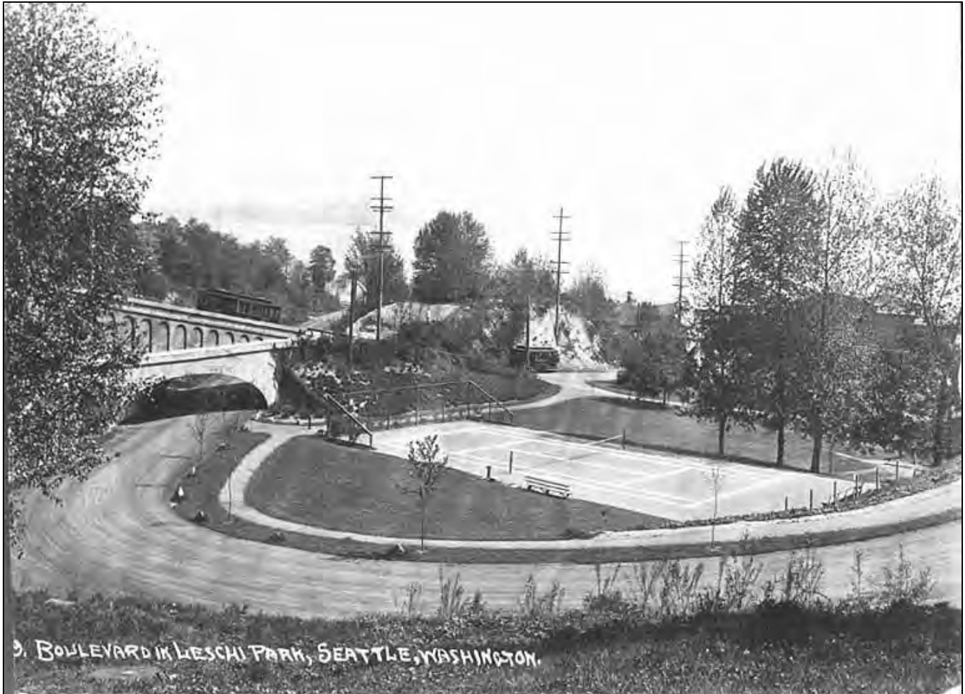
Figure 9. Lake Washington Boulevard in Leschi Park showing Yesler Way Cable Trestle. Image SEA2014, courtesy of the Seattle Photograph Collection via the University of Washington Library Digital Collections.
