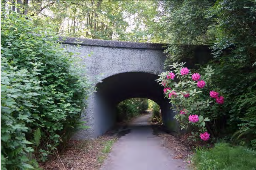
Photo 18. WA_KingCounty_LakeWashingtonBoulevard_0018. Colman Park Overpass No. 3 (contributing resource no. 6), view east.
