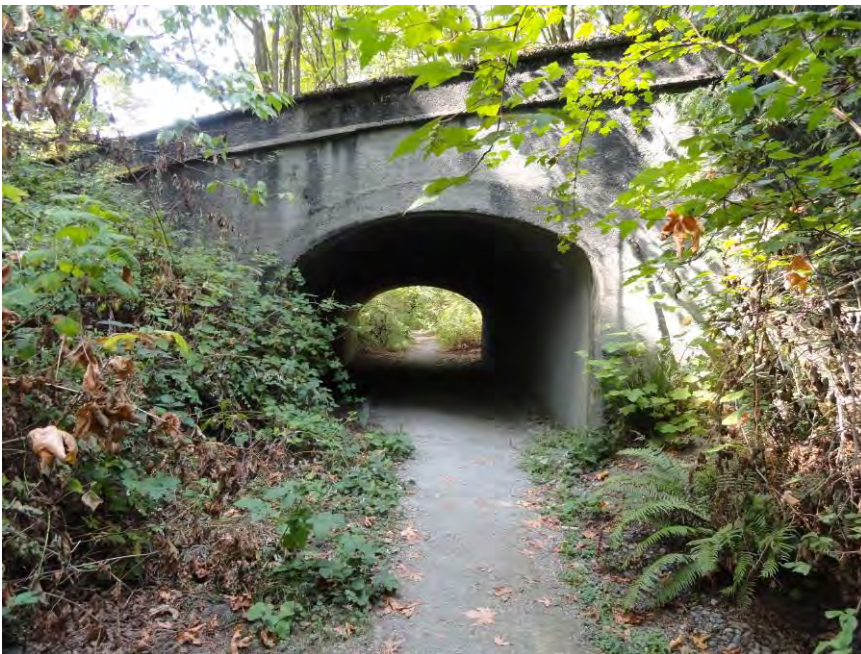
Photo 17. WA_KingCounty_LakeWashingtonBoulevard_0017. Colman Park Overpass No. 2, view north.
