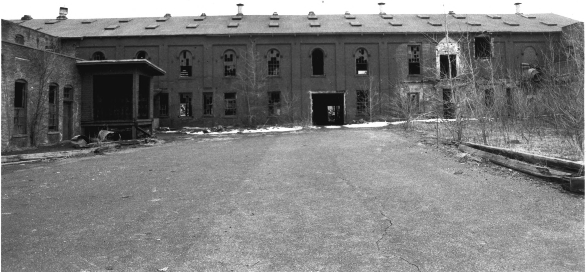
Photo 14: New Power Mill, North Side.
