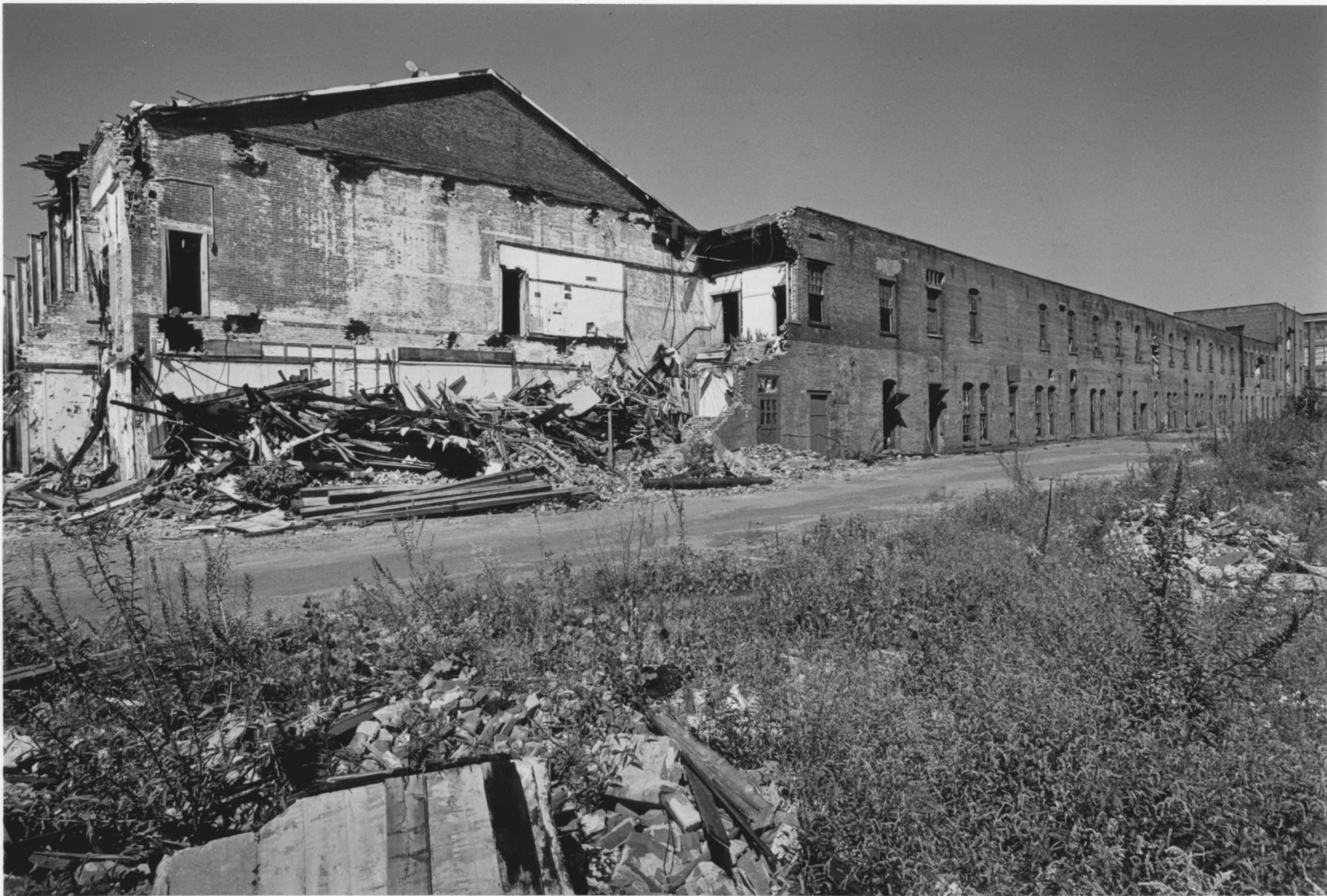
Photo 11: New Power Mill, East End (Dye House at right).
