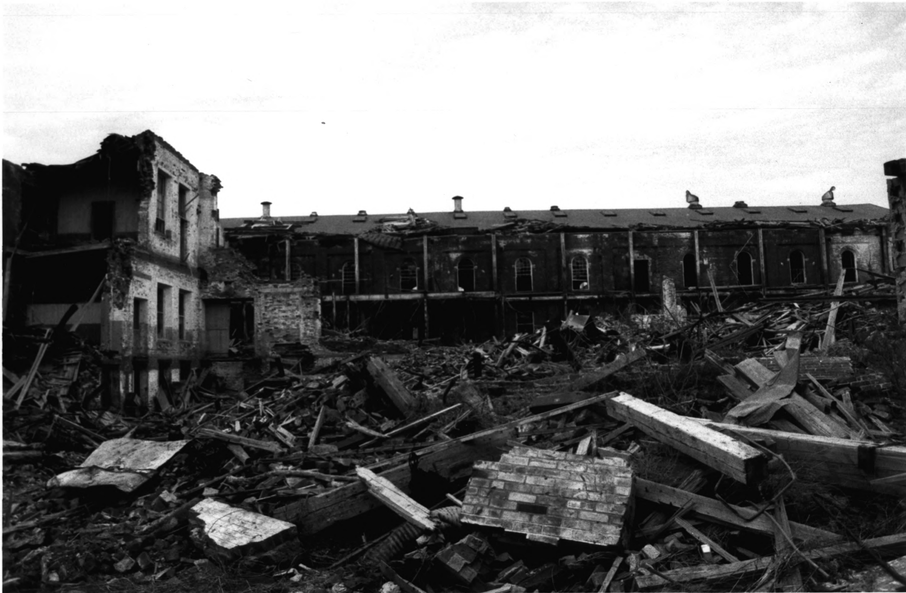
Photo 12: New Power Mill, South Side, with demolition of adjacent buildings in foreground.
