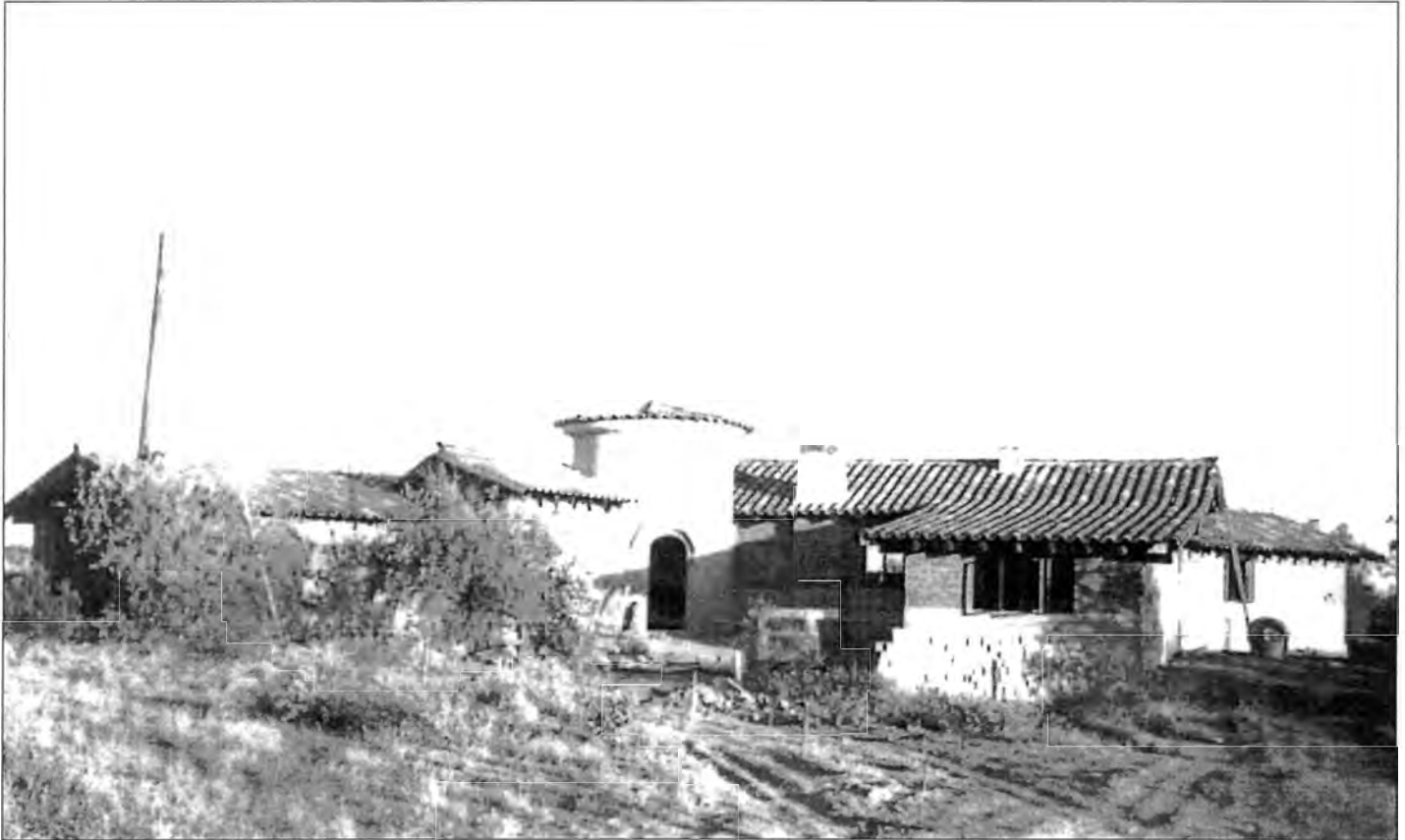
Figure 1. Harelson House under construction, ca. 1940. Courtesy of Peggy Duncan.
