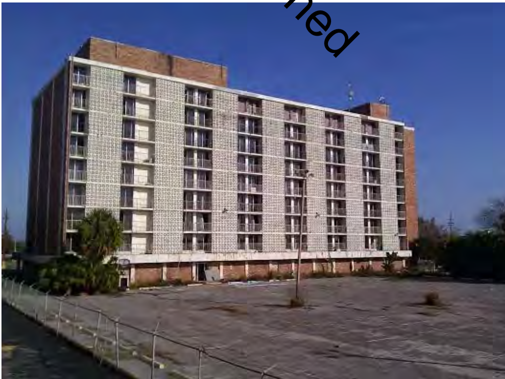
Figure 2. 2015 Photo of Holiday Inn at 6324 Chef Menteur Hwy, New Orleans Hamilton, Rob. "Highrise Inn at 6324 Chef Menteur Highway, New Orleans." Google. March 13, 2015. Accessed April 17, 2018. https://plus.google.com/RobHamilton79/posts/ZMghGaGHurM .
