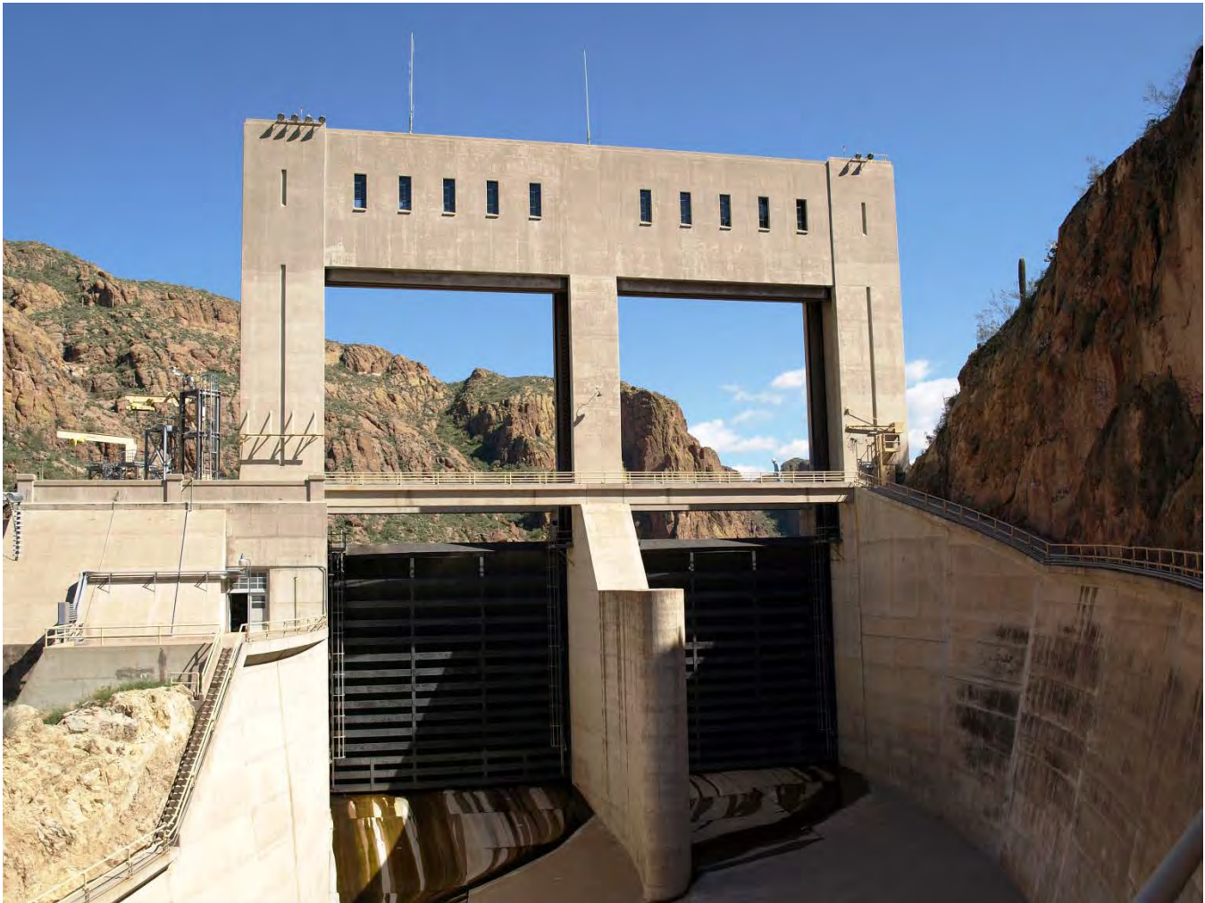
Photo 5: Spillway gatehouse looking east.
