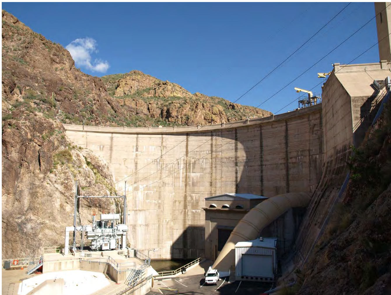
Photo 3: Mormon Flat Dam looking northeast.
