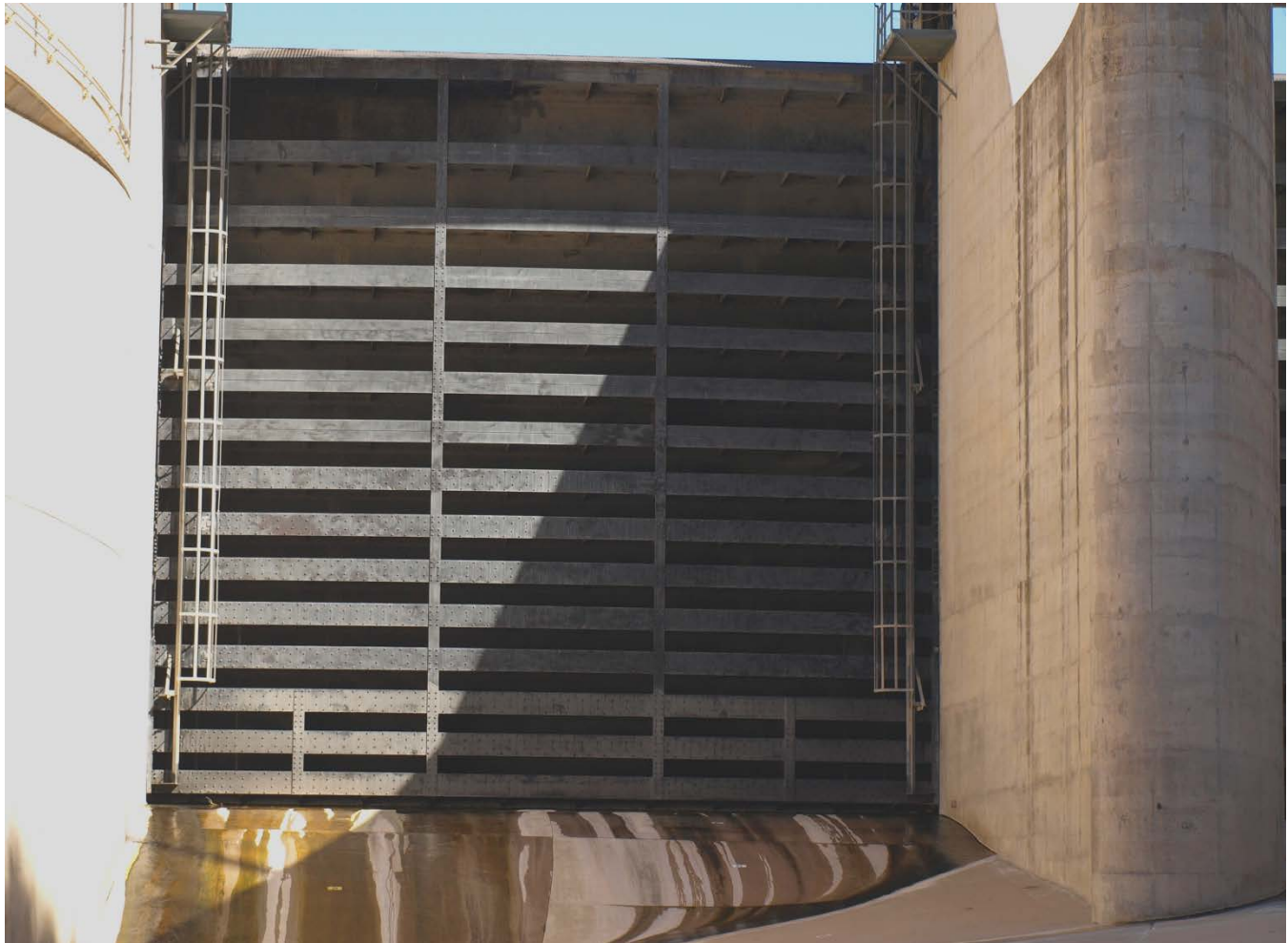
Photo 6: Spillway gates looking east.
