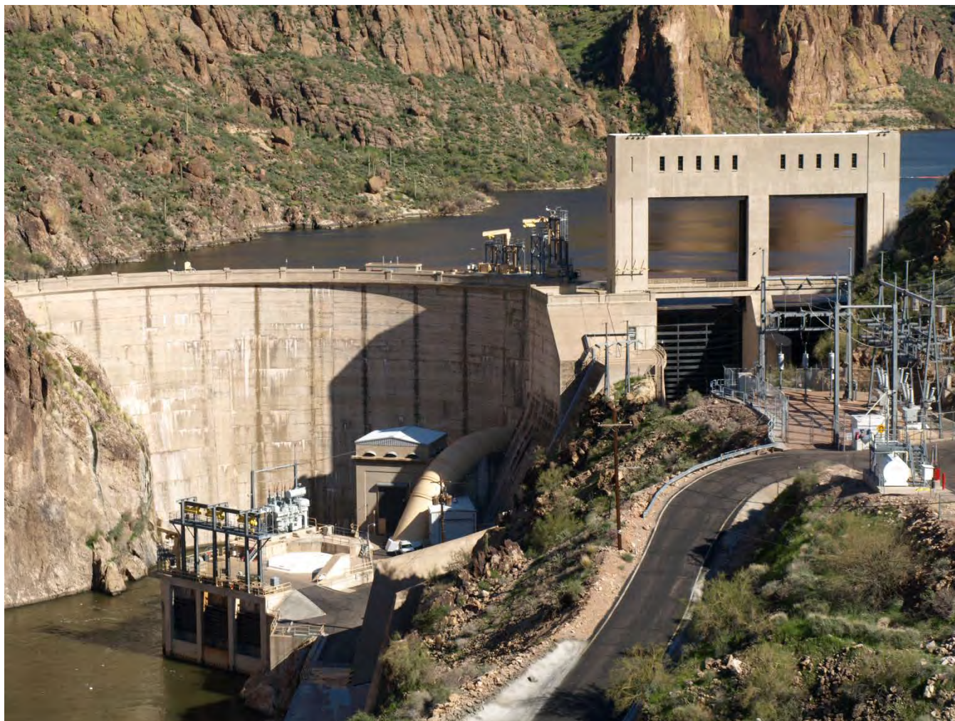
Photo 2: Mormon Flat Dam looking east.
