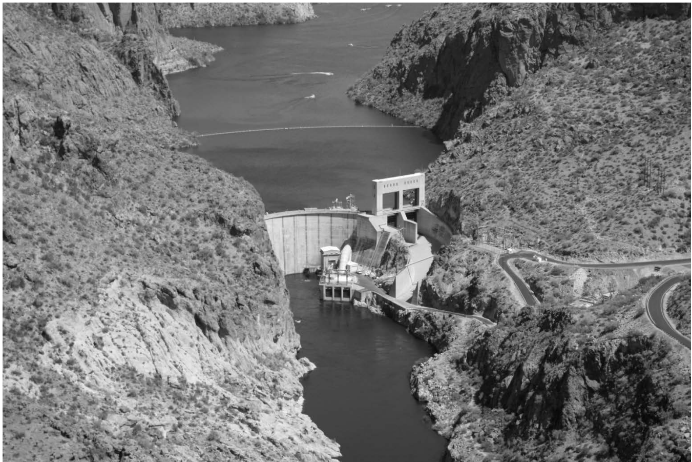
Photo 1: Mormon Flat Dam and Canyon Lake aerial looking east.
