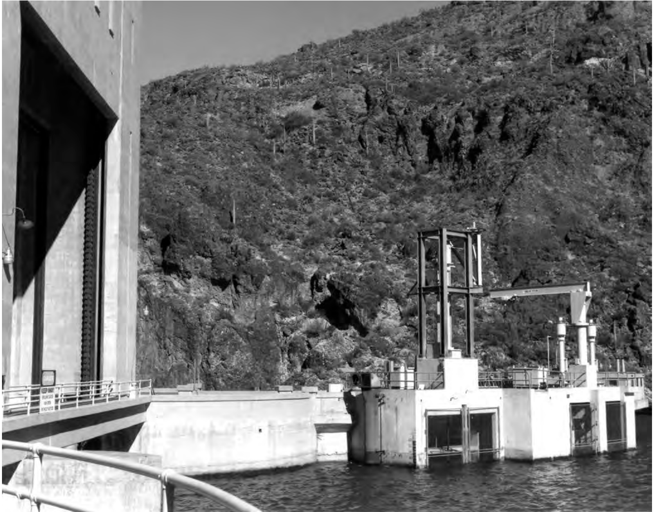
Historic Photo 12: Upstream face of spillway superstructure at left, and HEFU service tower at right, 1988. Mark Durben photo courtesy of the SRP.
