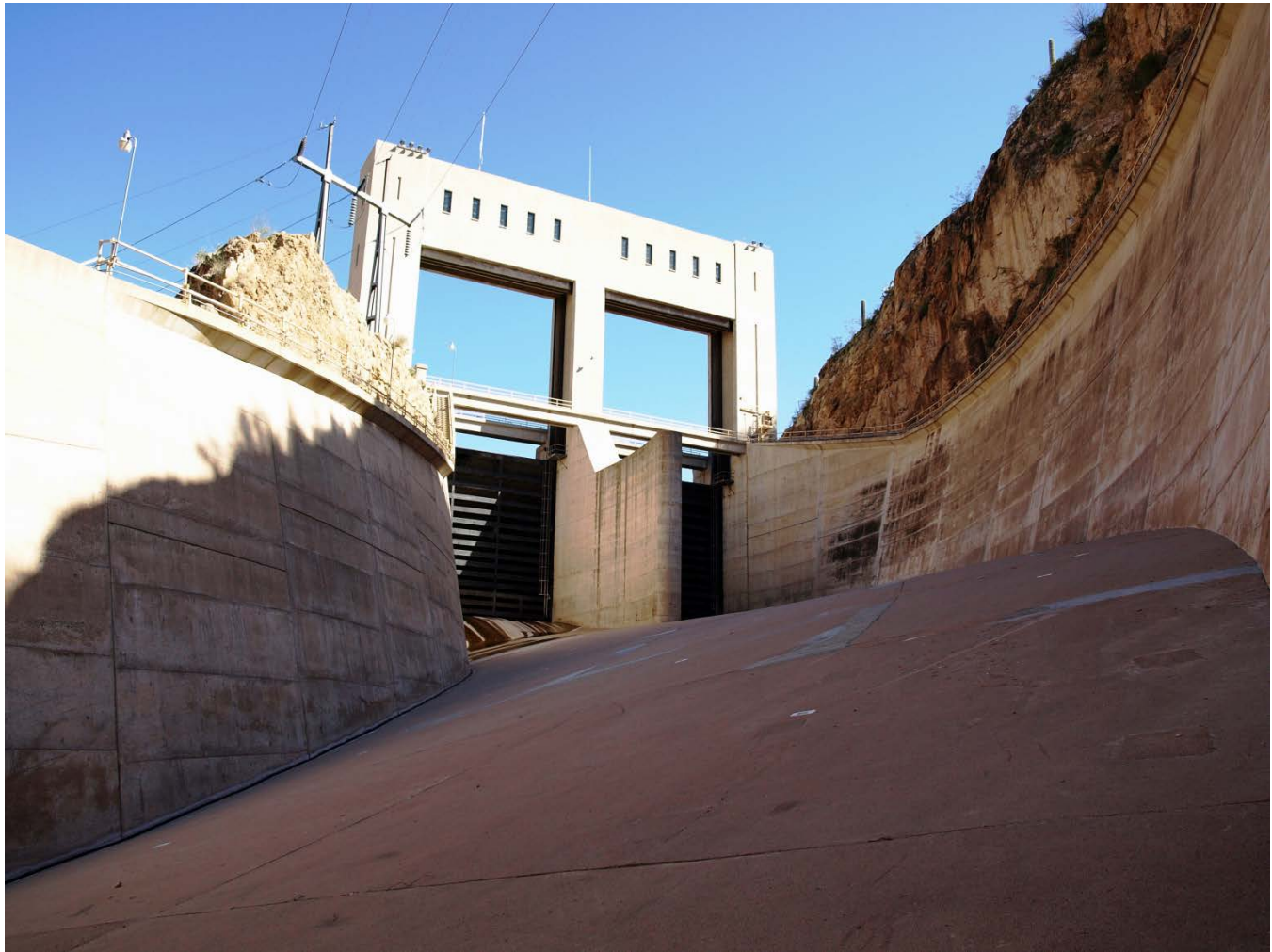
Photo 7: Mormon Flat Dam spillway and gates.
