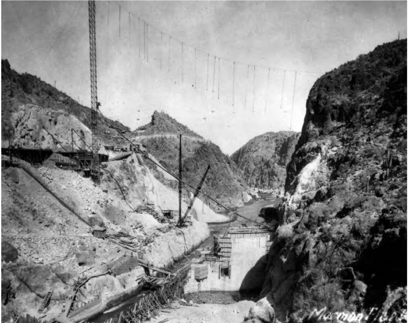
Historic Photo 4: Upstream view showing diversion flume at lower left and mixing plant at left center, June 1924. Photo courtesy of the SRP.
