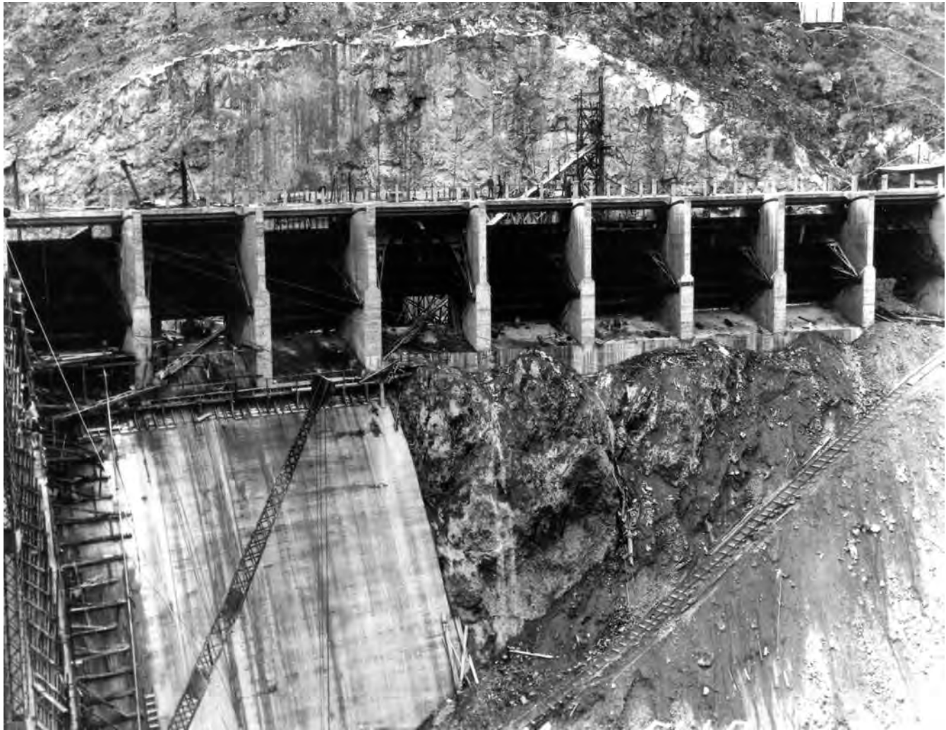
Historic Photo 7: Downstream view of spillway Taintor gates, February 1925. Photo courtesy of the SRP.
