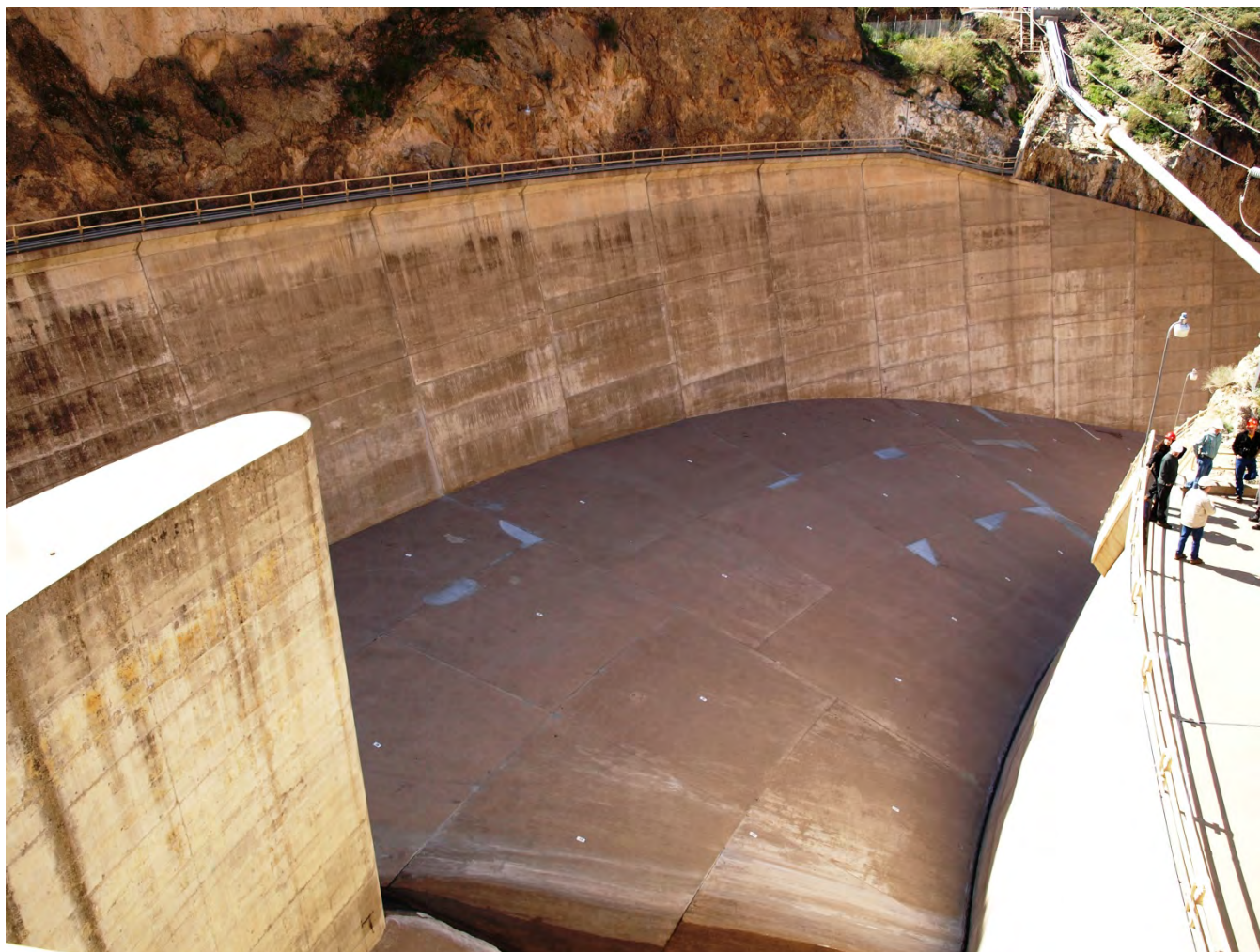
Photo 8: Mormon Flat dam spillway from crest.
