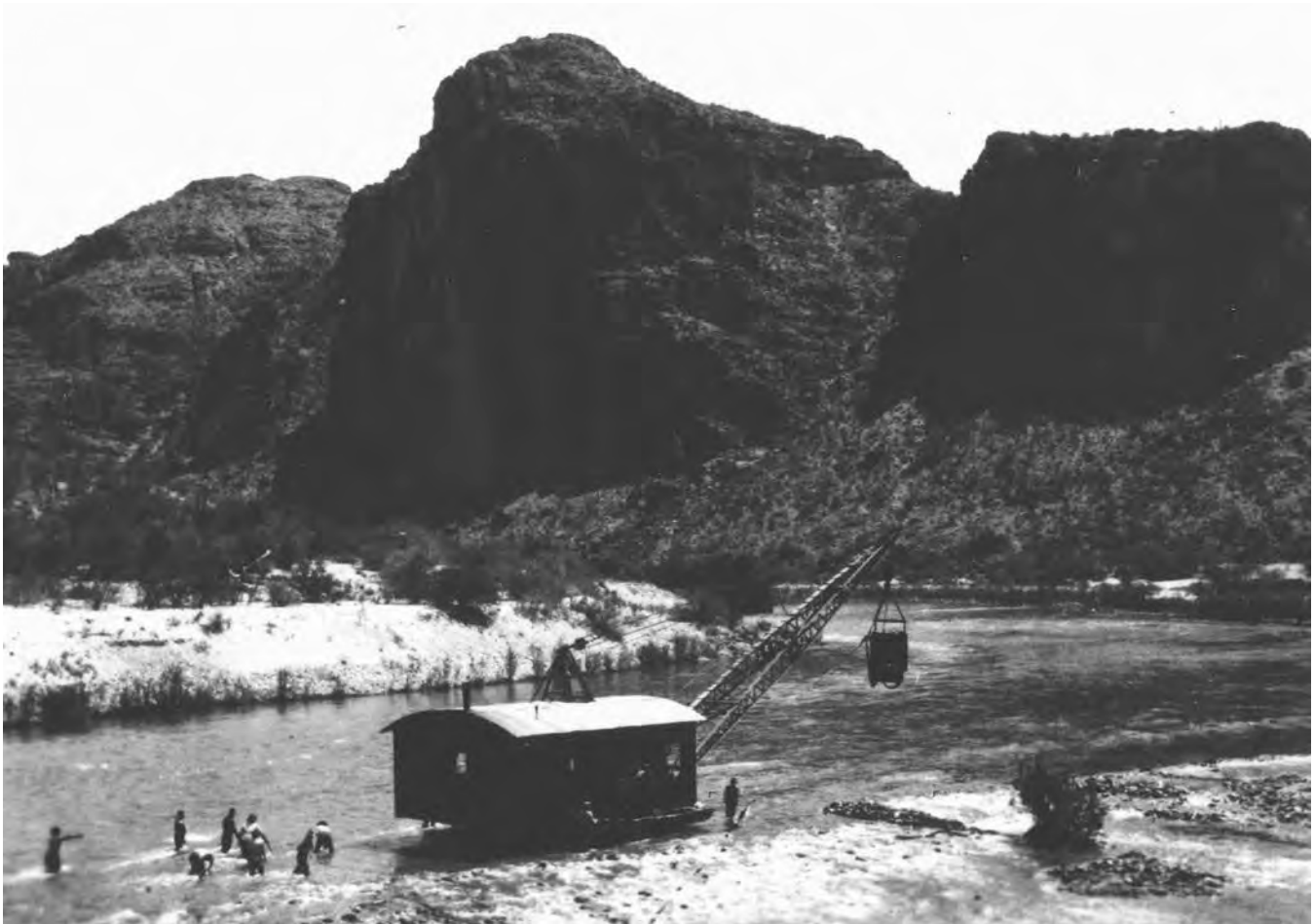
Historic Photo 3: Monighan dragline at work in the Salt River at Mormon Flat, 1923. Photo courtesy of the SRP.
