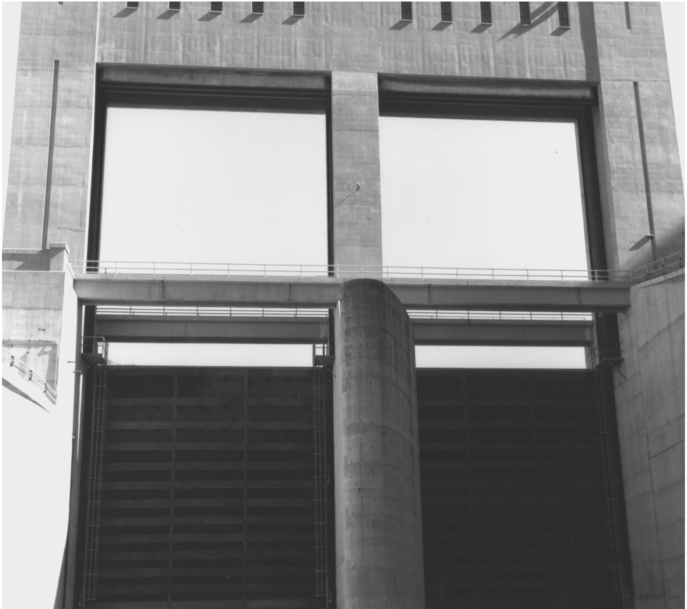
Historic Photo 11: Downstream side of the Mormon Flat spillway gates and superstructure, 1988. Mark Durben photo courtesy of the SRP.
