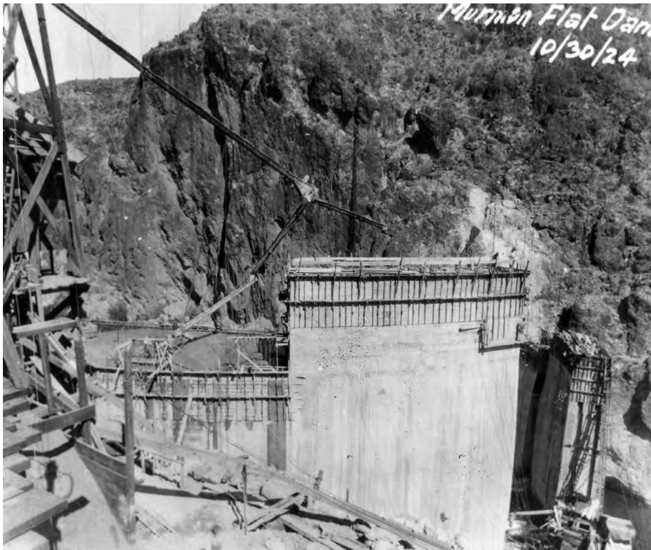
Historic Photo 5: View of upstream face and concrete tower chutes. Photo taken on October 30, 1924. Photo courtesy of the SRP.
