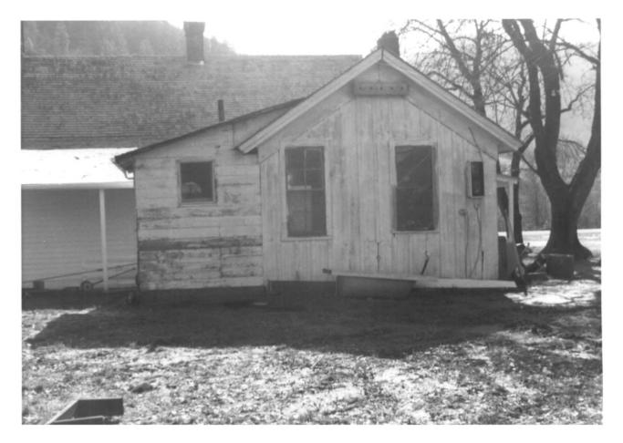
White (John B.) House 3 of 7 Rock Point, Jackson County, Oregon North elevation, showing board and batten siding on end of ell and later lean-to addition.
