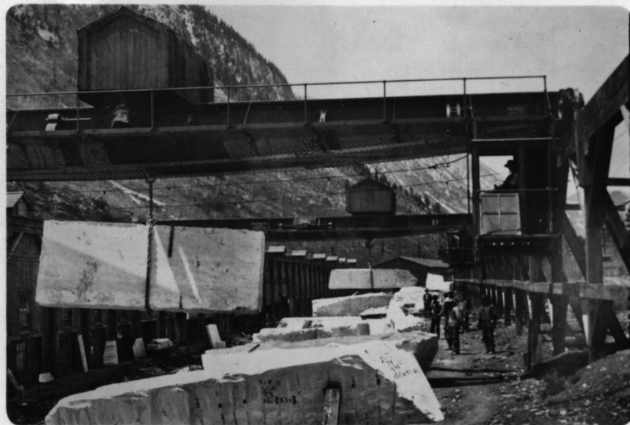
STAGING YARD AT FINISHING MILL IN MARBLE, COLO
