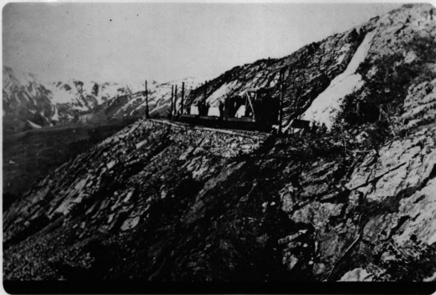
ELECTRIC TRAM BRINGING QUARRIED STONE AROUND WINDY POINT ON FOUR MILE TRIP TO FINISHING MILL.
