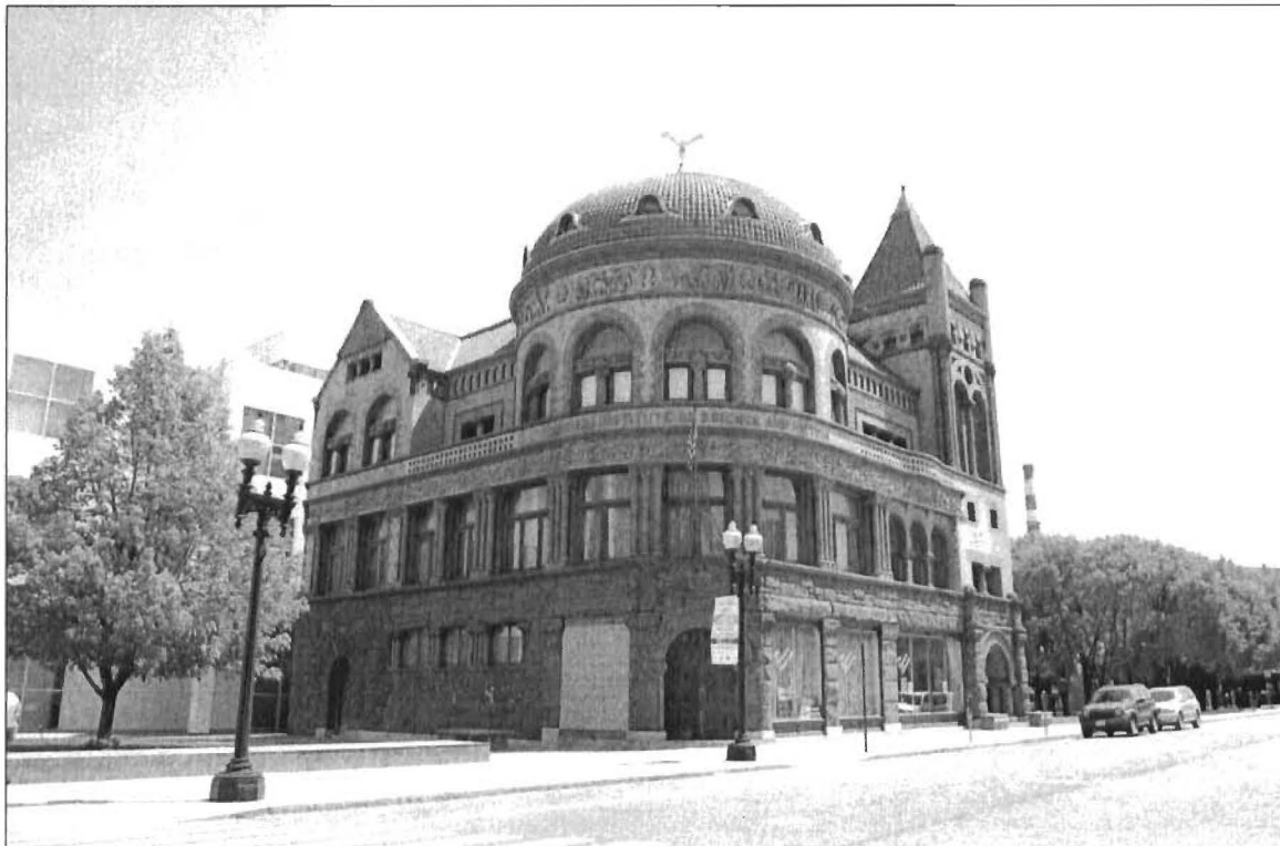
1 of 8. View looking southeast from Main Street at the north and west elevations.
