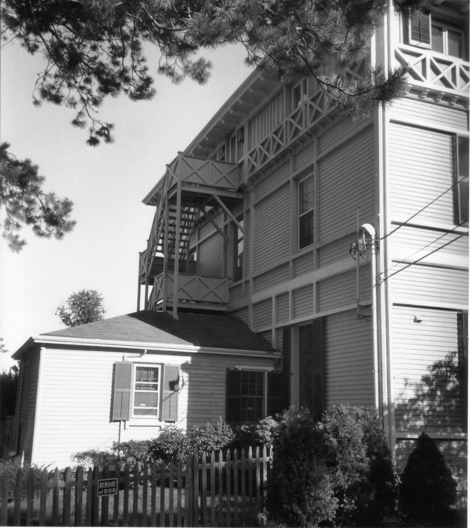
Hamilton Hoppin House Newport County, Middletown, R.I. Photo # 4 of 10
