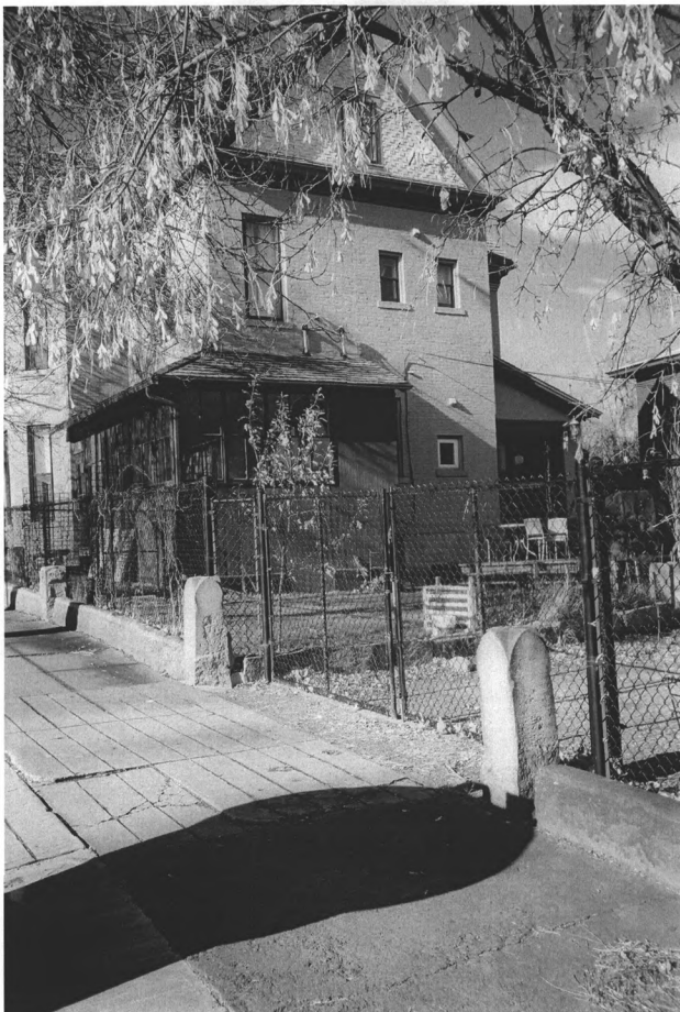
NR Photo #4: East (rear) elevation.
