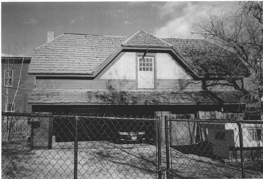
NR Photo #5: Carriage House, view to the north.
