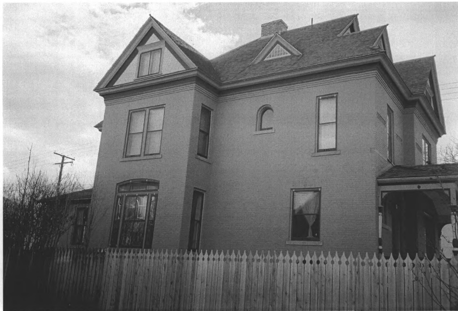
NR Photo #2: Side (north) elevation.
