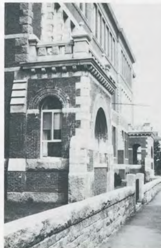
5. An entry is now a living area.
