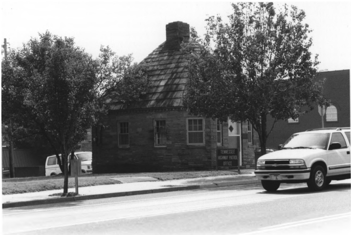
Crossville Tennessee Highway Patrol Building 9 of 22 Cumberland County TN
