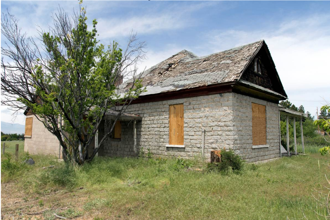
7 of 14. Southeast façade. Camera facing northwest.
