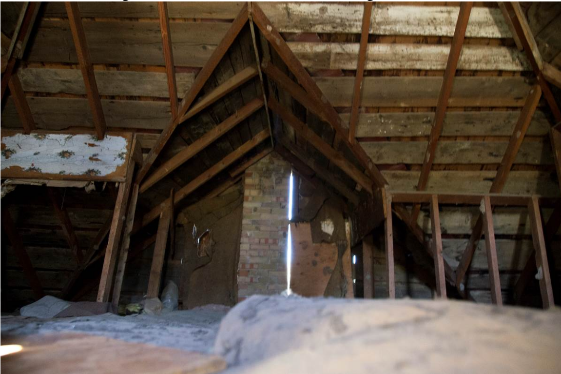
10 of 14. Roof and gable construction detail. Camera facing north.
