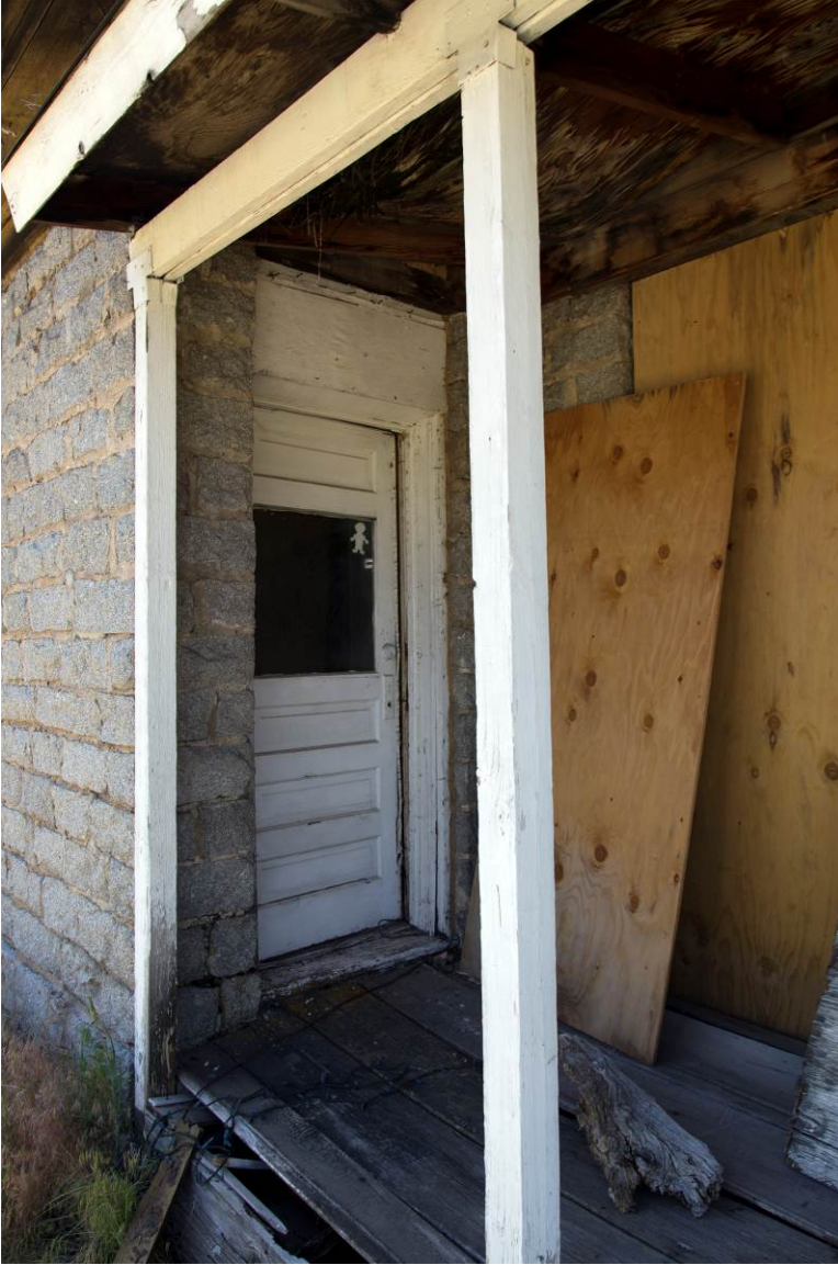
11 of 14. Porch and parlor entry five-panel door detail. Camera facing southwest.
