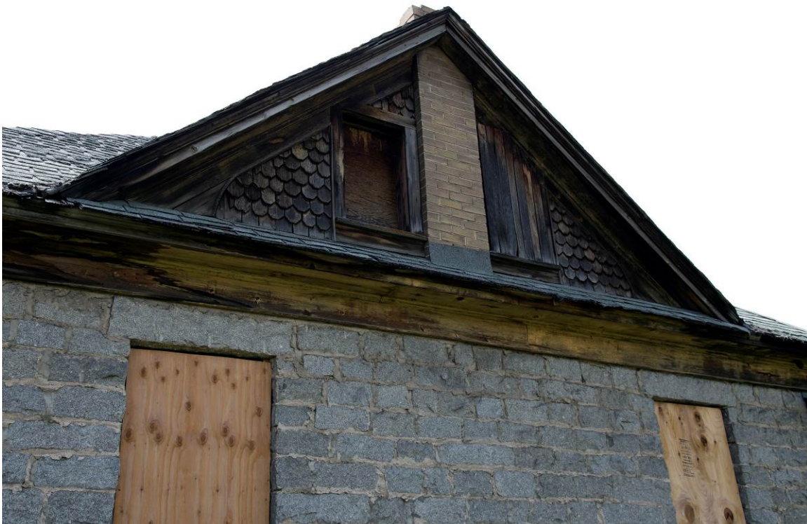
8 of 14. North façade gable detail. Camera facing south.
