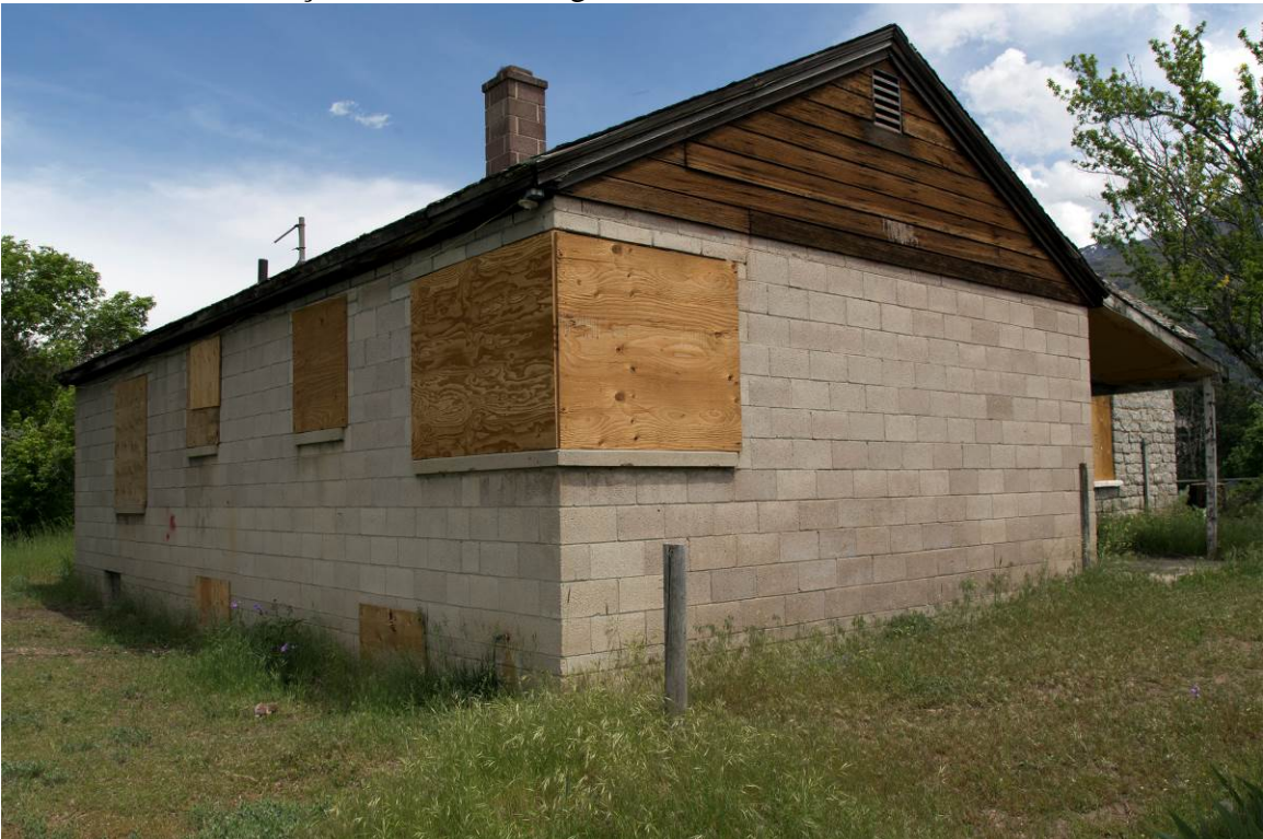
6 of 14. Southwest façade. Camera facing northeast.
