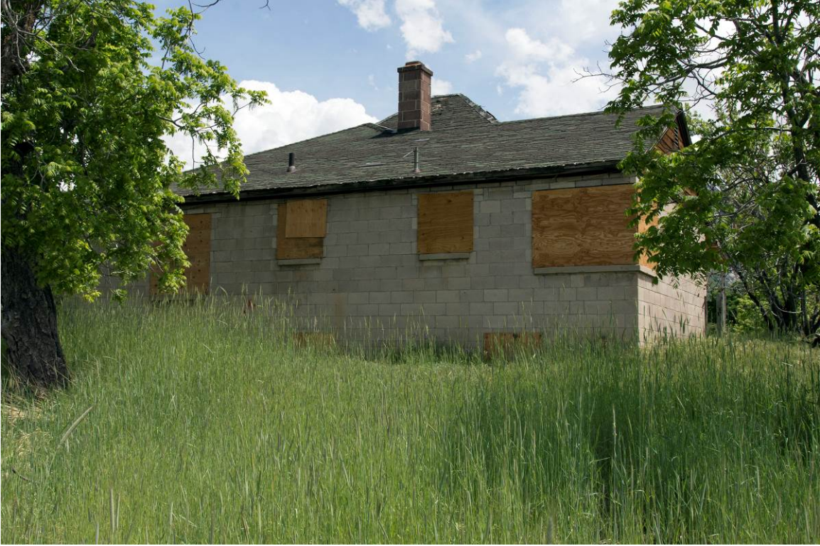
5 of 14. West façade. Camera facing east.
