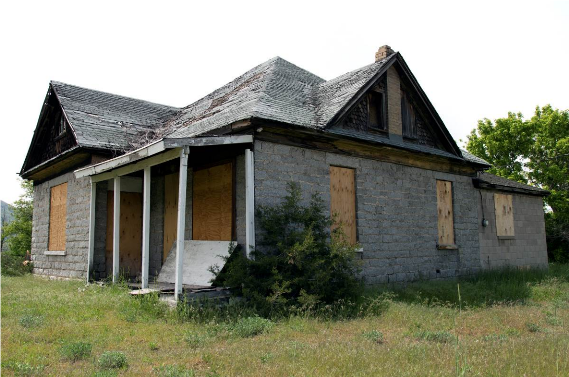
2 of 14. Northeast façade. Camera facing southwest.
