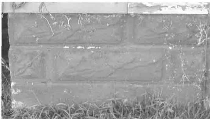
Detail of concrete block foundation
