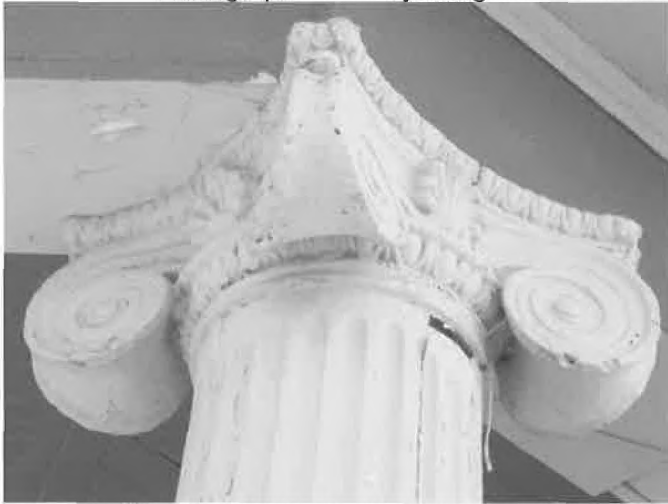
Detail of plaster capital on exterior porch column
