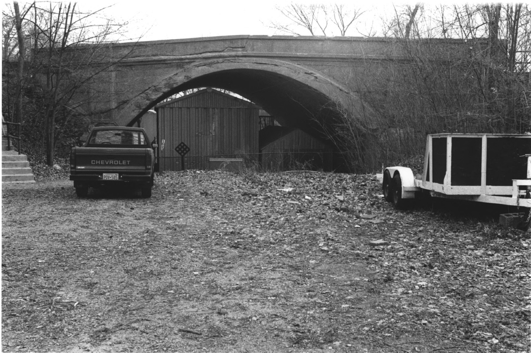
QUEEN AVENUE Bridge NO. C-9329 MINNEAPOLIS, HENNEPIN CO., MN Photo I.D. 09734 # 9
