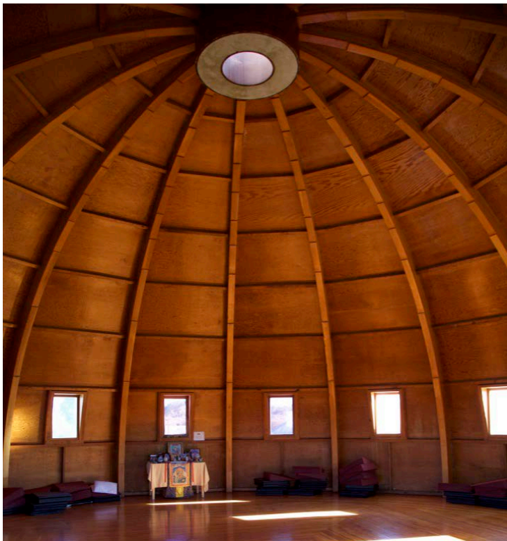
Figures 33 and 34. The glue-laminated Hughes HK-1/H-4 Hercules (Spruce Goose) fuselage construction compared to Integratron dome level interior. Curved, meridian rib predominance with secondary stringers; both are designed relative to compression. Photo (figure 33): Bettmann. Photo (figure 34): Daniel Paul.
