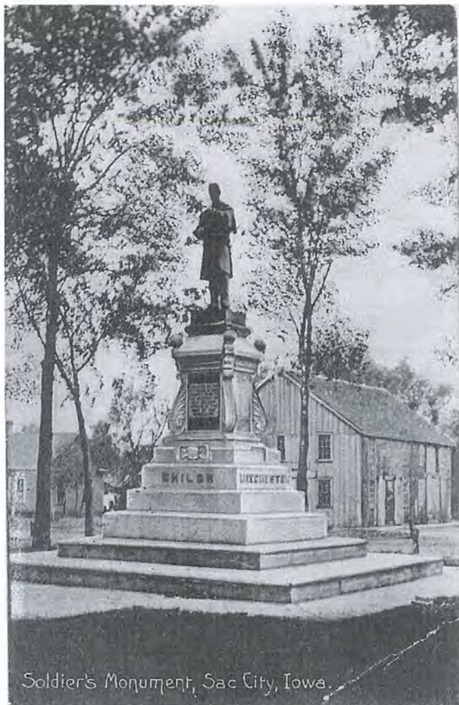
Image 40: 1911 view of Soldiers' Monument showing wooden buildings that originally surrounded Monument Square. The two-story wood building in the background shows the building torn down to make room for American Legion Hall. (Perry collection)
