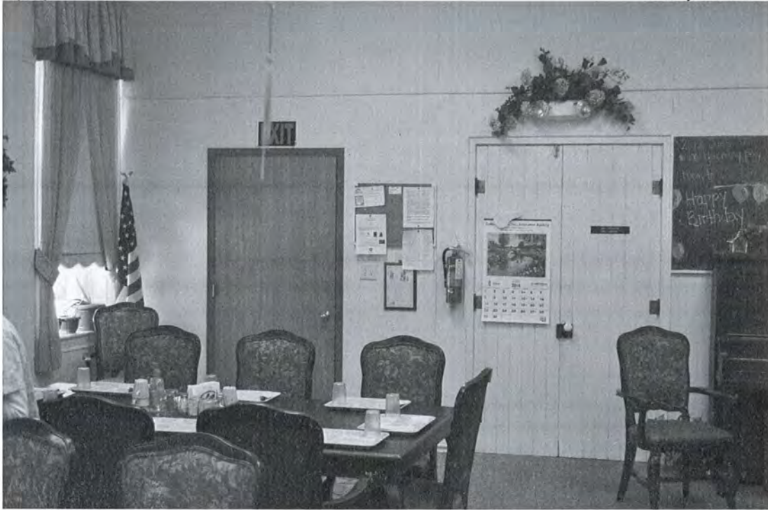
Image 8: A new door was added for entrance from the ante room to the meeting room in General Sherman Hall. The original double doors with peep hole are intact and now lead to a partitioned area of the ante room that contains freezers to preserve food for congregate meals. (photo Perry)
