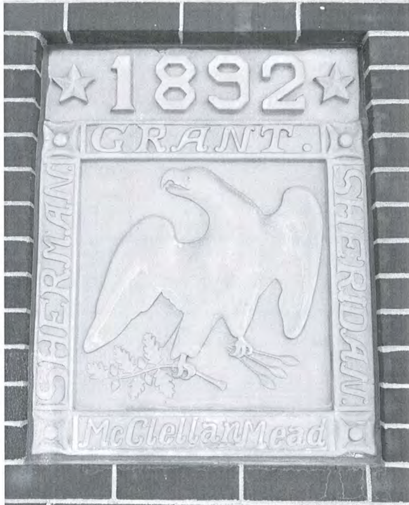
Image 5: East Bas relief inset on the north face of General Sherman Hall. The date 1892 would indicate that this piece served as the building's corner stone. The names of important Union Generals surround the rather curious bird bearing both symbols of stability and aggression in its talons. (photo Perry)
