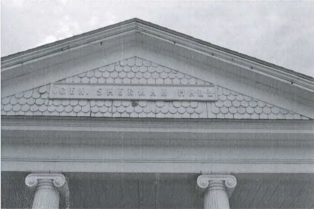
Image 2: Original sign, fish scale trim, and tops of Ionic pillars on north face of General Sherman Hall. (photo Perry)
