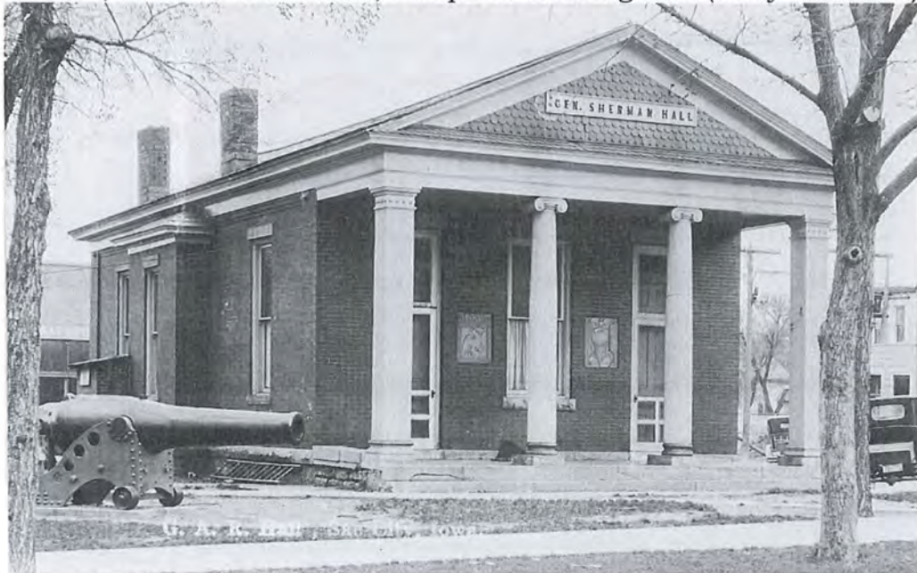
Image 19: 1924 photo of the front of General Sherman Hall showing original front doors, chimneys, and fish scale front above the portico. (Perry collection)
