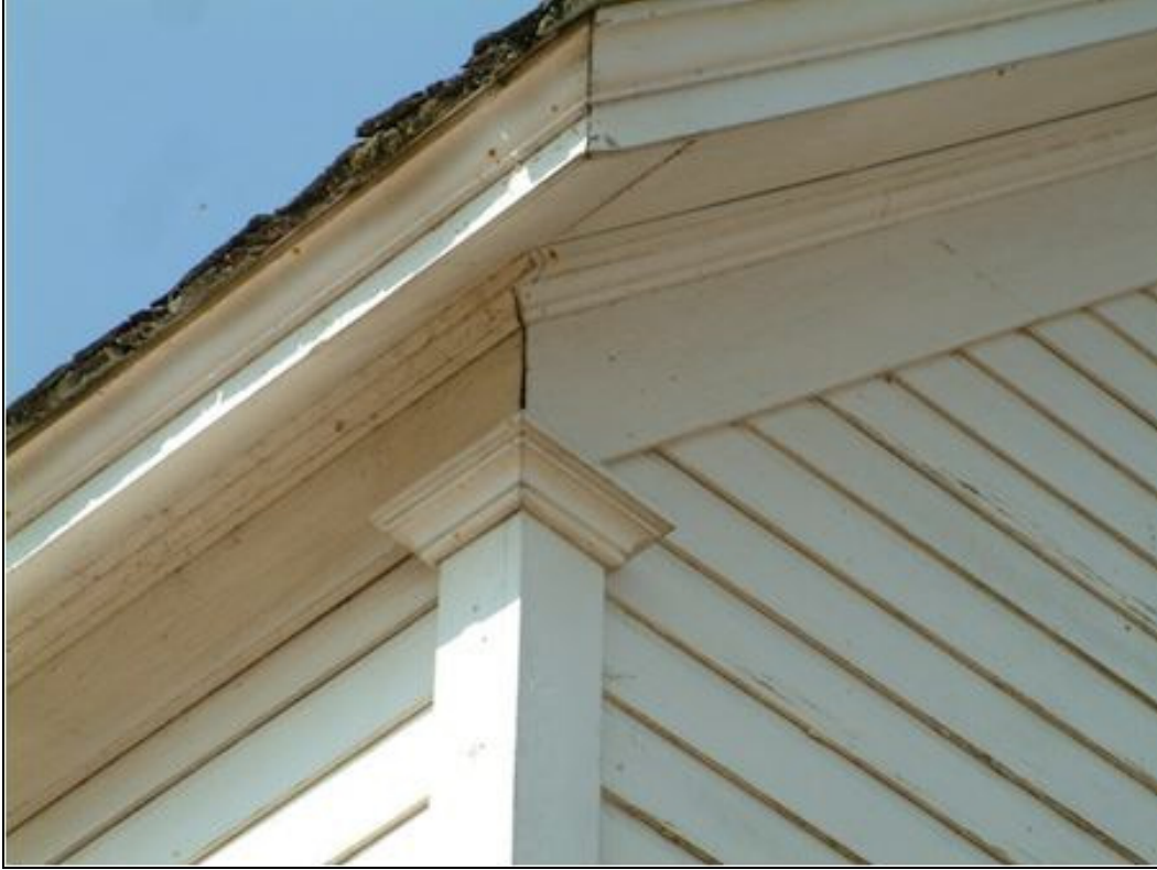
Photo 9 of 12: Detail of cornerboard and cap, frieze and eave.
