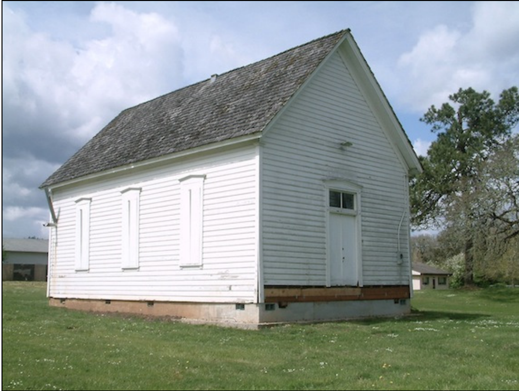
Photo 5 of 12: South and east elevations.
