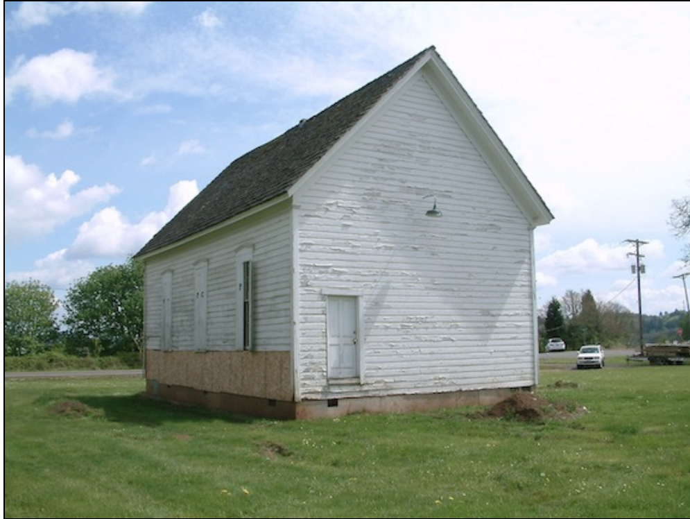
Photo 7 of 12: West (rear) elevation.
