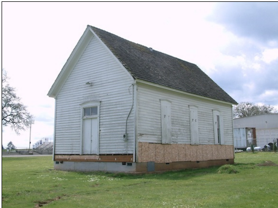
Photo 4 of 12: East (front) and north elevations.
