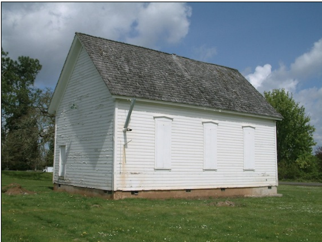
Photo 6 of 12: West (rear) and south elevations.
