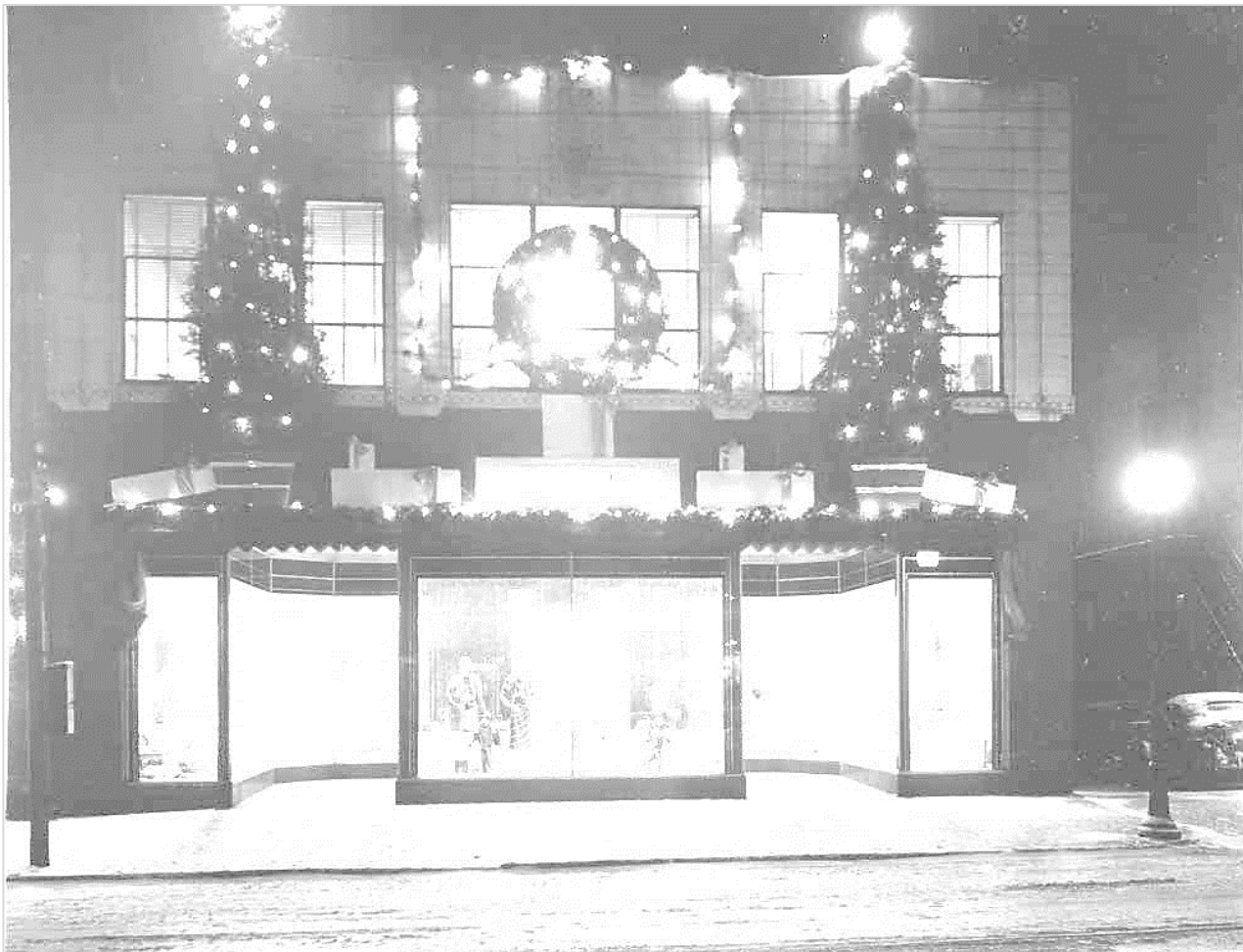
Figure 31. Noncontributing Spring-Holzwarth, 320 East Main Street (#16) showing terra cotta façade, Photo 5 December 1935.
