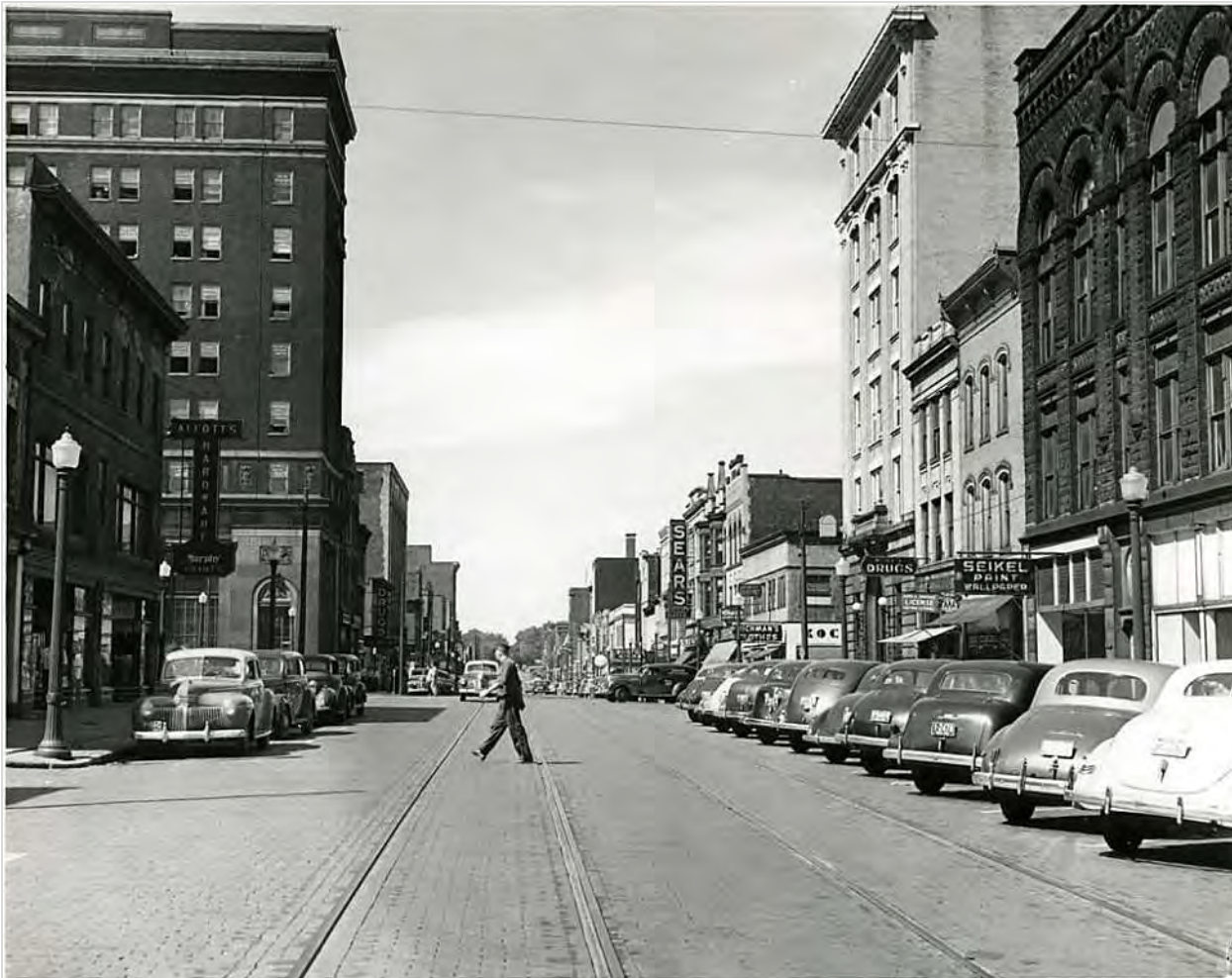
Figure 37. East Main Street, Photo 1941. View facing west from Seneca Ave.
