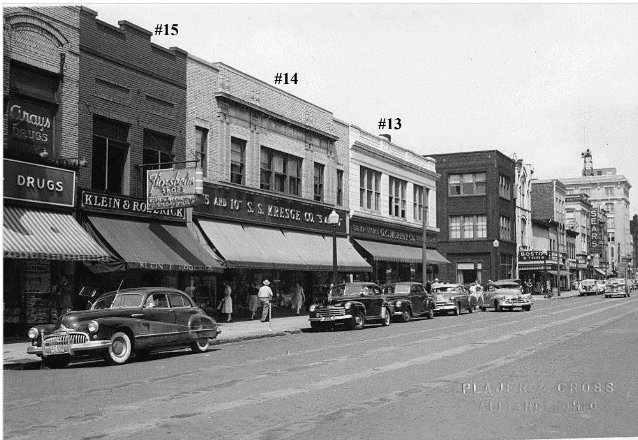
Figure 42. Klein & Roderick Building (#15), S.S. Kresge Building (#14), McCrorry Building (#13) 344-358 East Main Street, Photo 1950s. View looking east from Arch Street.
