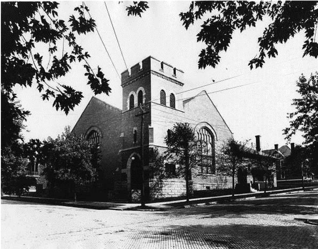
Figure 43. First Presbyterian Church Complex, 425 East Market St. (#72), Photo Undated.
