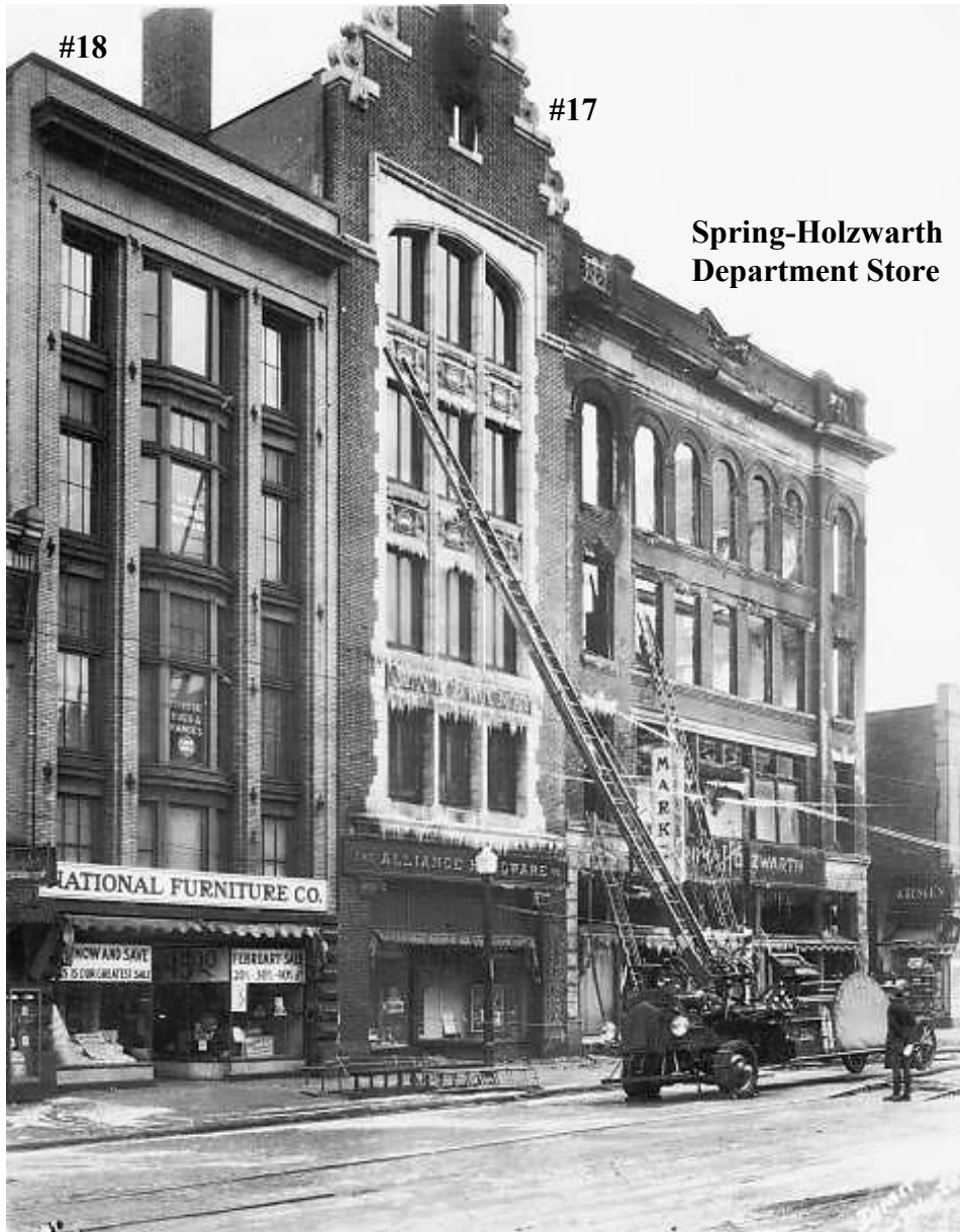
Figure 29. February 1, 1931 Fire. Destroyed Spring-Holzwarth Department Store at 320 East Main St. and fractable of Alliance Hardware, 318 East Main St. (#17). Cassaday Furniture Co. Building, 314 East Main St. (#18) also pictured.
