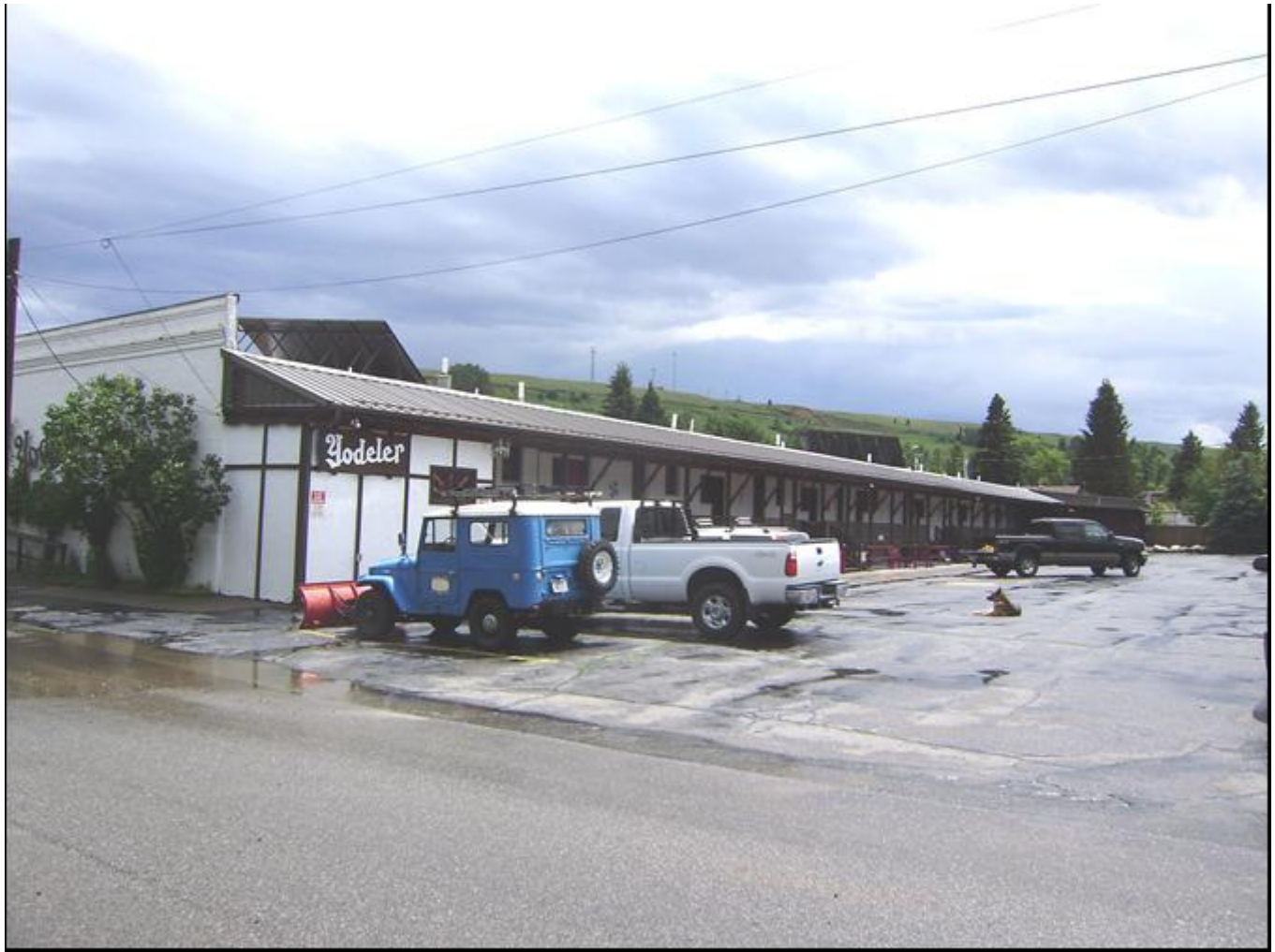
Photo 0013. West Facade. View to the southeast.
