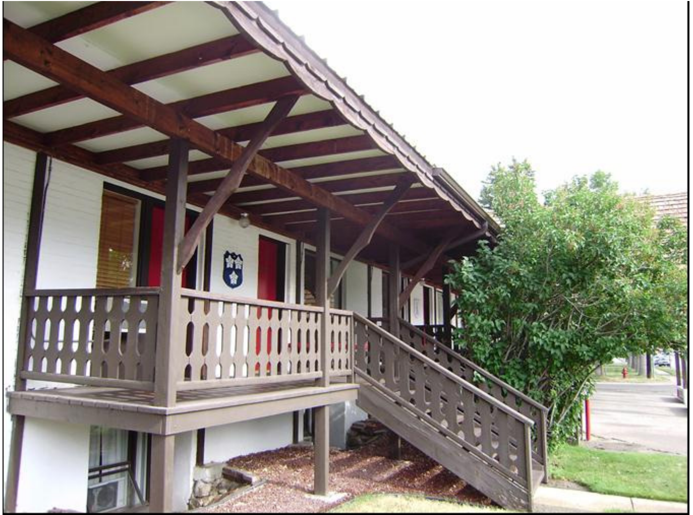
Photo 0004. Facade. View to the north-northwest.
