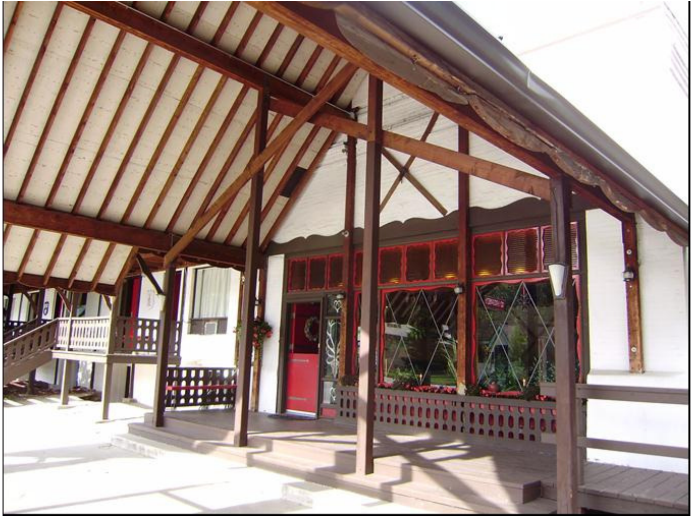
Photo 0009. Office/Reception Area. View to the southwest.
