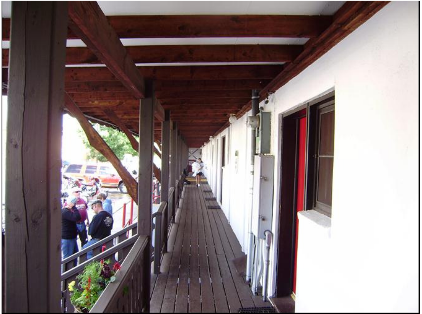
Photo 0014. West Façade Walkway. View to the north.
