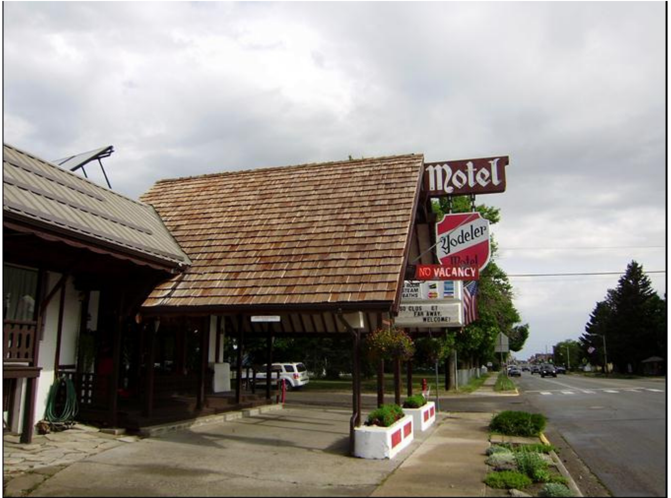
Photo 0007. Office/Reception Area. View to the north.
