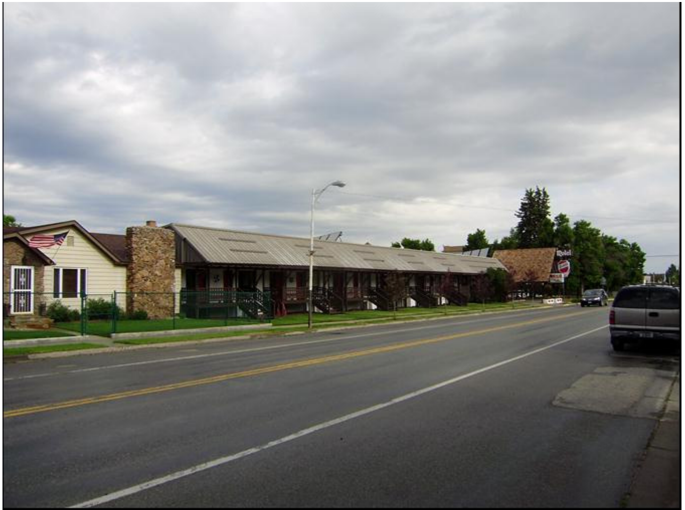
Photo 0002. Façade Overview. View to the north-northwest.
