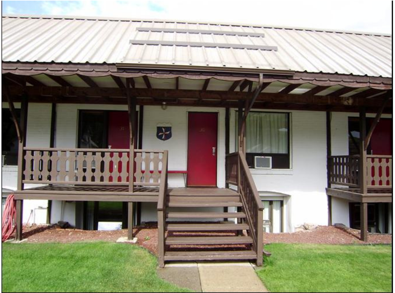
Photo 0005. Detail of room entries. View to the west.
