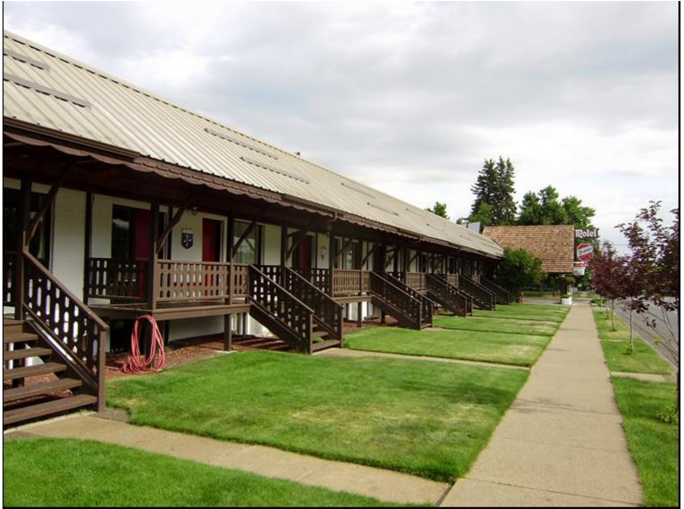
Photo 0003. Facade. View to the north-northwest.
