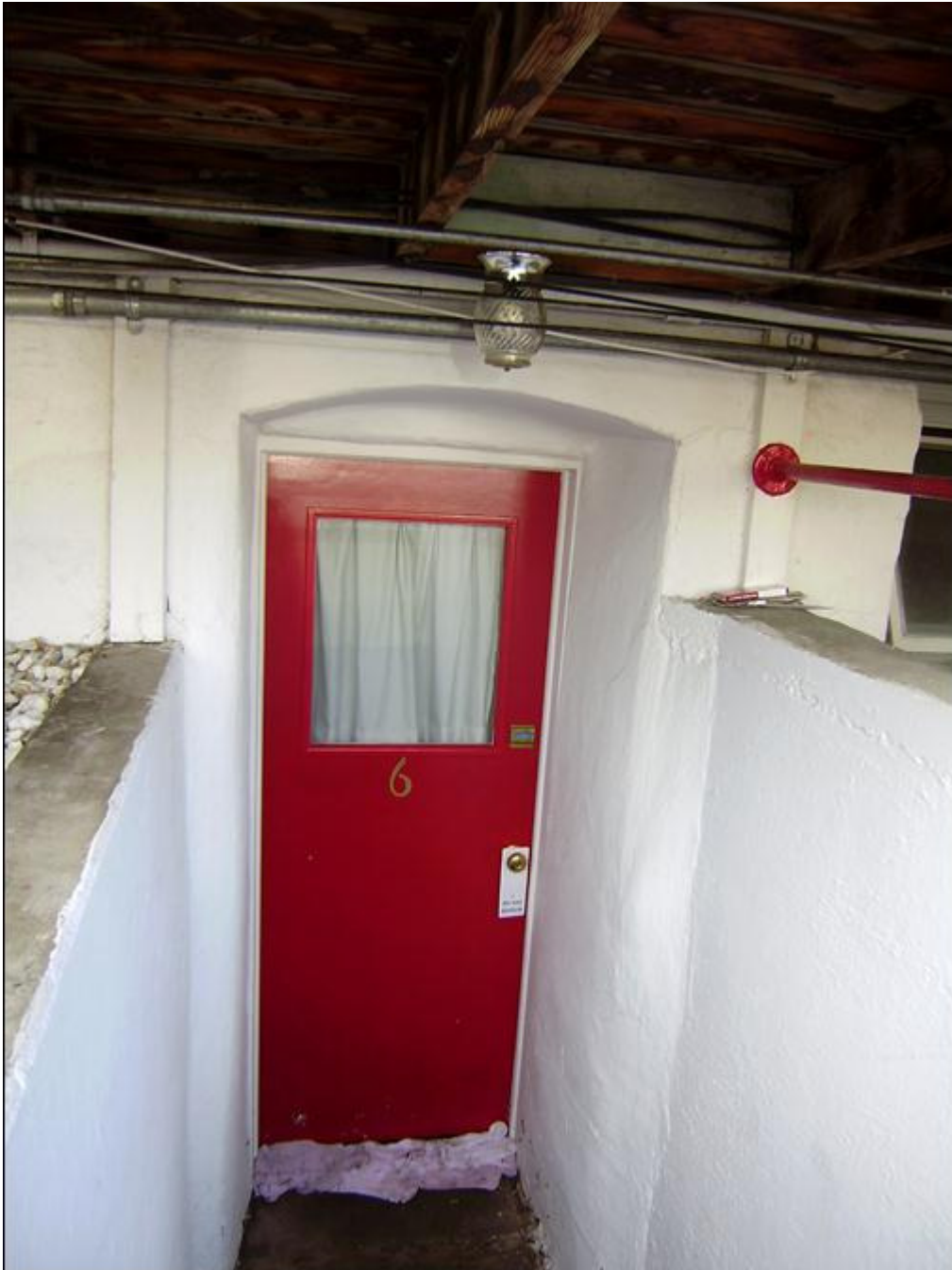
Photo 0016. Detail of West Façade Entry. View to the east.
