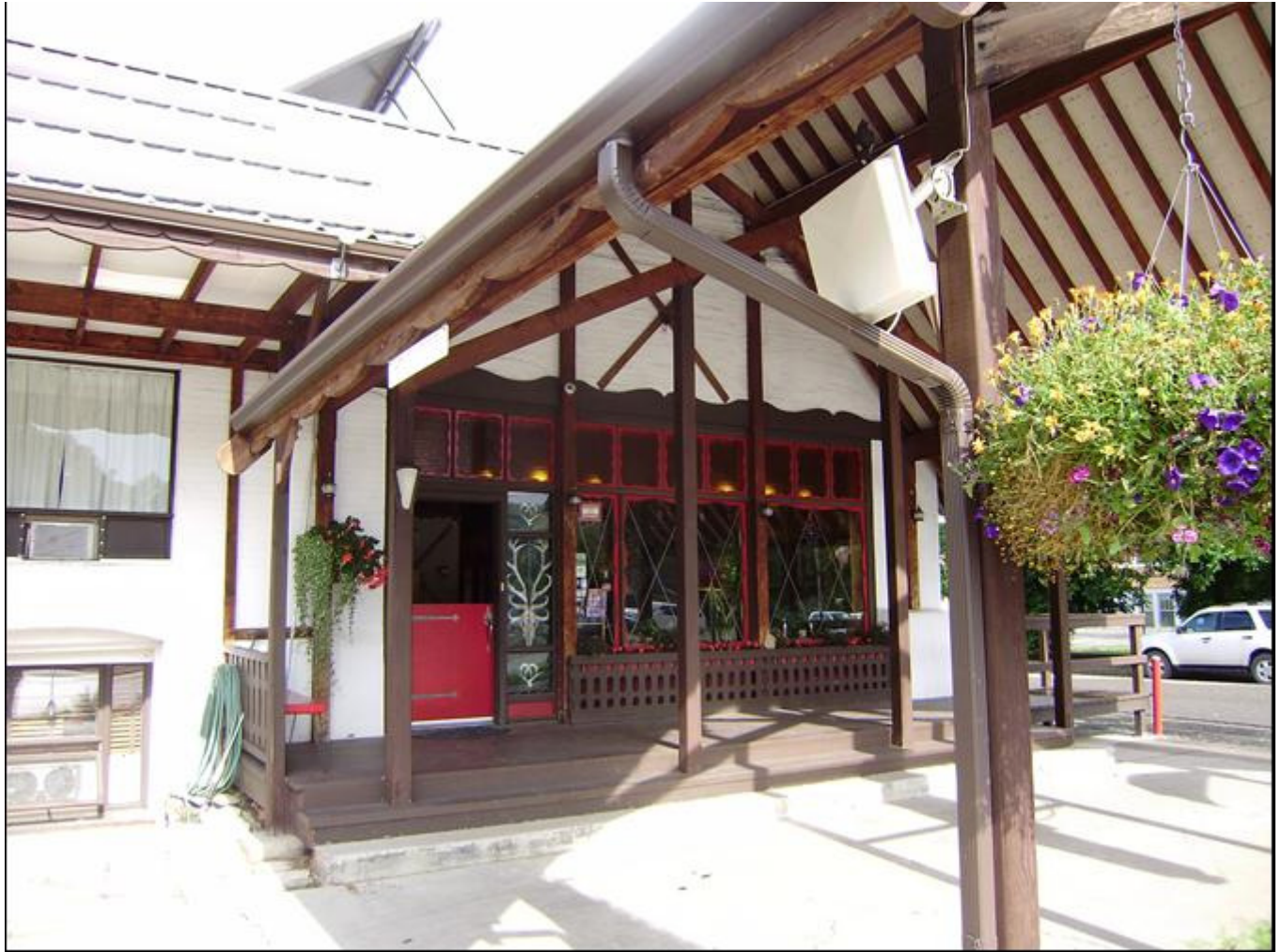
Photo 0008. Office/Reception Area. View to the northwest.
