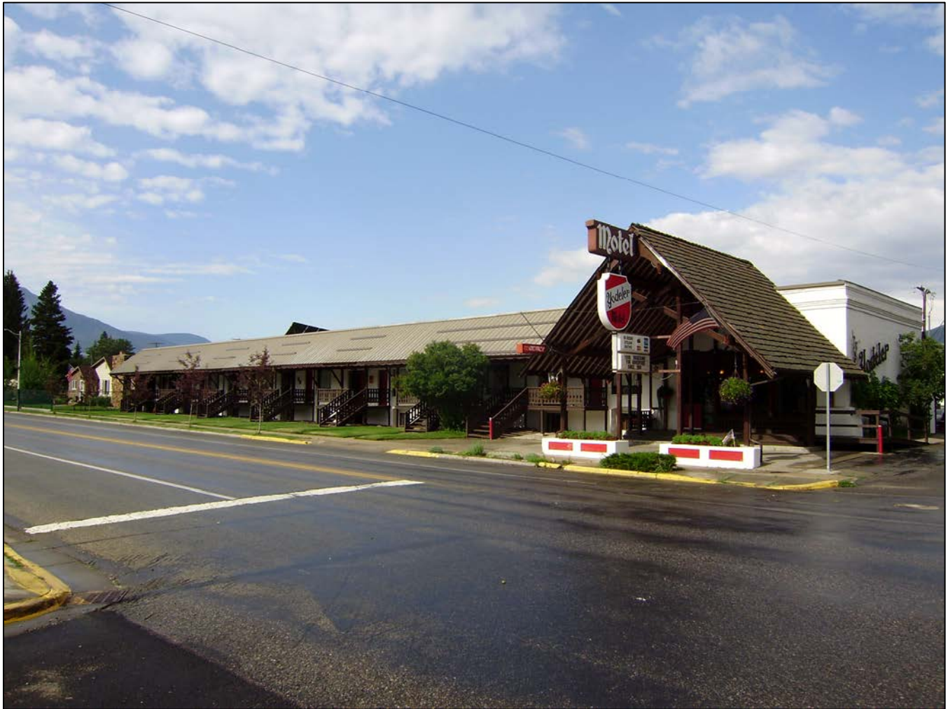
Photo 0001. Façade overview. View to the southwest.
