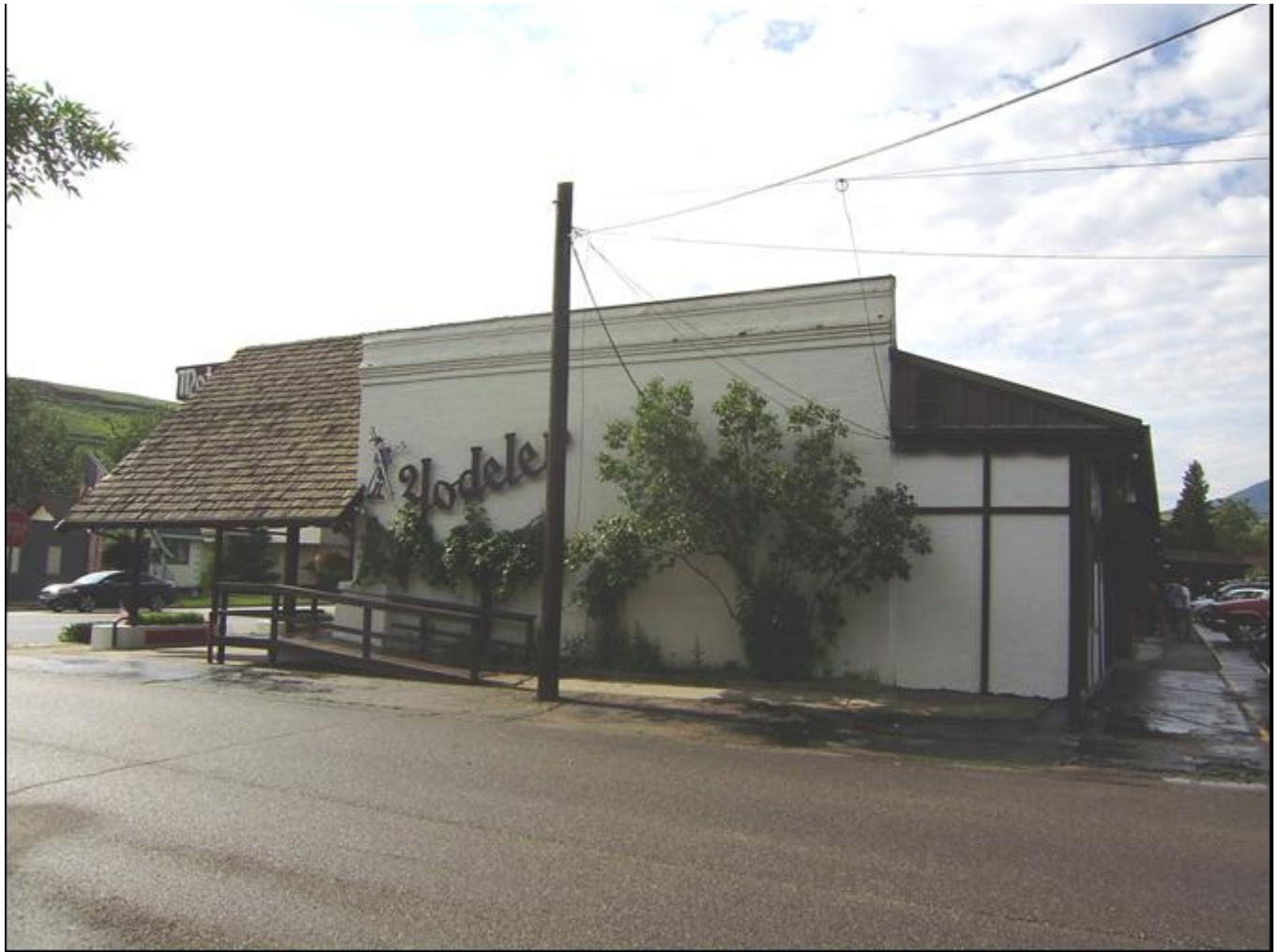
Photo 0011. North Elevation. View to the south.
