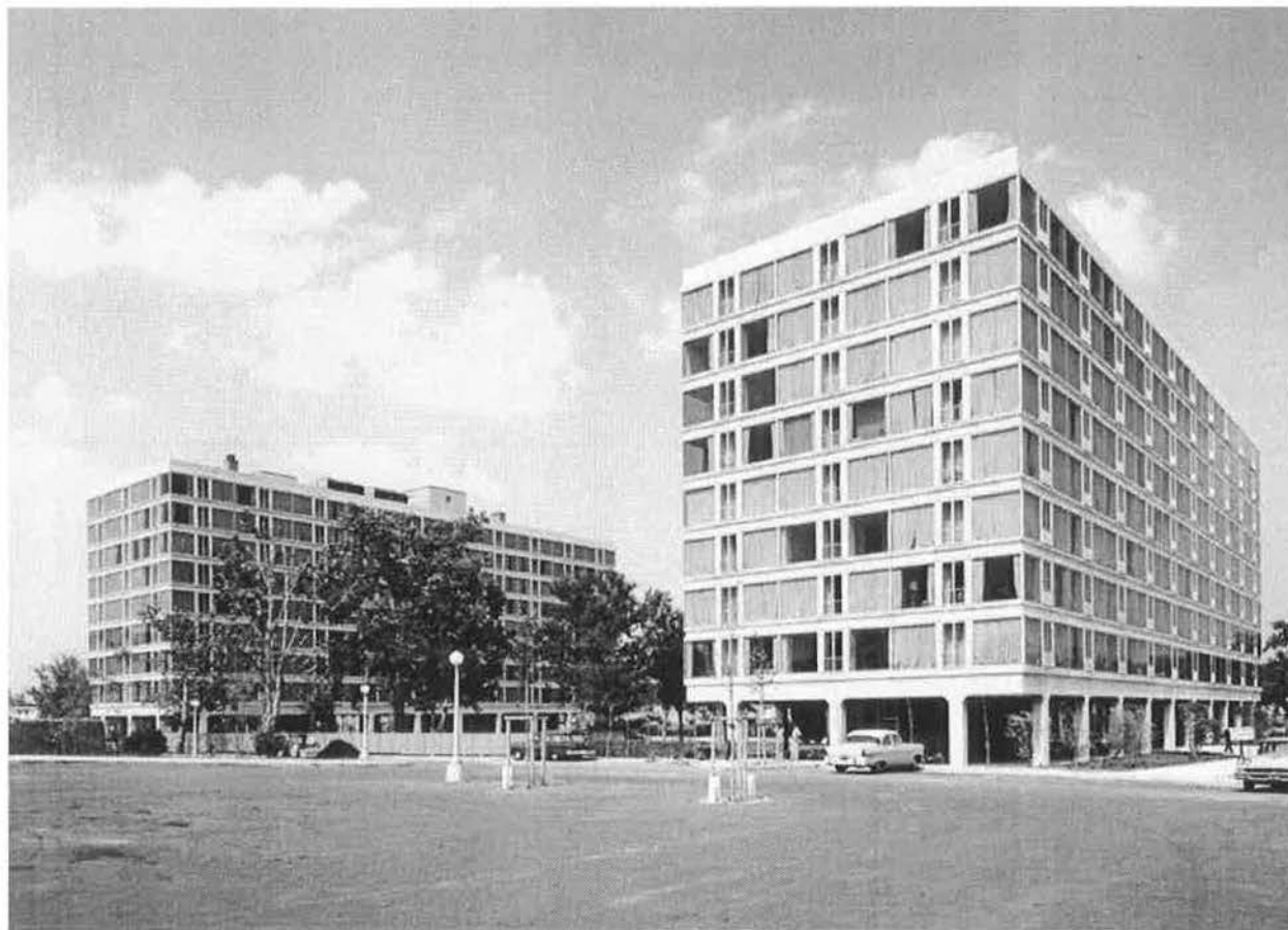
Post-construction photo of Town Center Plaza Apartment Towers showing courtyard privacy wall with egress, Photographer: George Cserna (Courtesy Pei Cobb Freed & Partners)
