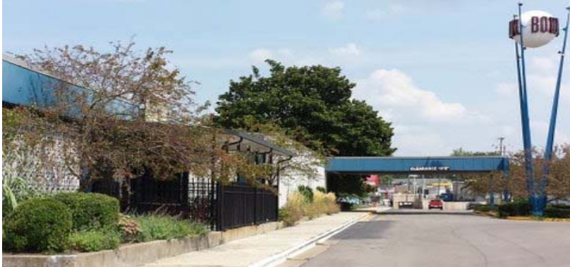
Southland Bowling Lanes, 205 Southland Drive, Lexington, KY, Built 1963
