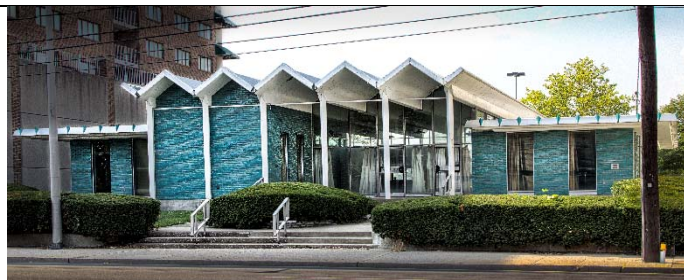
Exterior View of Folded Plates
