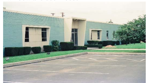
Pepsi Cola Bottling Plant, Built 1968 559 S Forbes Road, Lexington, KY Blue ceramic glazed brick with concrete window and door hoods
