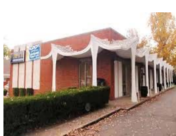
Doctors Office Building, Built 1965 1529 Nicholasville Rd, Lexington
